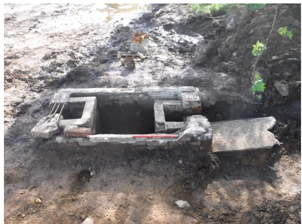
Plate 88 Settling tank [292], general view. Facing E
