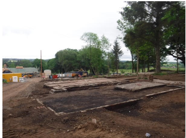
Plate 11 Type 1 specialised Buildings 15 (foreground) and 14 (background), general view. Facing SW
