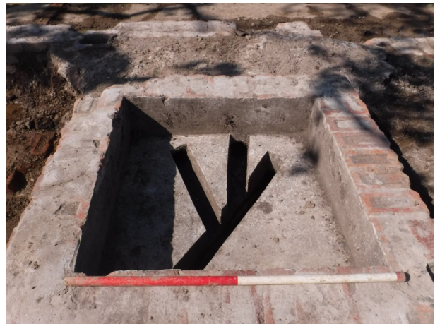
Plate 80 Junction box [325] detail. Facing N
