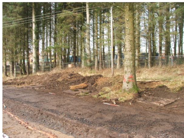
Plate 6 Camp Road [045], north-eastern extent, with drainage features [040], [041], [042] on north side. Facing north-west
