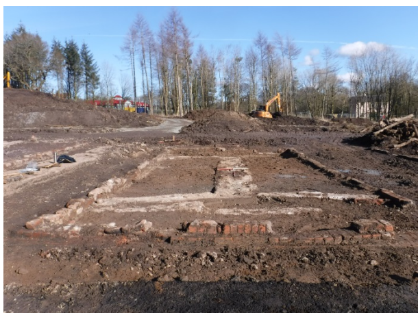
Plate 34 Building 35, general view with internal sanitary block features. Facing E
