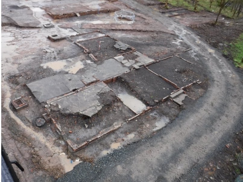
Plate 53 Building 87, general view. Facing NE
