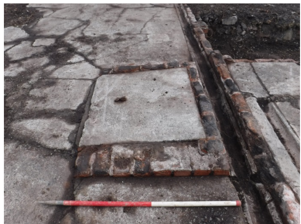
Plate 57 Building 87, Room E, detail of concrete plinth [255]. Facing E
