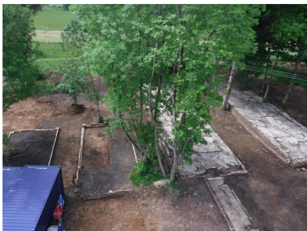
Plate 16 Type 1 Building 39 (left), Type 2 Building 70 (right). Facing W
