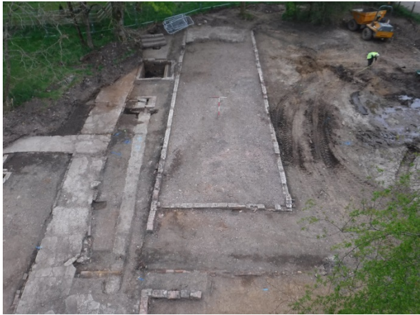
Plate 26 Building 58 general view. Facing E
