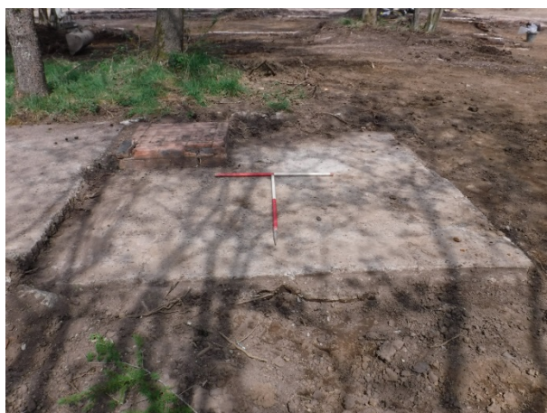
Plate 43 Building 59, general view, NE end with lower floor and plinth [291]. Facing SW
