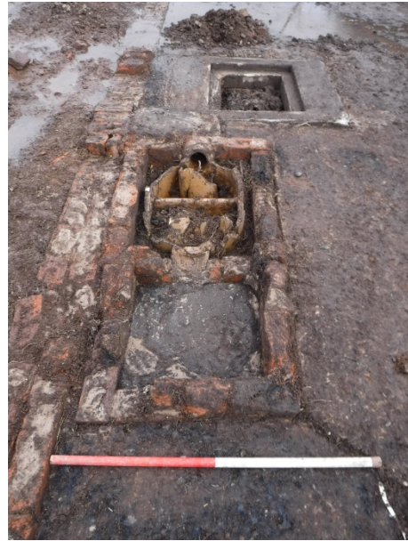
Plate 90 Settling tank [074] with [075] in background. Facing E
