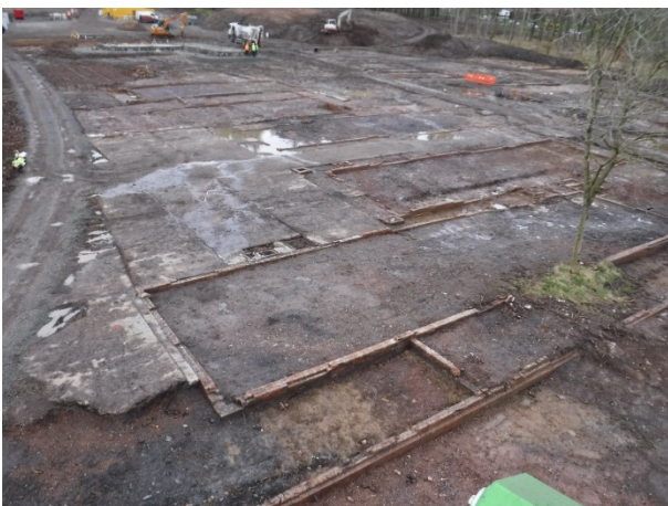
Plate 51 Building 86, general view of north-east flank of building with open area [031]. Facing NE
