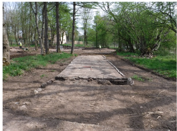
Plate 41 Building 59, general view, SW end with sandstone rubble walls [300]. Facing NE
