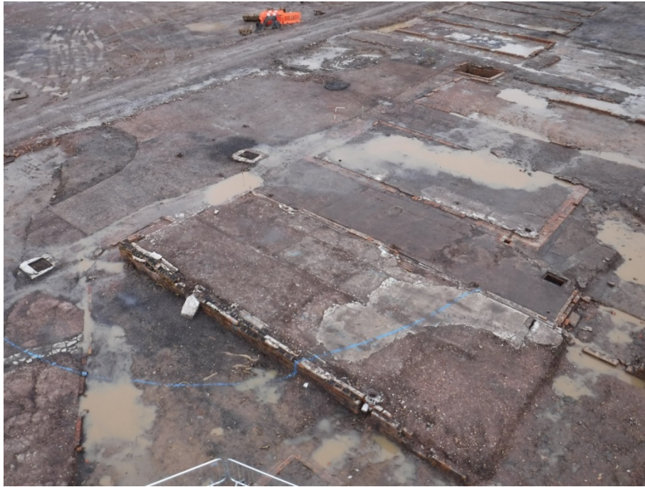
Plate 58 Buildings 29 (foreground), 52 and 46 with open area [246]. Facing NW
