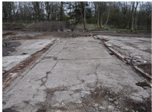
Plate 62 General view concrete surface [233] between Buildings 29 and 52. Facing E
