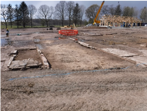
Plate 65 Building 46, general view. Facing W
