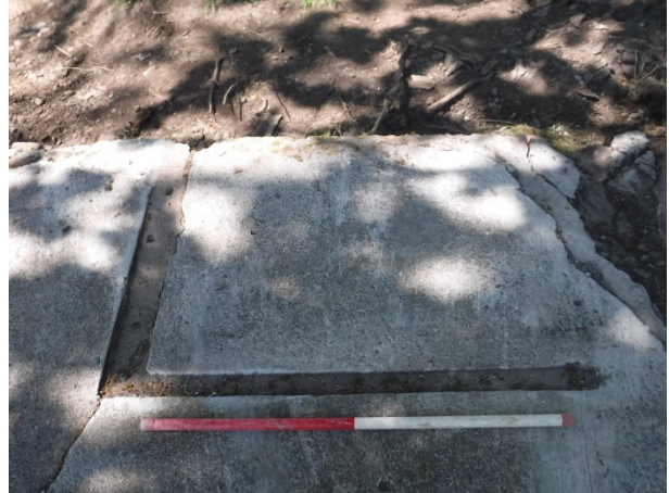
Plate 19 L-groove in concrete floor, windbreak partition? Building 72 floor [407], W end. Facing W
