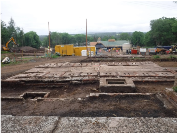
Plate 12 Specialised Type 1 Building 14 (latrine), general view. Facing S
