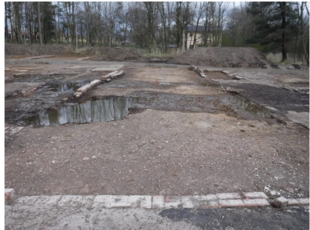
Plate 66 Building 46, general view. Facing E
