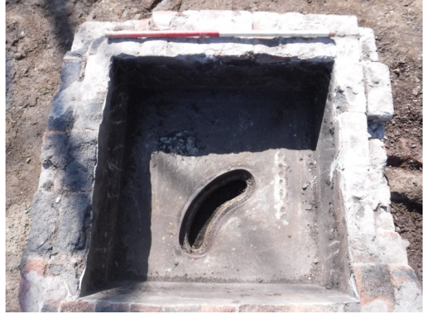
Plate 78 Junction box [323] detail. Facing W
