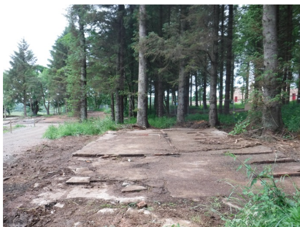
Plate 35 Building 81, general view with internal sanitary block features. Facing W
