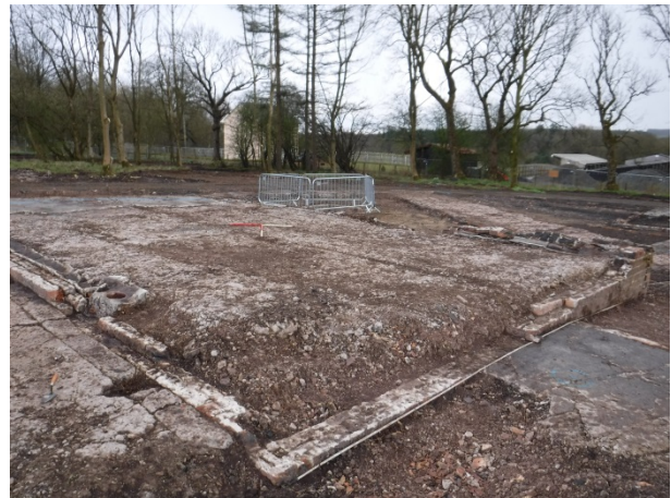
Plate 60 Buildings 29 general view. Facing SE
