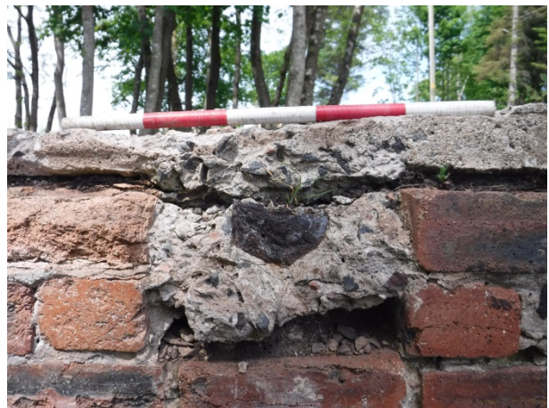
Plate 23 Type 2 Building wall socket. Building 73. Facing S
