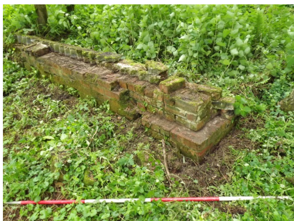
Plate 37 Type 3 Building 84, general view showing superstructure. Facing S
