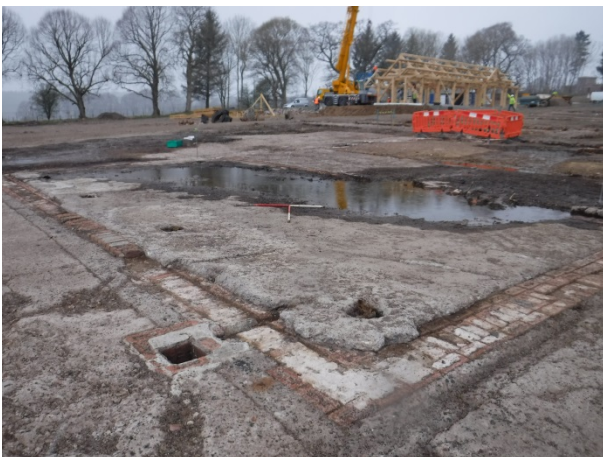
Plate 61 Building 52 general view, with part of posthole alignment [236]. Facing NW
