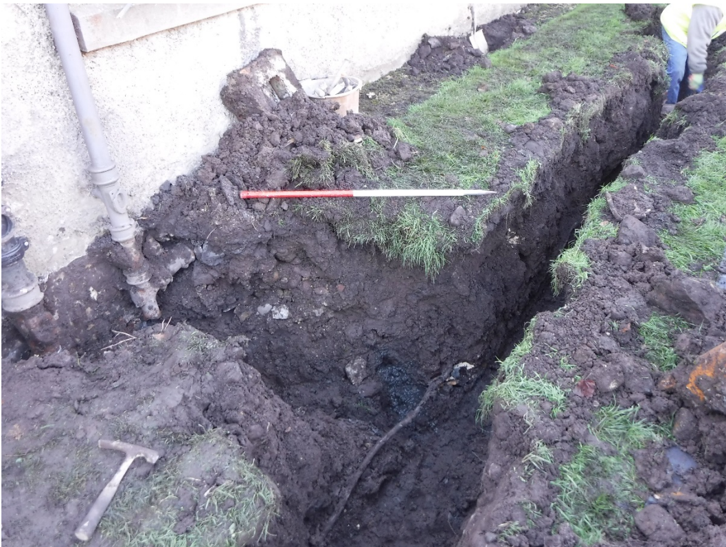
Plate 2 Working section of a branching pipeline in the excavated trench
