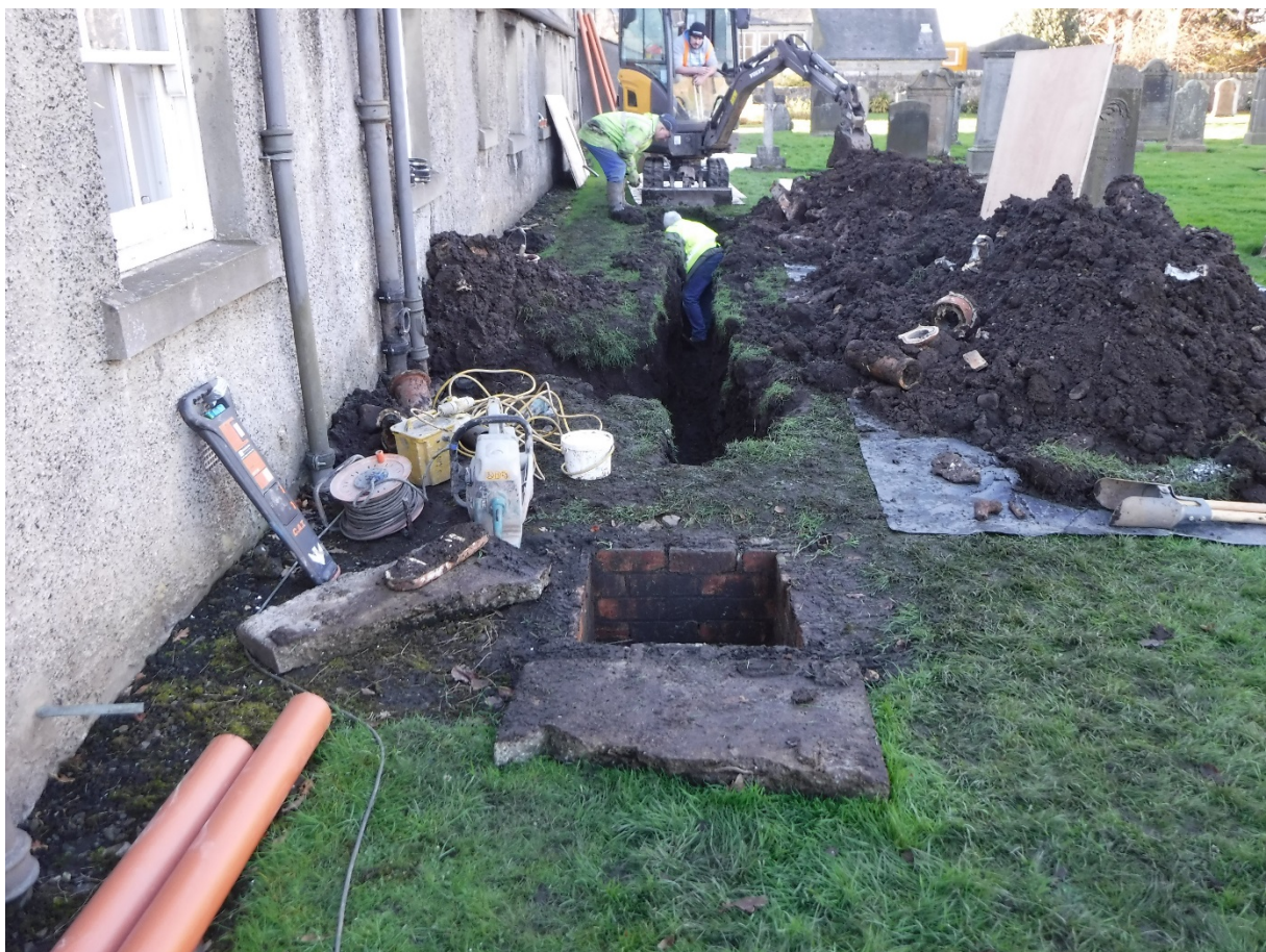
West-facing view of the excavations in progress
