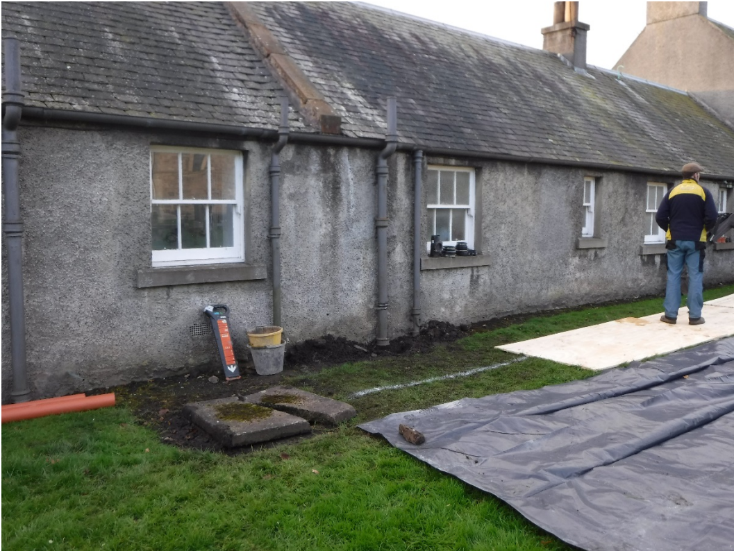
Plate 1 East end of the trench prior to the commencement of works
