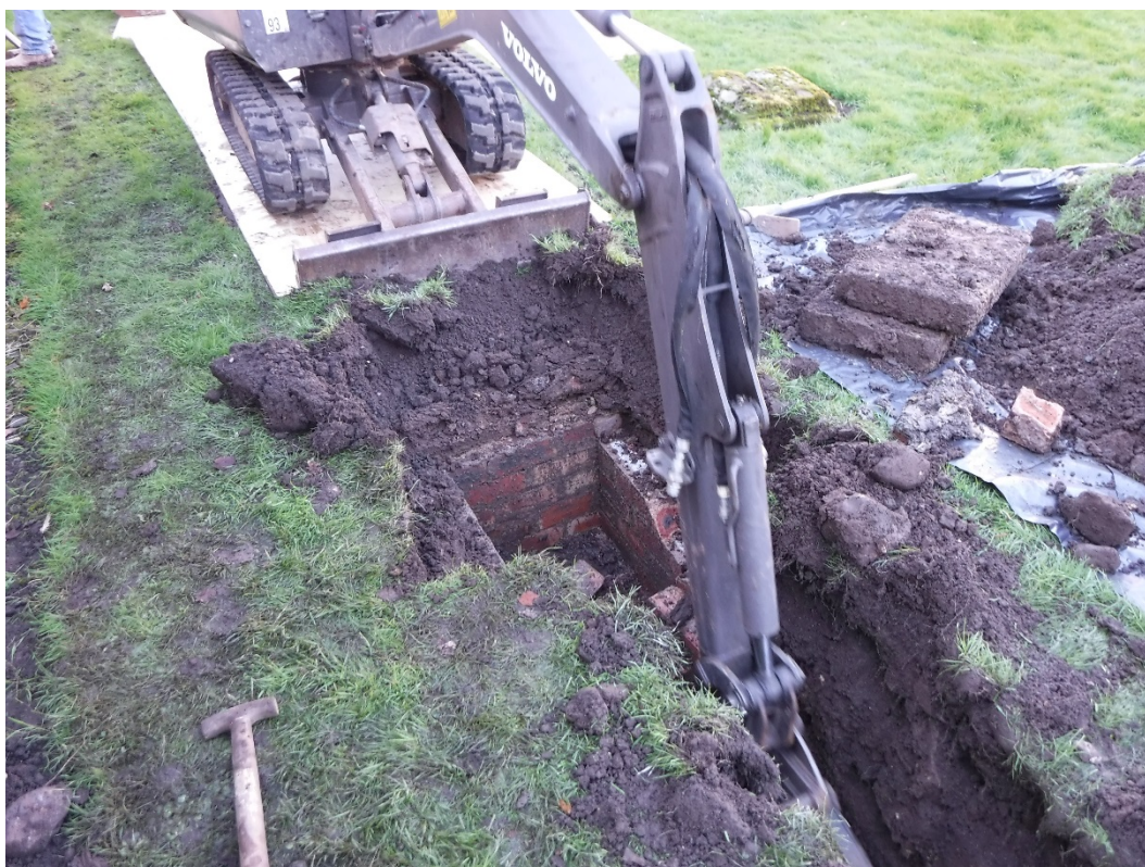
Plate 3 Demolition of the inspection chamber in progress
