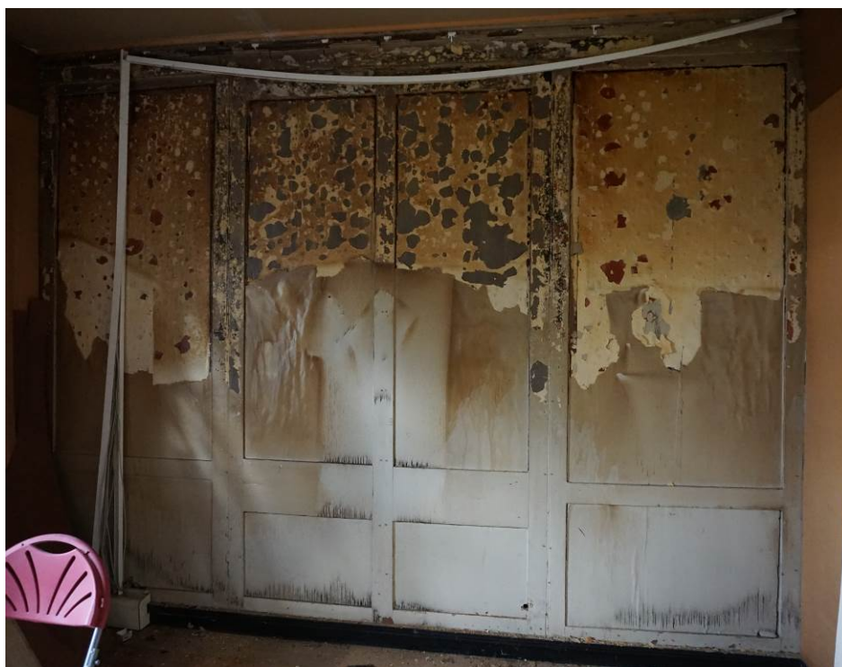
Plate 20 room F.03 early panelling exposed
