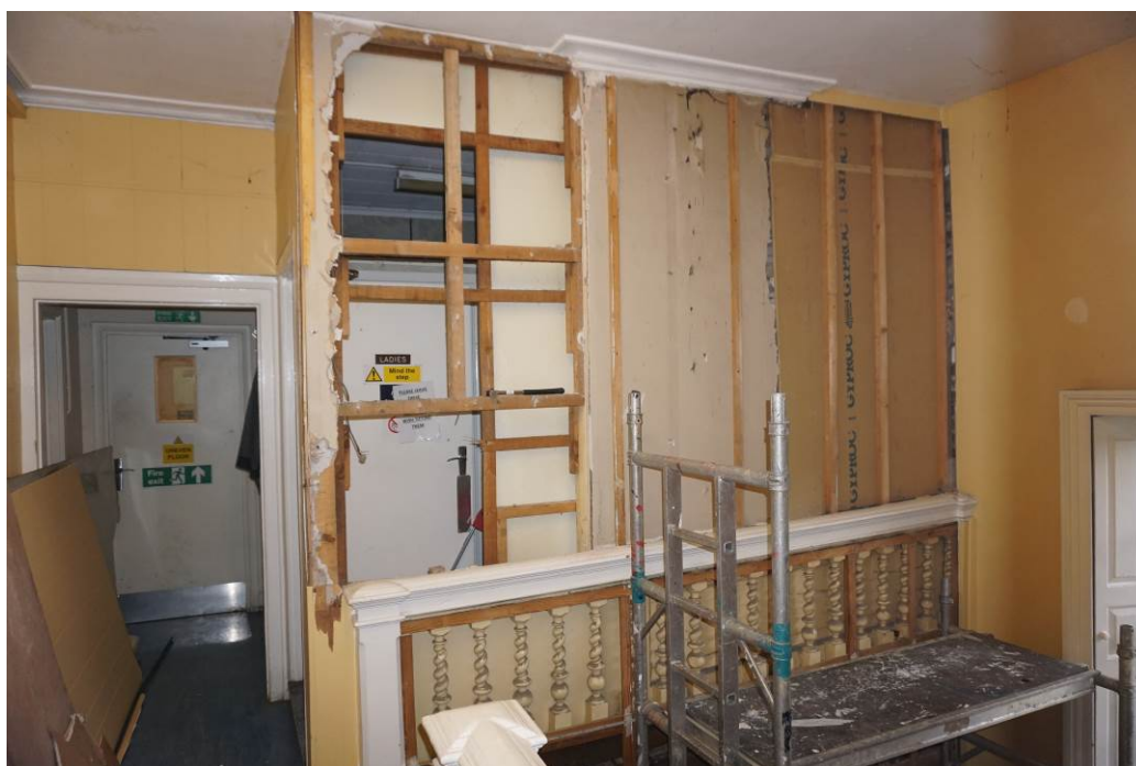
Plate 14 1st floor partition between stair F.01 and toilets F.04 showing surviving strip of original fabric down the middle with mid-20 th C stud partition extension to left and later 20 th C repairs to the right pre removal. Note truncated cornice
