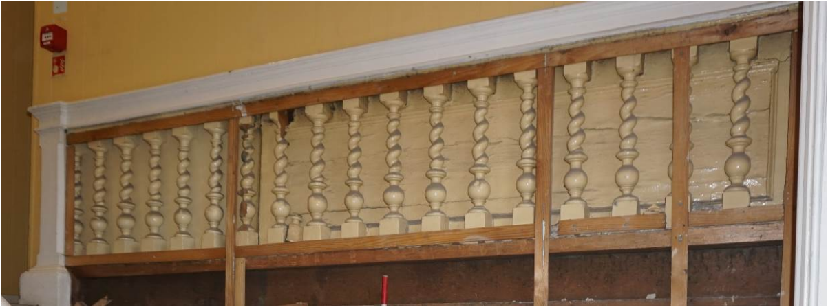
Plate 15 papered over boarded panelling behind baluster
