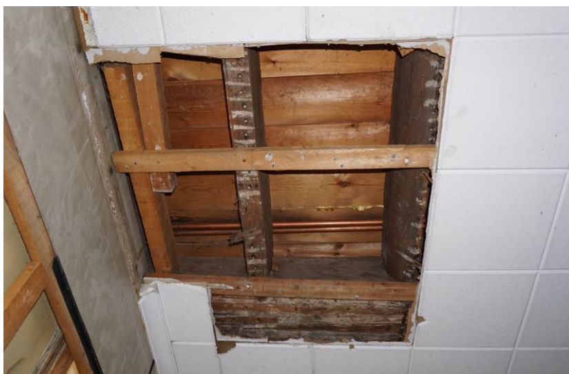
Plate 17 room F.04 ceiling investigation shows floor structure
