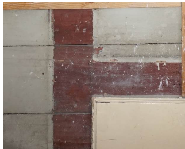
Plate 10 panelling detail showing original reddish finish and dirt shadow on paint around lost applied mouldings
