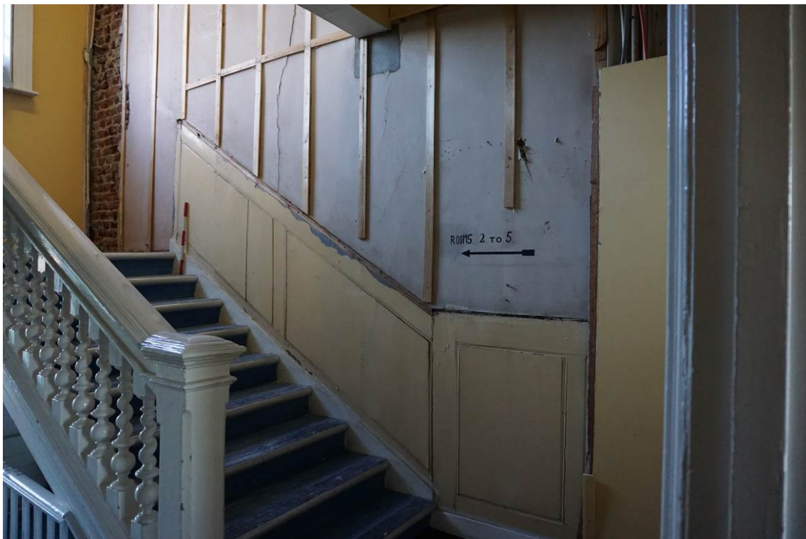
Plate 5 room F.01 stairwell shows exposed panelling on south elevation
