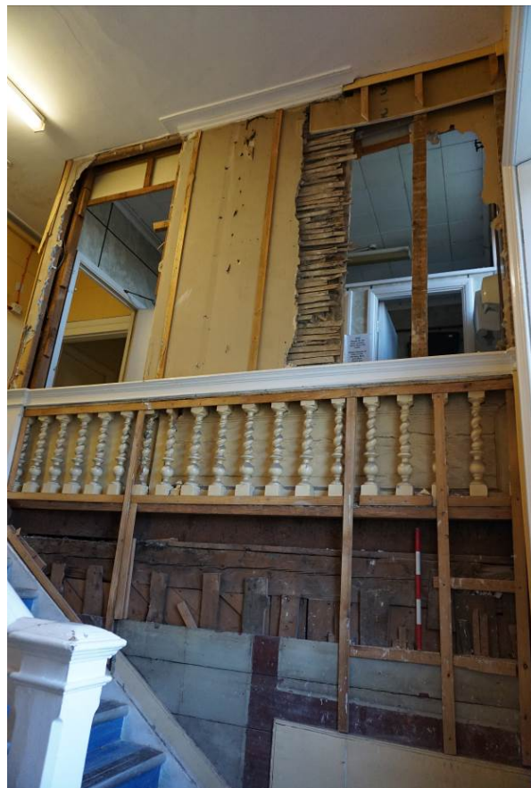
Plate 8 room F.01 stripped elevation showing exposed early structure on north elevation
