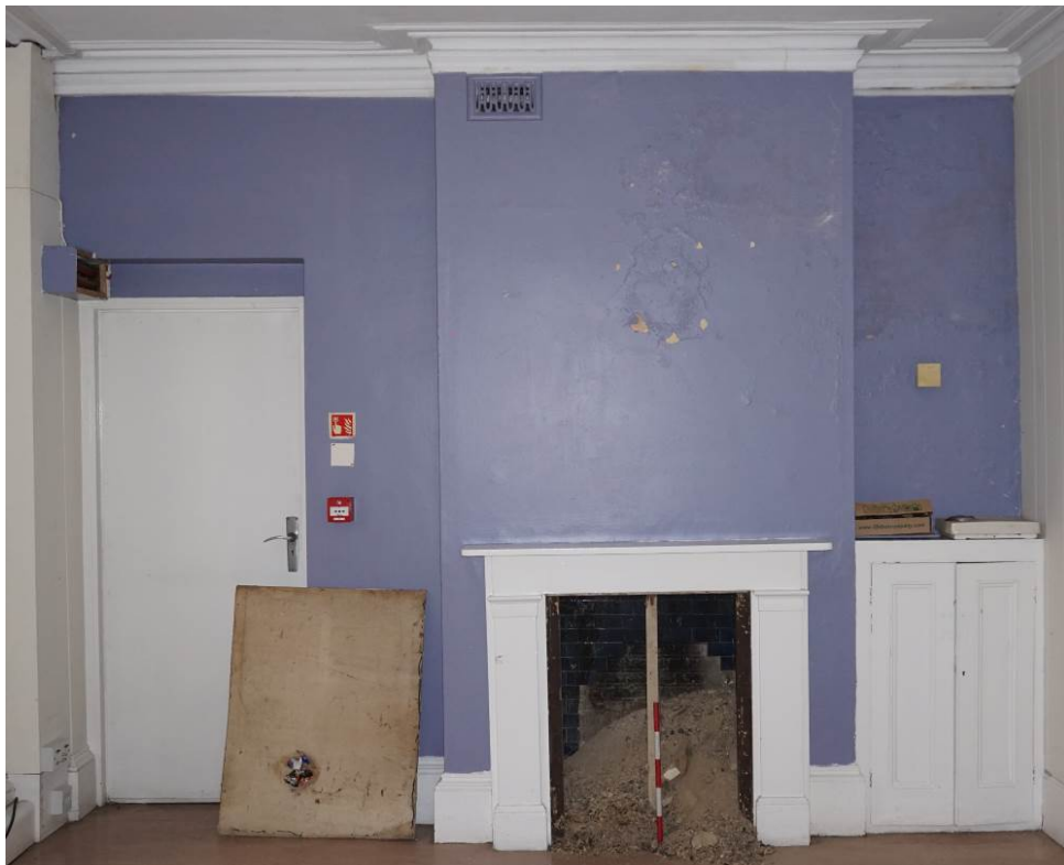
Plate 3 room G.06 fireplace uncovered
