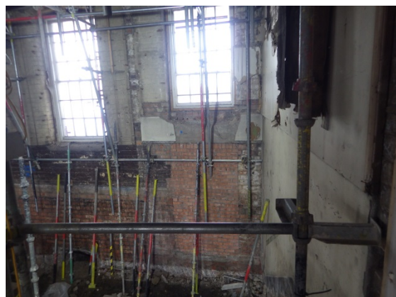
Plate 34 Brick-blocked internal face of door 116.
