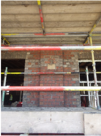
Plate 17 Detail of bi-chrome decoration on Phase 1 ground floor brick, south-west elevation .
