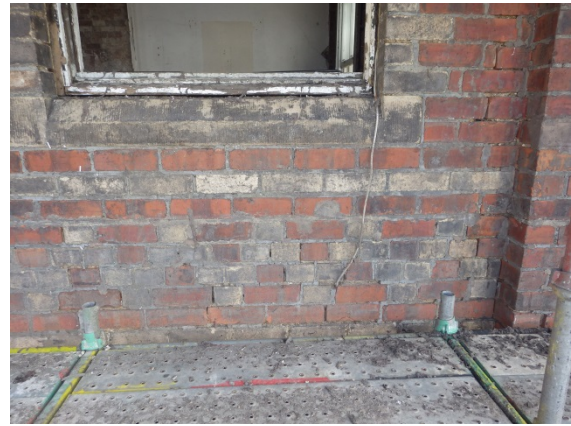
Plate 18 Detail of bi-chrome decoration on Phase 1 first floor brick, south-west elevation.
