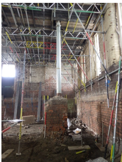
Plate 49 Steel column with foundations.
