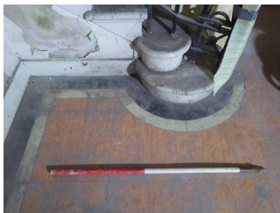
Plate 28 Lower ground floor, detail of stair hall marble-effect rubber floor tiles.
