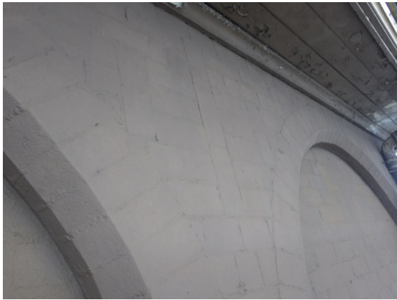
Plate 11 Detail of cruciform brick decoration between bay arch heads.
