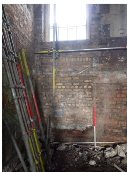
Plate 36 Brick-blocked internal face of door 143.
