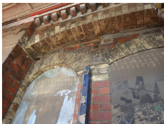
Plate 26 Doors 062 and 063 with arched bay and denticulated cornice.
