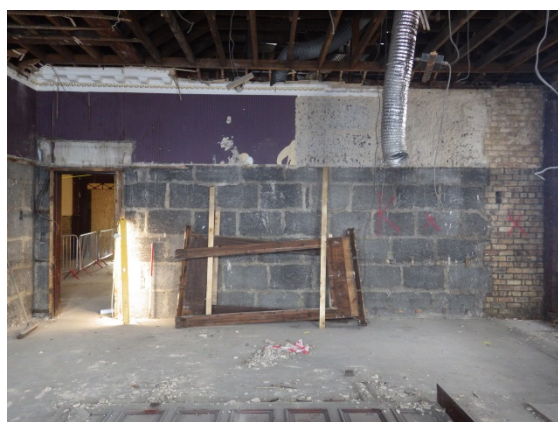
Plate 60 First floor interior, east room with Phase 2 brick, Phase 3/4 breezeblock and egg-and-dart denticulated crown moulding. Facing NW.
