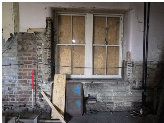
Plate 47 Window 094/095 with inserted brickwork
