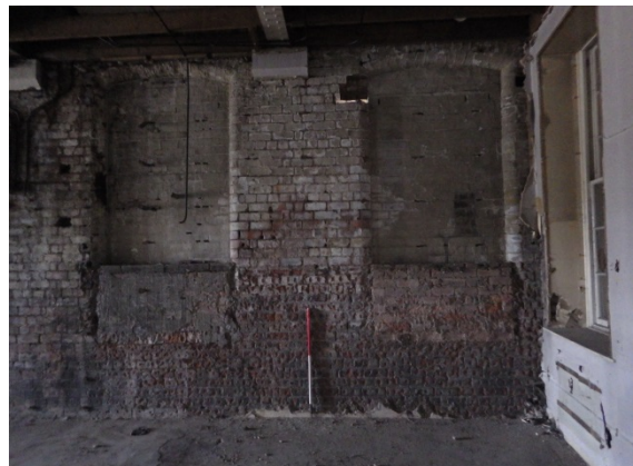
Plate 54 Windows 008 and 009, blocked in Phase 2B. Facing SW
