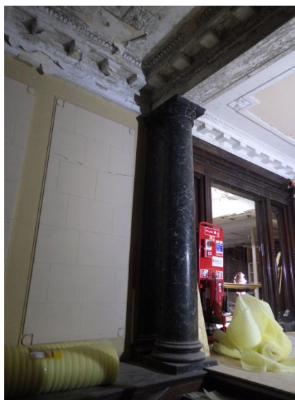
Plate 40 Rubber-clad column, main entrance hall.
