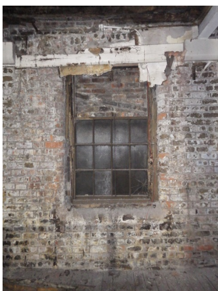
Plate 69 First floor interior, blocked window 002 with lean-to pitched roof bricks 126. Facing SW.
