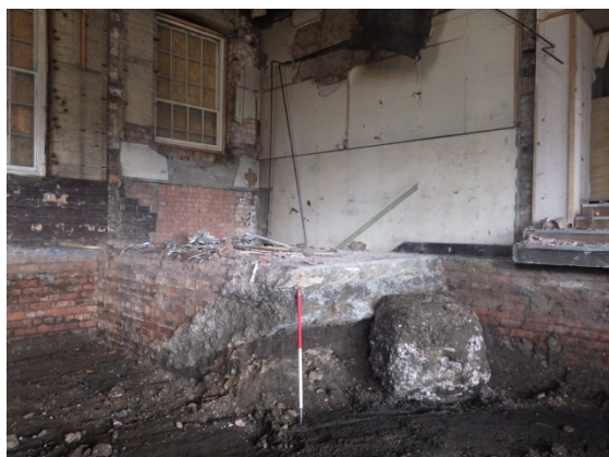
Plate 33 Brick and concrete-blocked staircase with brick-blocked door 116 in background.
