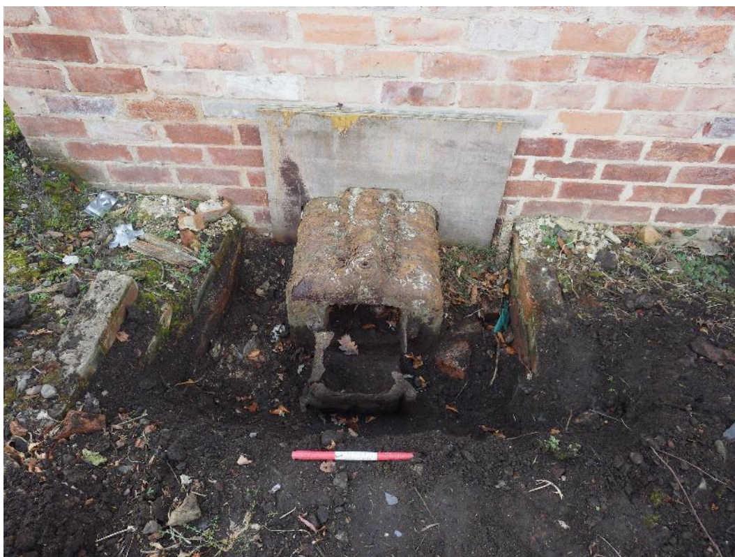
Plate 1 glasshouse boiler, looking south-west
