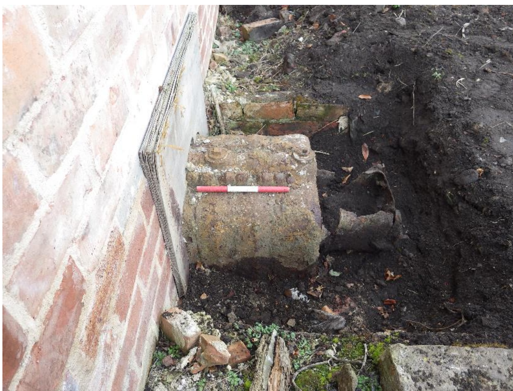
Plate 2 glasshouse boiler, looking north-west
