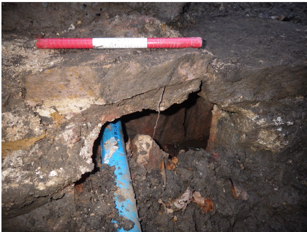
Plate 5 heated flue and hollow interior, looking south-west
