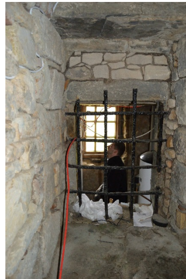
Plate 22 Component 4, basement window detail (photo 100)
