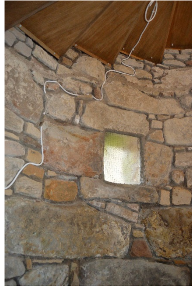
Plate 26 Component 4, ground floor window detail (photo 211)
