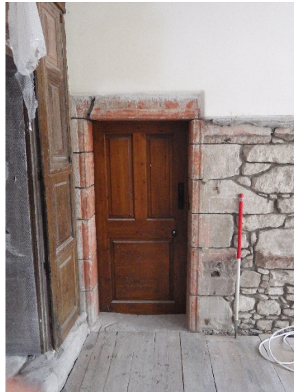
Plate 16 Component 21, east entrance detail (photo 015)
