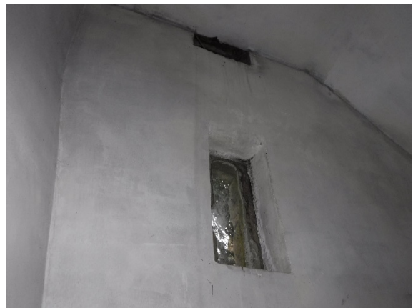
Plate 28 Component 4, first floor window (photo 300)
