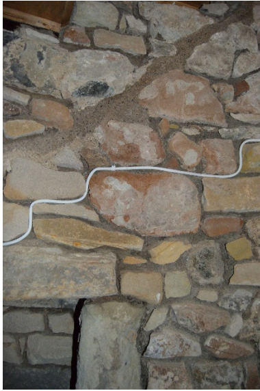
Plate 25 Component 4, pointing detail (photo 200)
