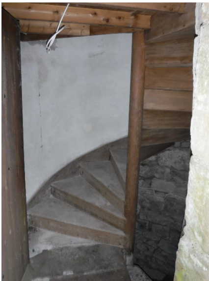
Plate 27 Component 4, ground floor (photo 280)
