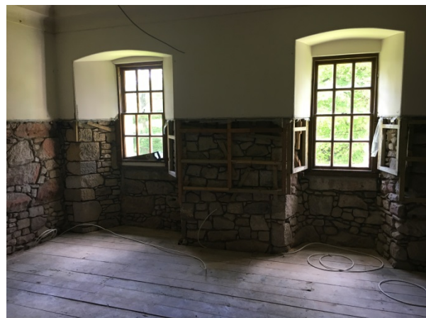
Figure 4: South wall, room 21 with dado panelling removed
