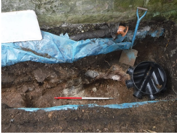
Plate 11 Foundations [013], end of excavation (photo 337)
