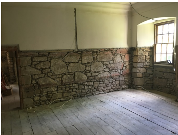
Figure 3: East wall, room 21 with dado panelling removed
