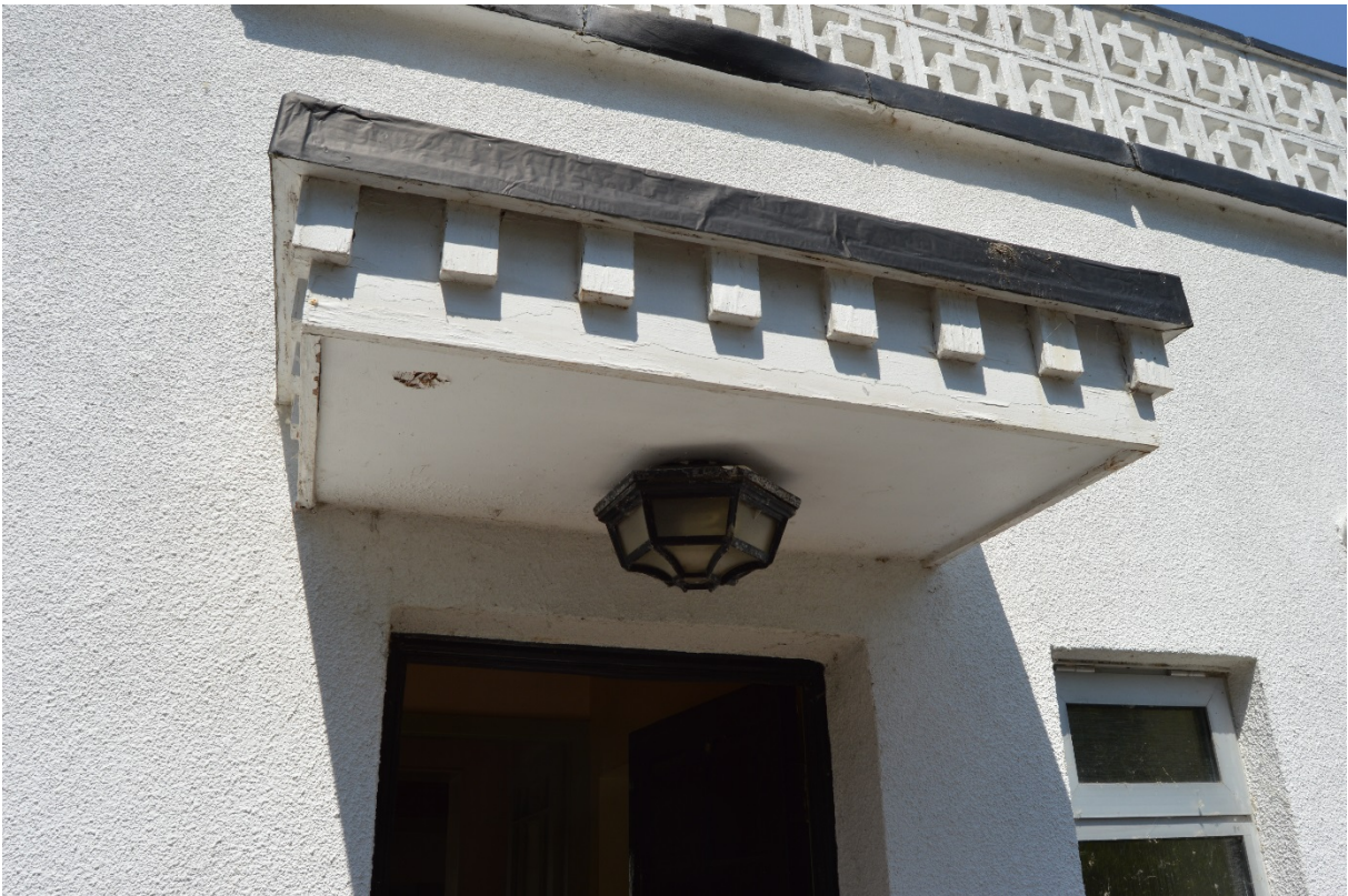
Plate 12 Porch light, southern entrance (photo 082)
