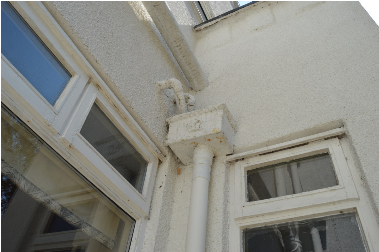
Plate 10 Drainage hopper, west elevation (photo 053)
