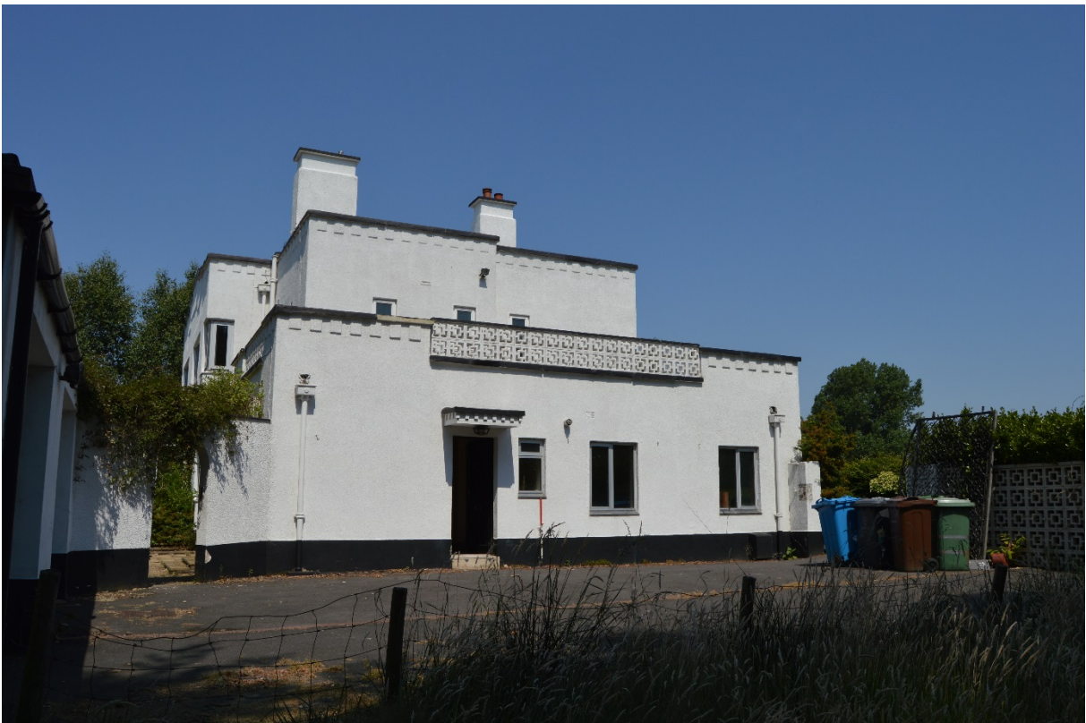
Plate 6 South elevation of Greenridges (photo 017)
