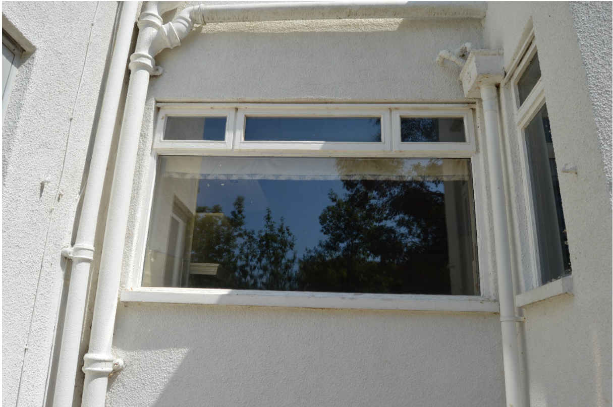
Plate 9 Original casement window, west elevation (photo 054)
