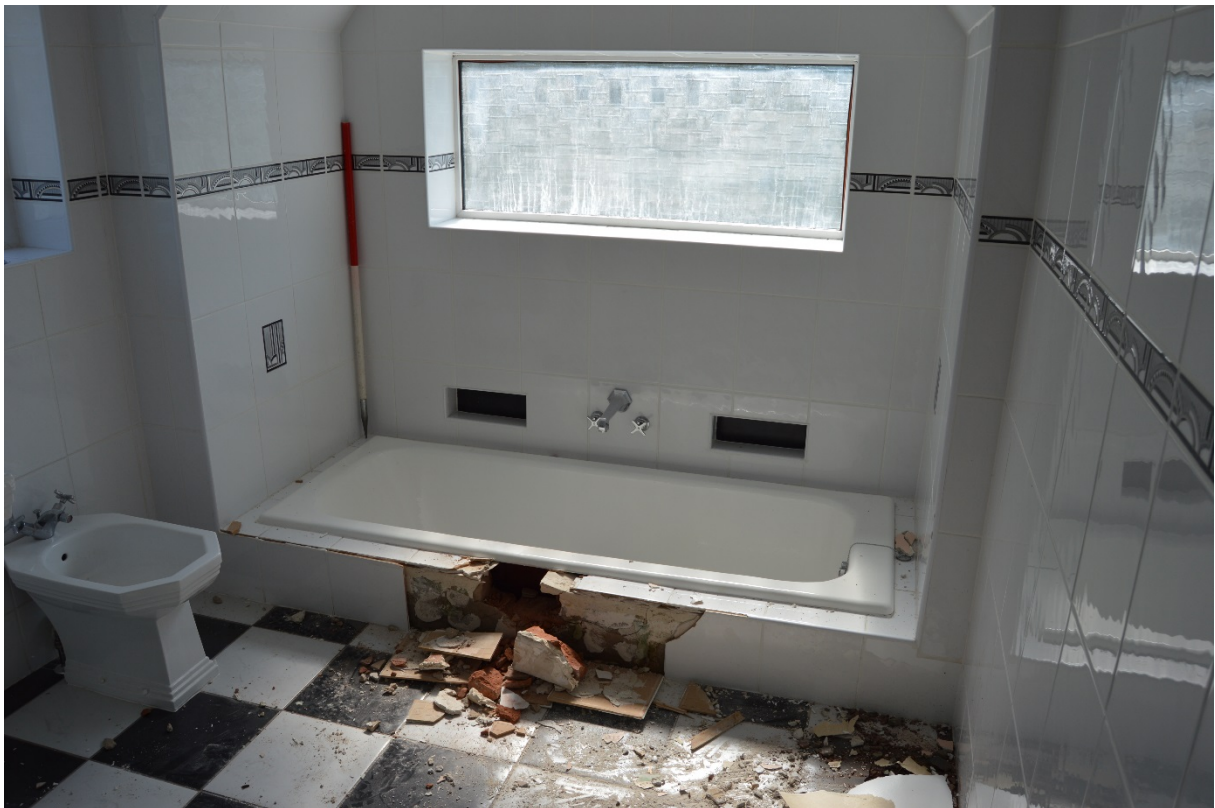
Plate 26 Bathroom, first floor (photo 340)
