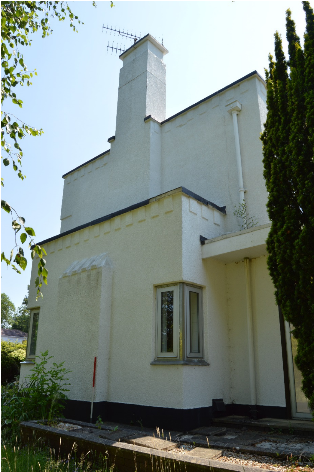
Plate 4 North elevation of Greenridges (photo 027)
