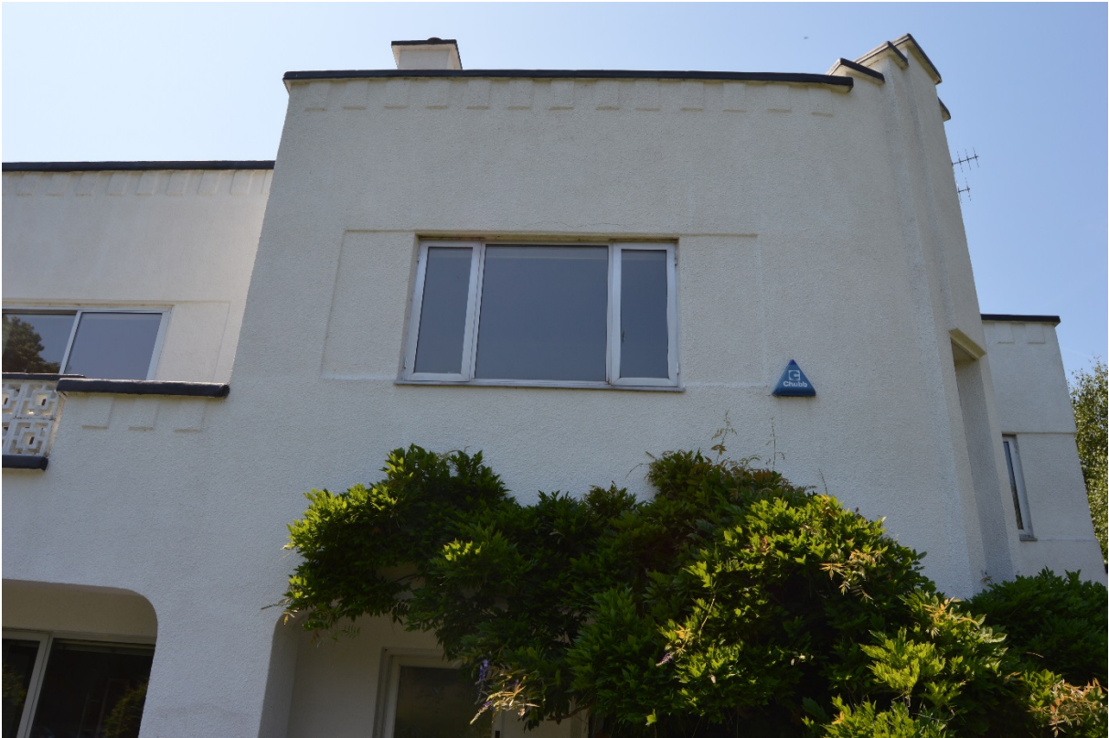
Plate 7 Casement window, principal elevation (photo 068)
