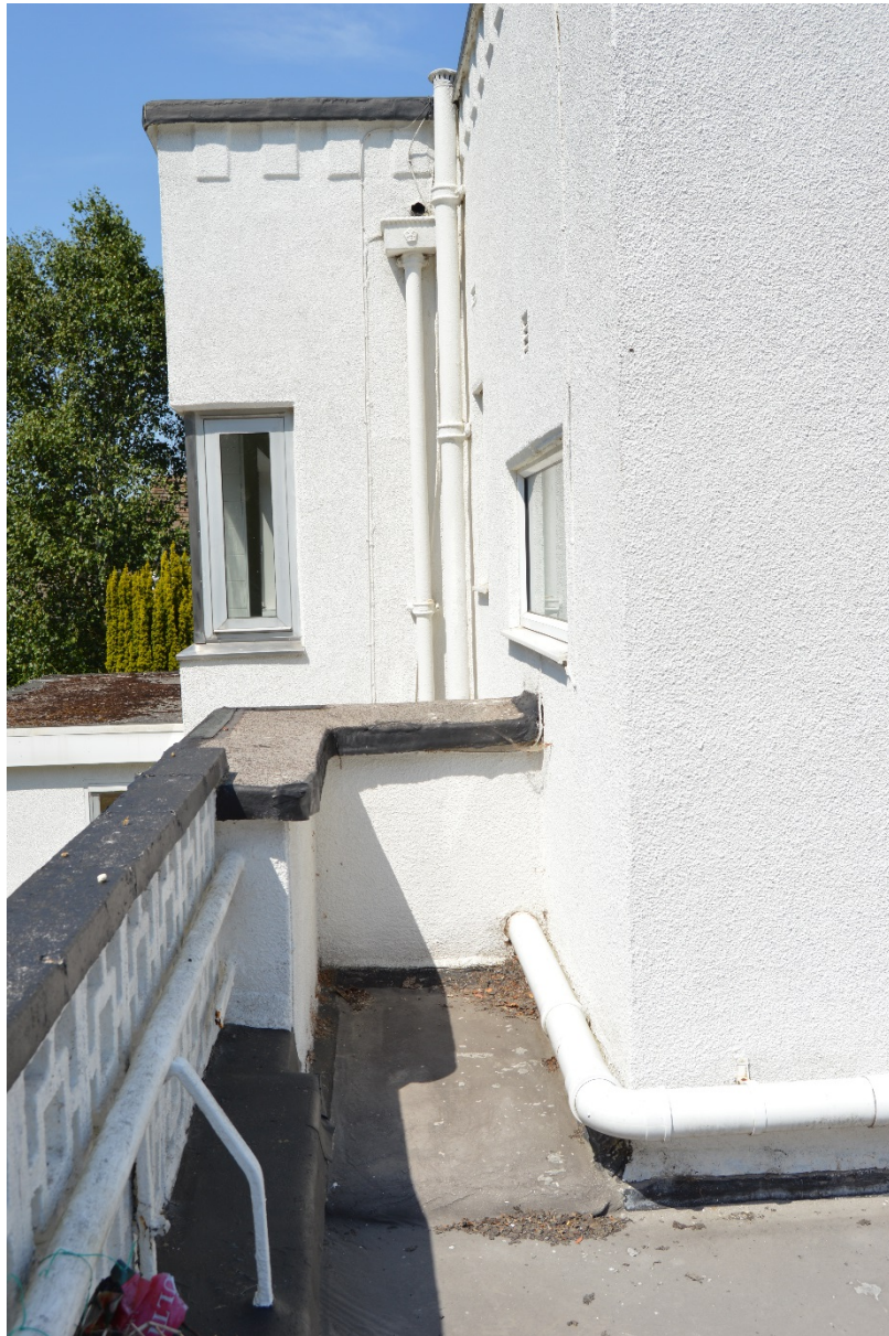
Plate 28 Roof terrace, first floor (photo 130)
