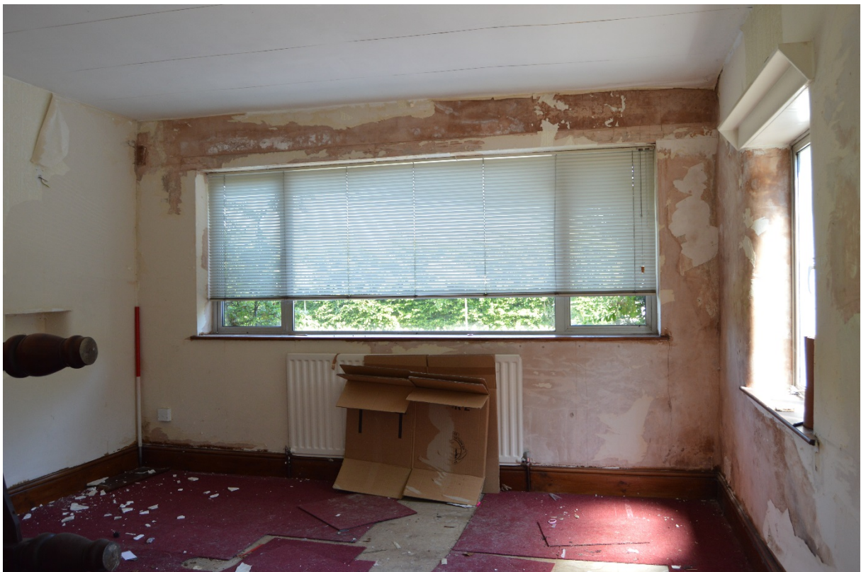
Plate 18 Games room, former integrated garage (photo 141)
