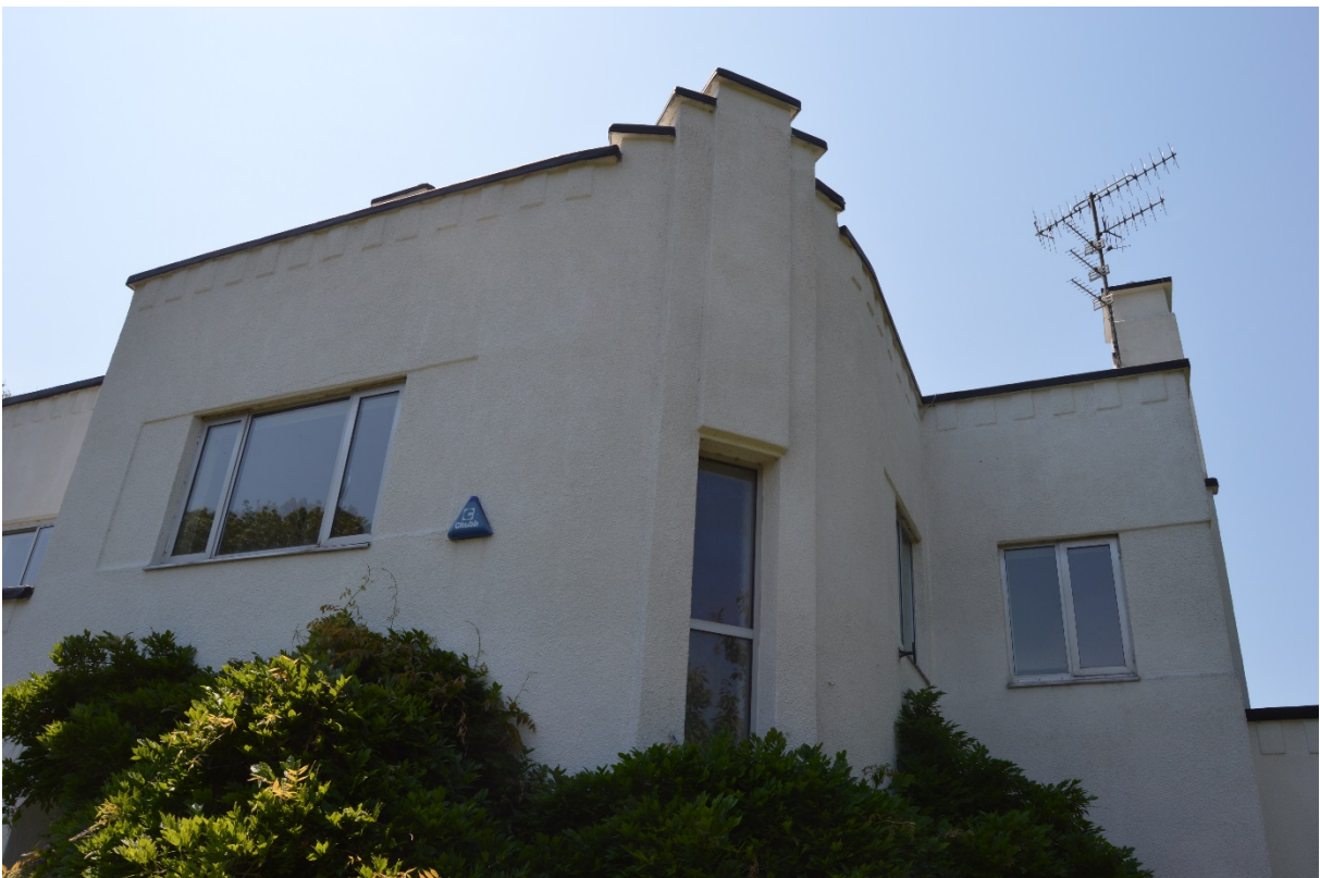
Plate 8 Casement window, north-east corner (photo 067)
