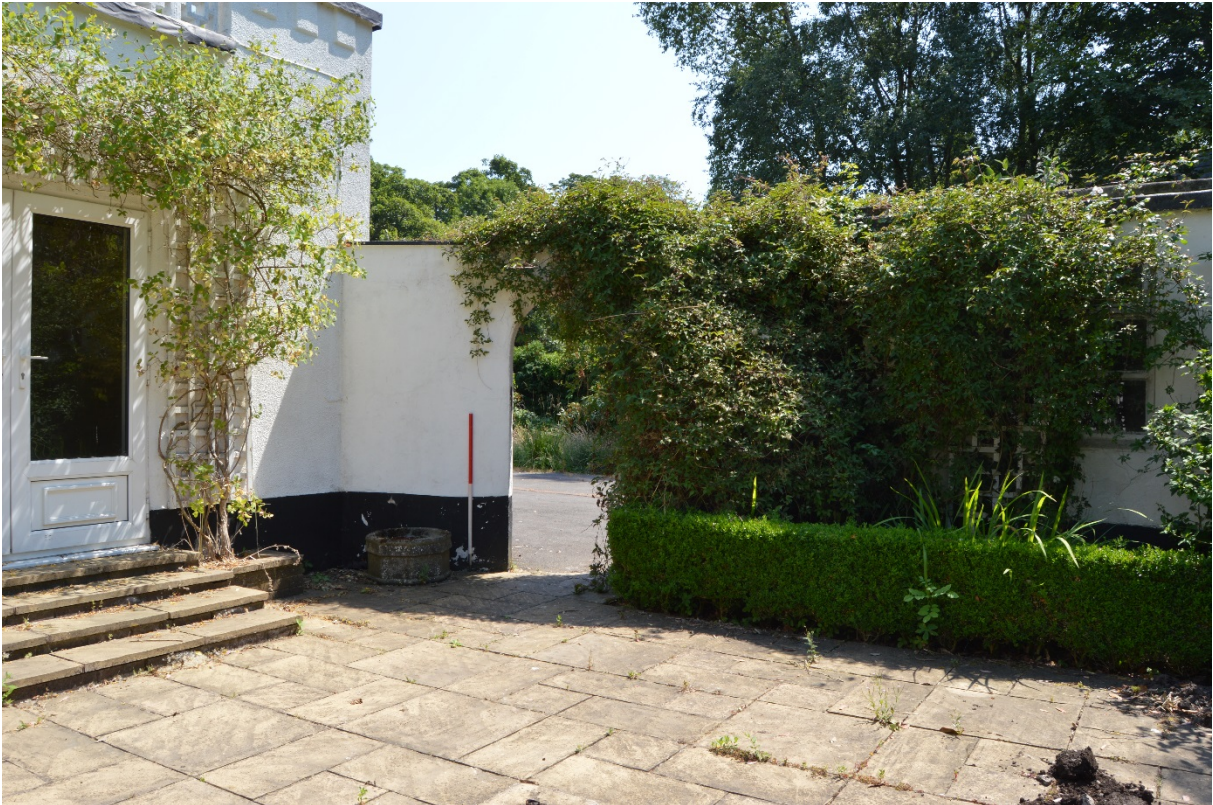
Plate 30 Panel wall linking house to garages (photo 049)
