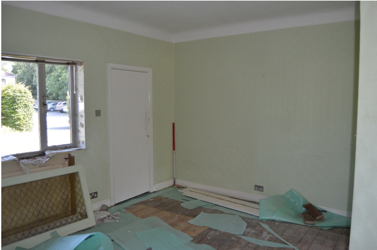
Plate 14 Morning Room, ground floor (photo 191)
