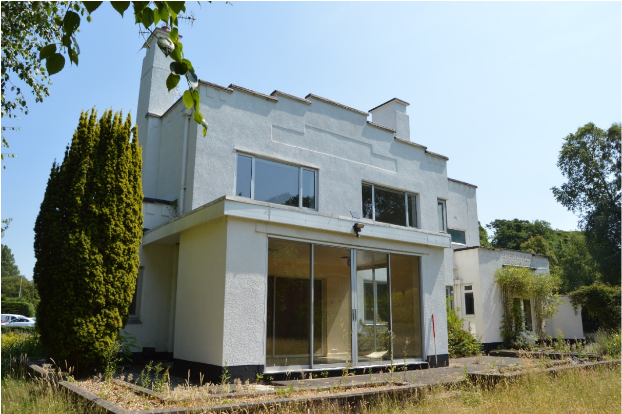
Plate 11 Inset panel, first floor west elevation (photo 024)
