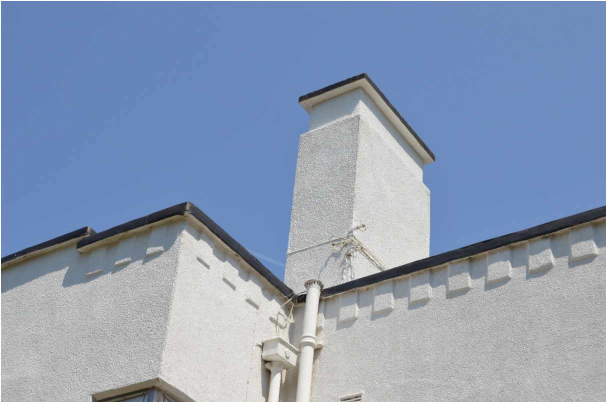
Plate 3 Detail of chimney stack (photo 089)
