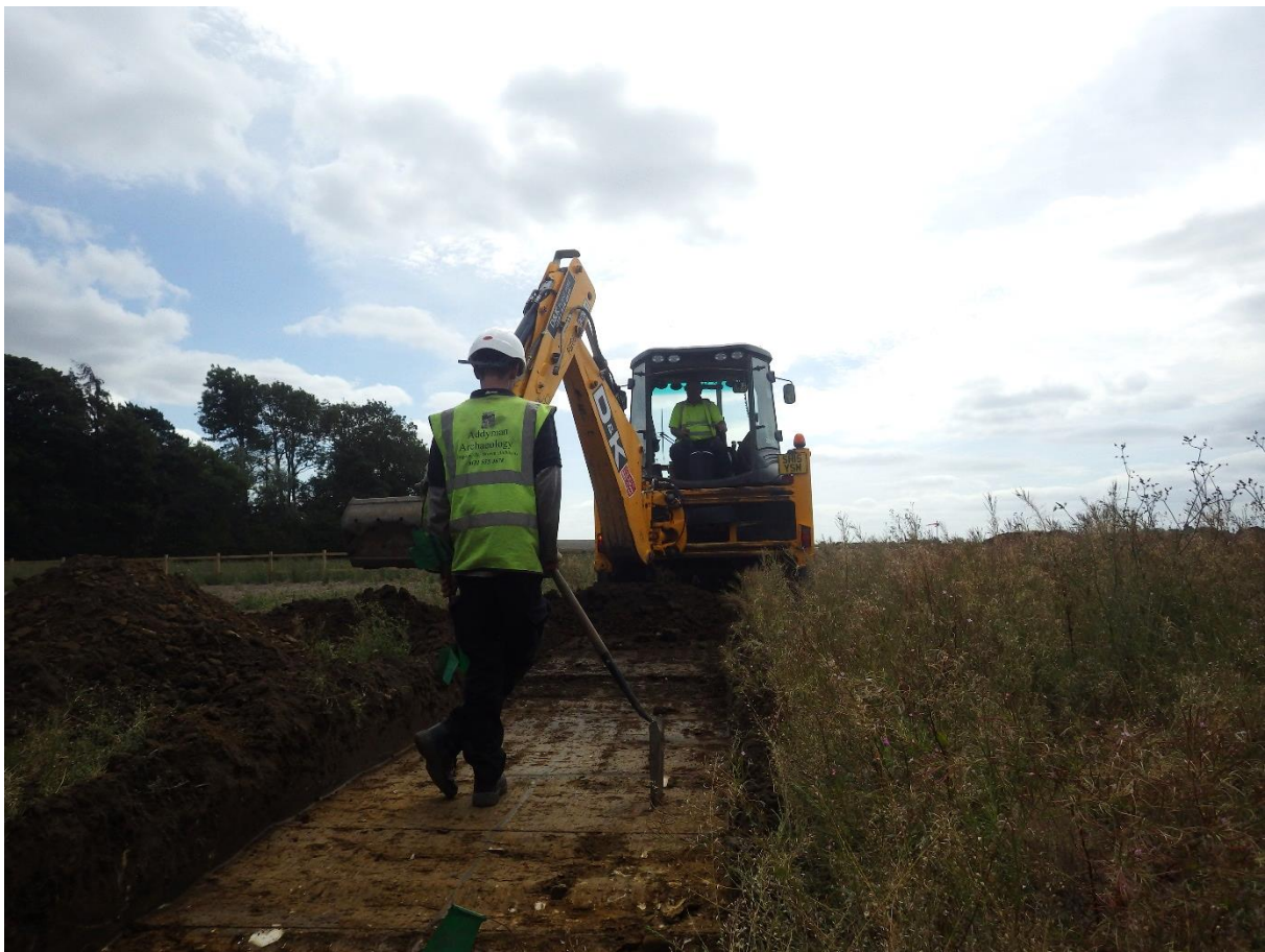
Excavating the trenches
