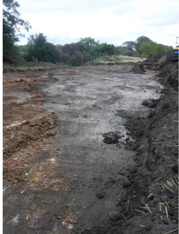
Plate 2 Ramp area, looking north-west showing linear feature [010]
