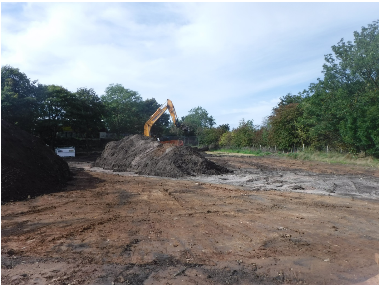
Excavation in progress
