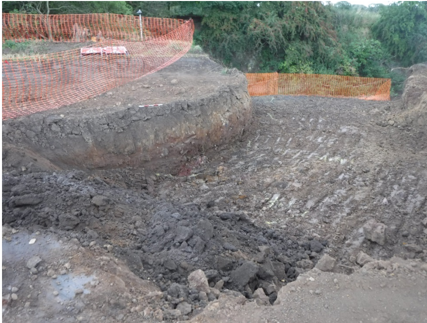
Plate 5 Excavations for ramp at north-west end, showing feature [011] in section
