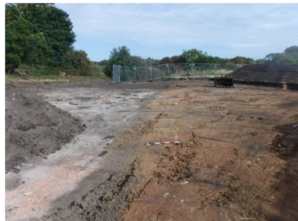
Plate 4 Ramp area, looking north-west, showing linear feature [010] from other side of spoil heap
