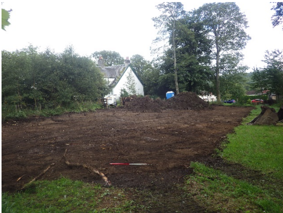
Plate 3 General view of the site after stripping, looking east
