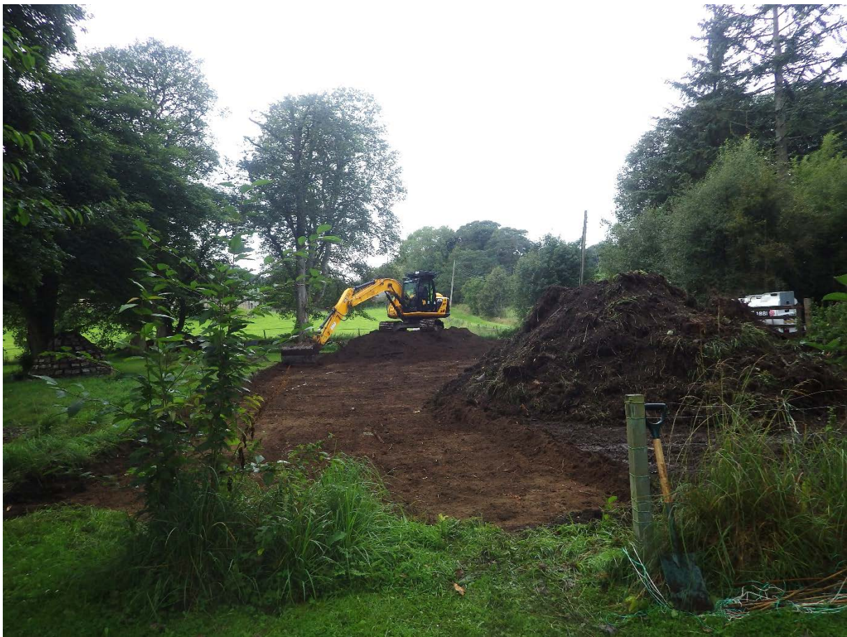
General view of the site
