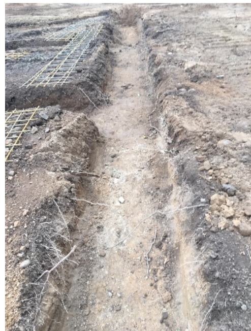
Plate 8 View of excavated foundation trenches
