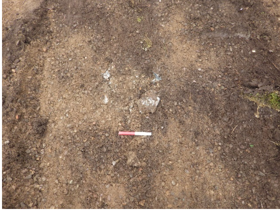
Plate 5 Construction material dump: Type 1
