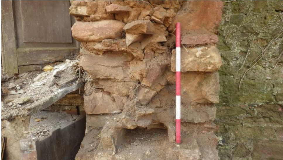
Plate 7 Buildings 4 wall showing junction between clay and lime mortar, (0260)
