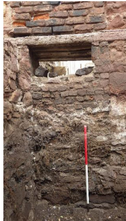
Plate 4 Blocked doorway window between Buildings 1 and 2. (0232)
