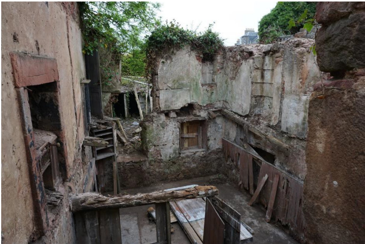
Building 4, looking west
