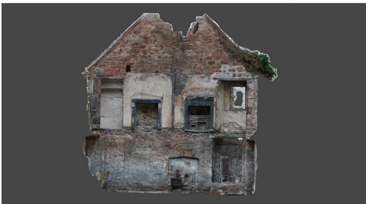
Figure 9 West interior elevation of Building 1
