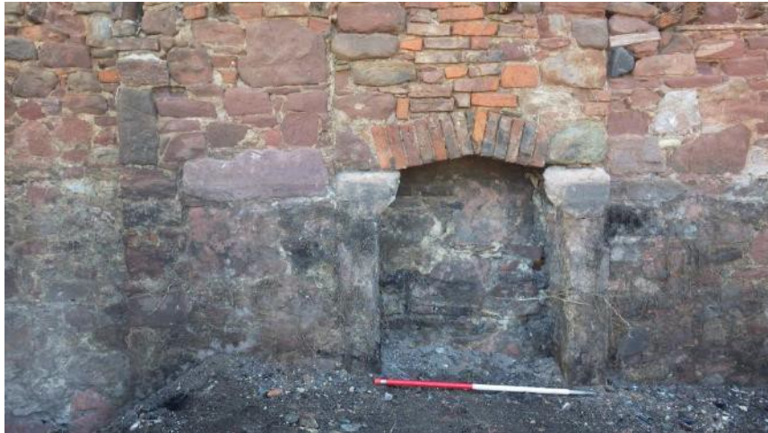
Plate 5 Fireplace in Buildings 3. (0278)
