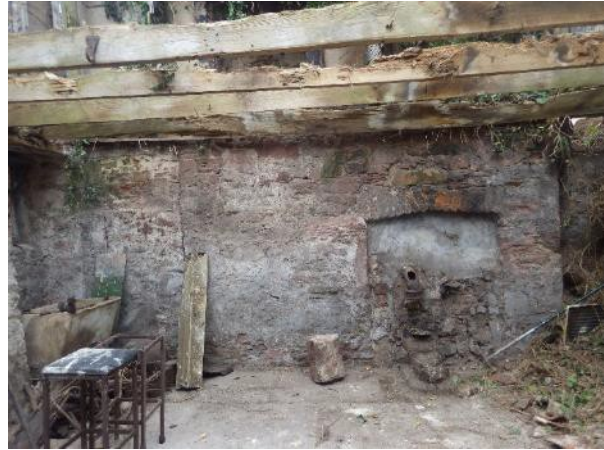
Plate 2 West wall of Building 1 (0160)
