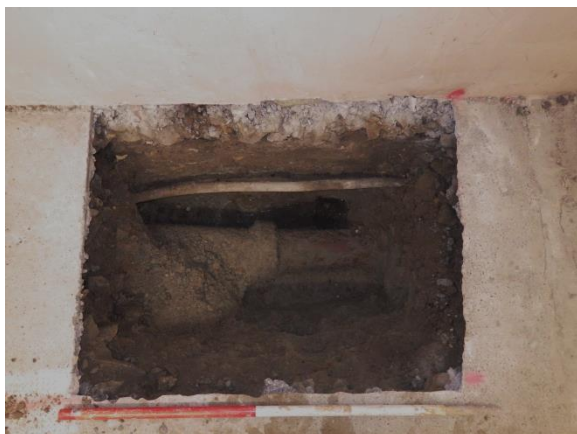
Plate 9 Trial Pit 5, General View
