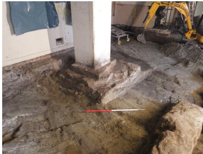
Plate 13 Pillar Sandstone Foundations [057]
