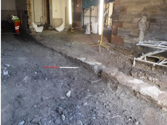
Plate 11 Sleeper Wall [024], showing Break for Ceramic Drain
