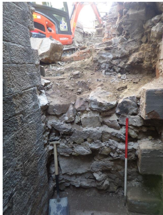
Plate 30 General view of excavations of southern courtyard, rubble blocking
