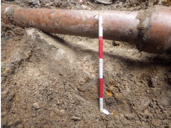
Plate 21 Drain [048] showing Cut in Bedrock
