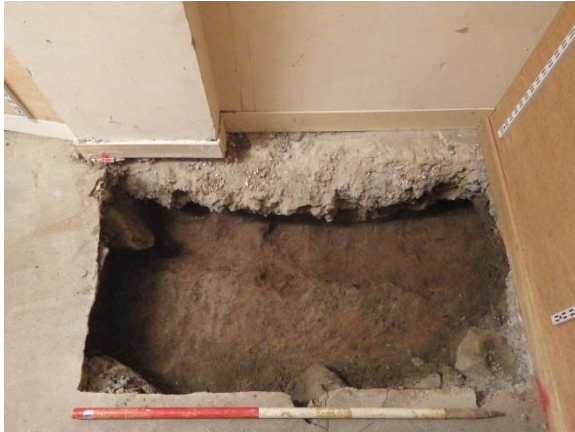
Plate 5 Trial Pit 3, General View
