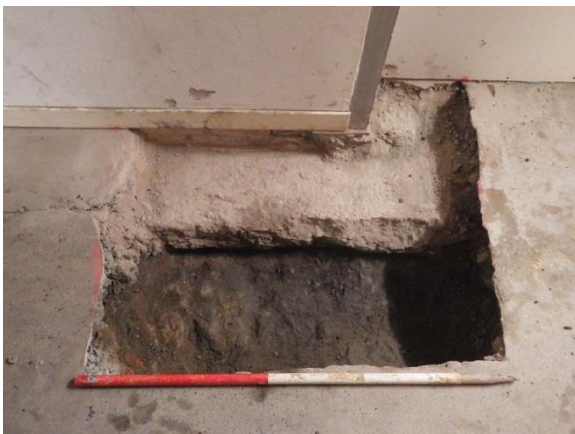
Plate 7 Trial Pit 4, General View
