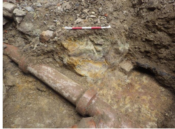
Plate 22 Drain [045] and Cut [055]
