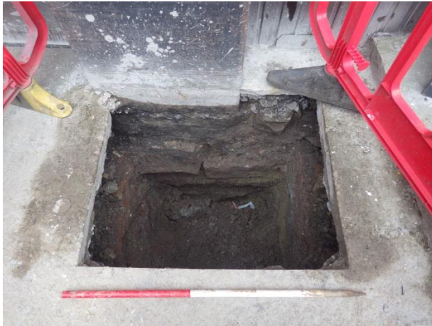
Plate 1 Trial Pit 1, General View
