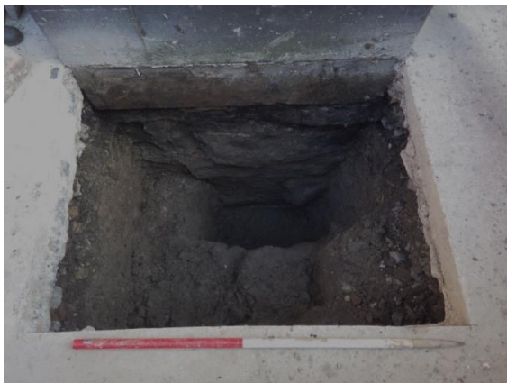
Plate 3 Trial Pit 2, General View
