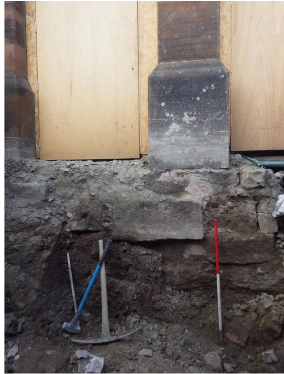
Plate 28 Exposed foundations of school building from southern courtyard excavations
