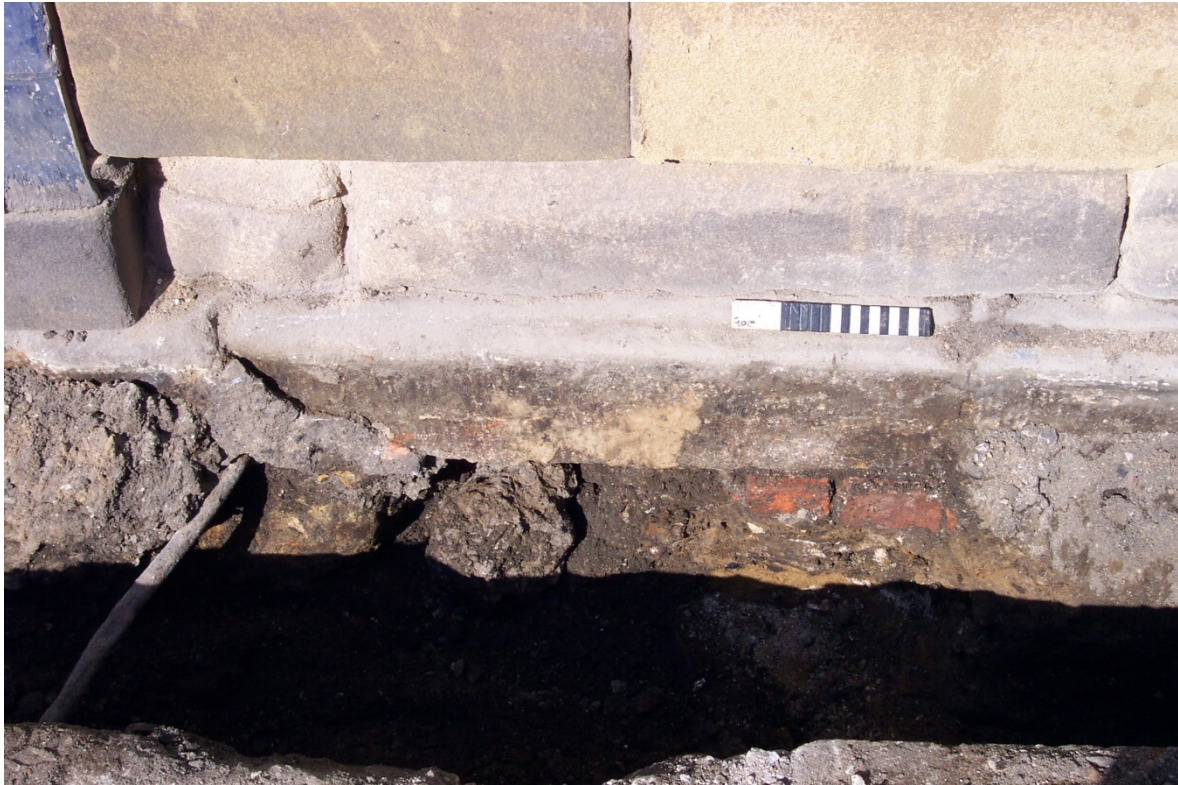
Plate 27 Wall foundation exposed below ground, 20cm scale
