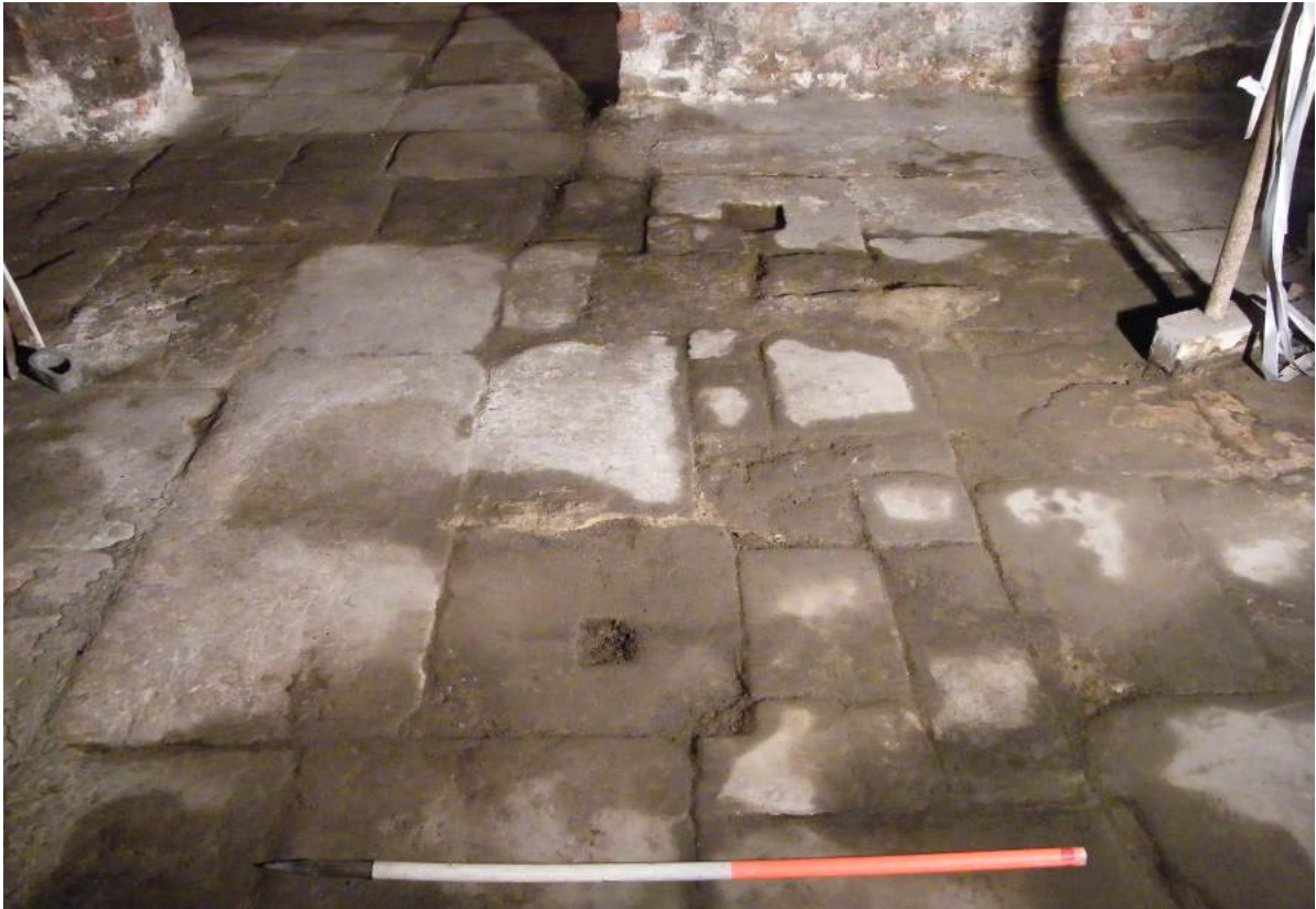
Plate 13 Flagstone flooring within the central part of the rear room, looking south
