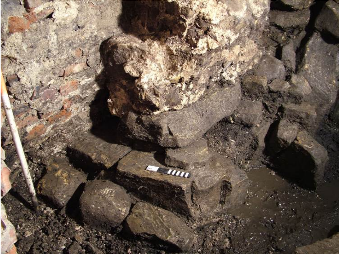
Plate 18 Wall footing 052, sectioned with drain [080] mid ground and alignment of 3 stones to left
