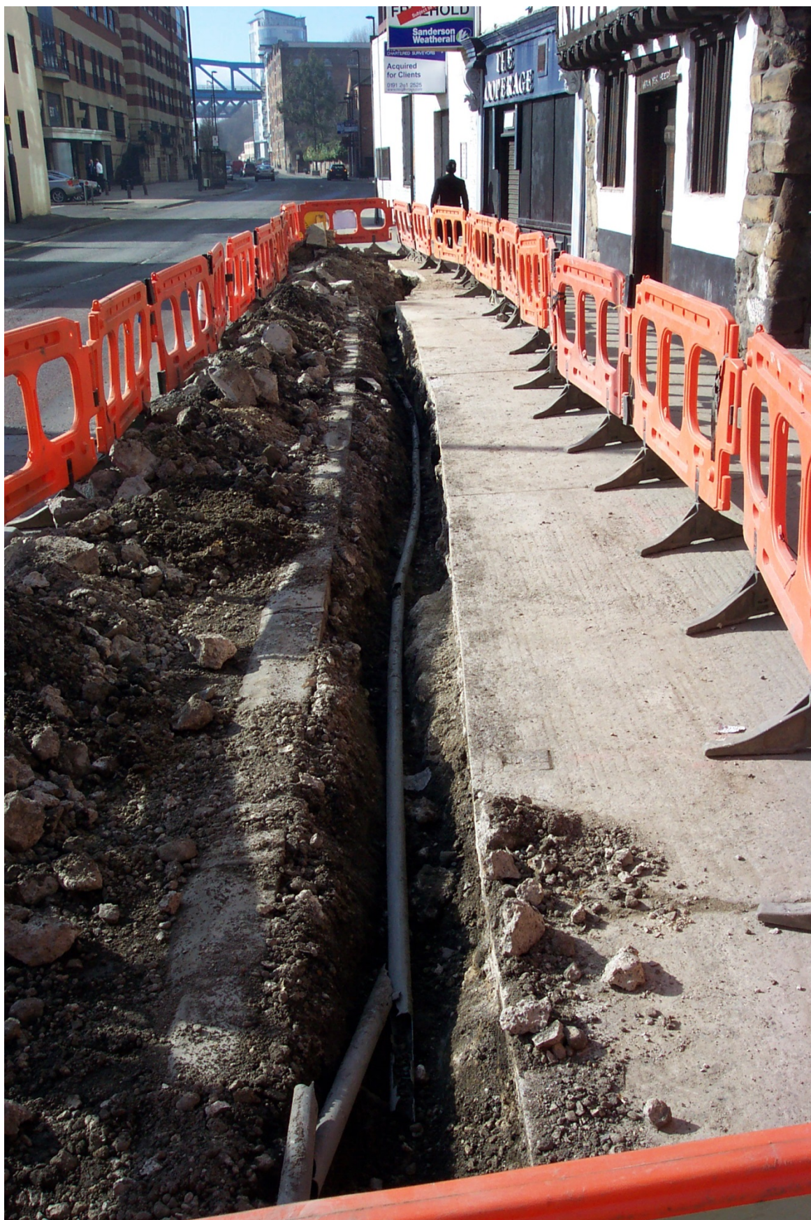
Plate 28 Trench extending westwards along the street frontage showing exposed cable(012).
