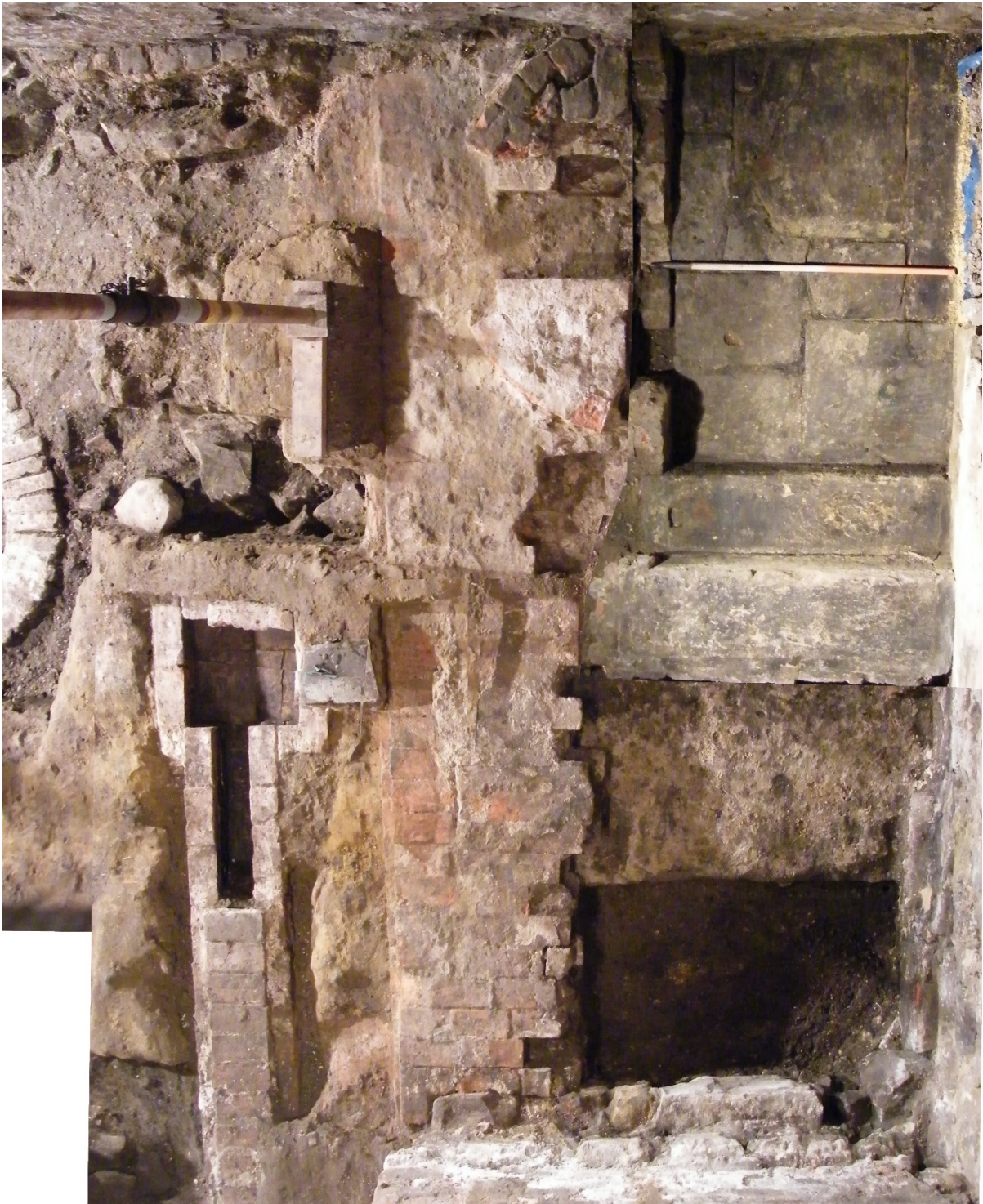
Plate 8 Vertical view of the eastern side of the excavation area showing the surviving extent of the (014) brick platform, the later sunken stair and paving to top right (005, 043) and later drain to lower left (010); north at top
