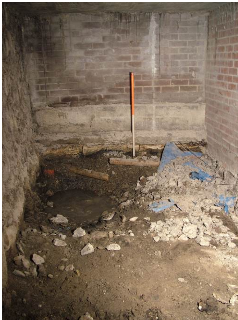
Plate 16 Pre-excavation view of the interior of the north-west room, looking north
