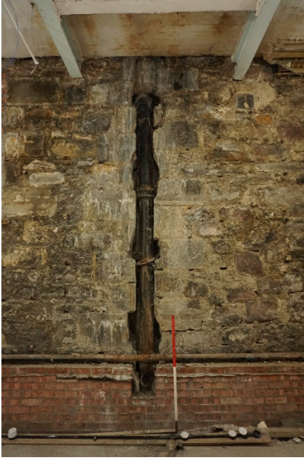
Plate 9 Opening for Downpipe [004]
