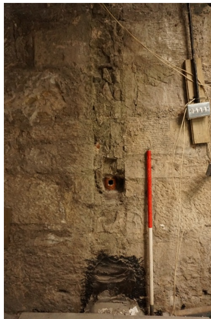
Plate 15 Downpipe within Opening [010]
