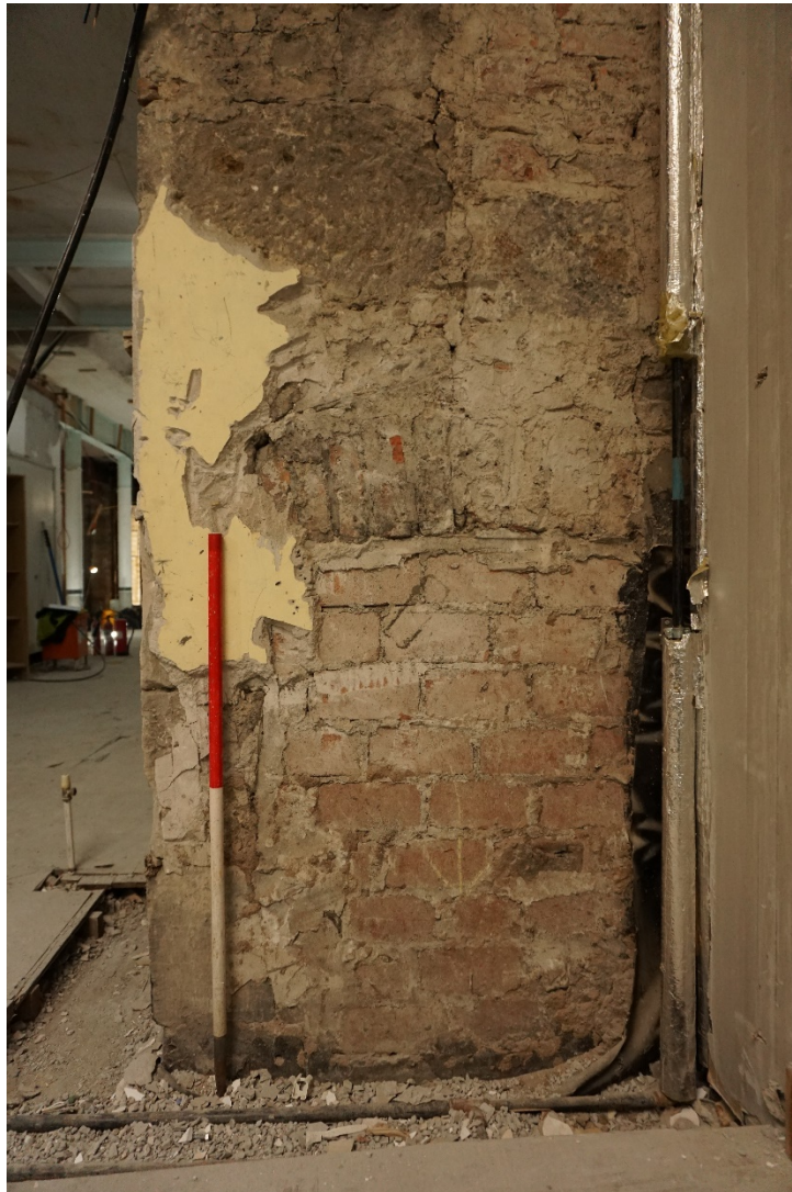
Plate 16 Inserted Fireplace [007] and later Blocking
