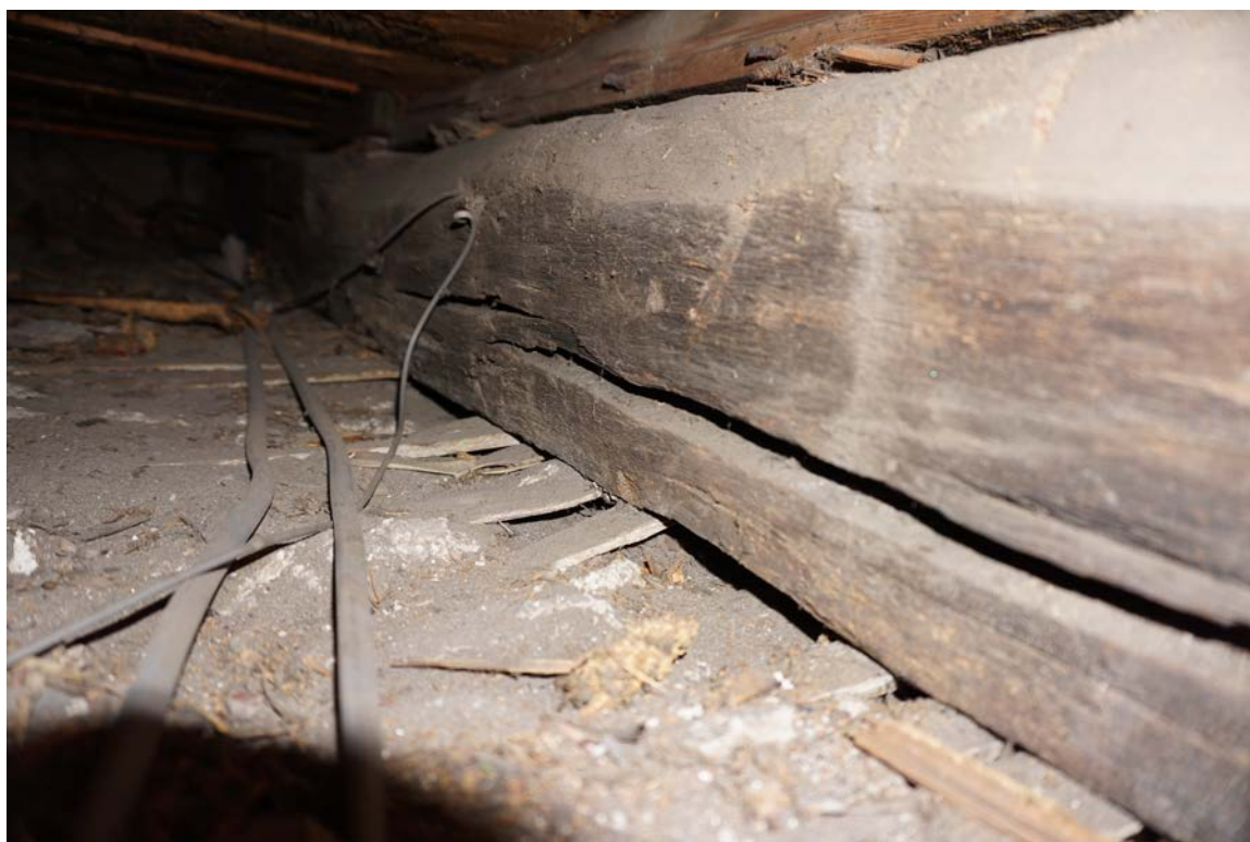
Plate 4 joist 4 showing deep shakes and possibly detached plaster, looking south (photo 24)
