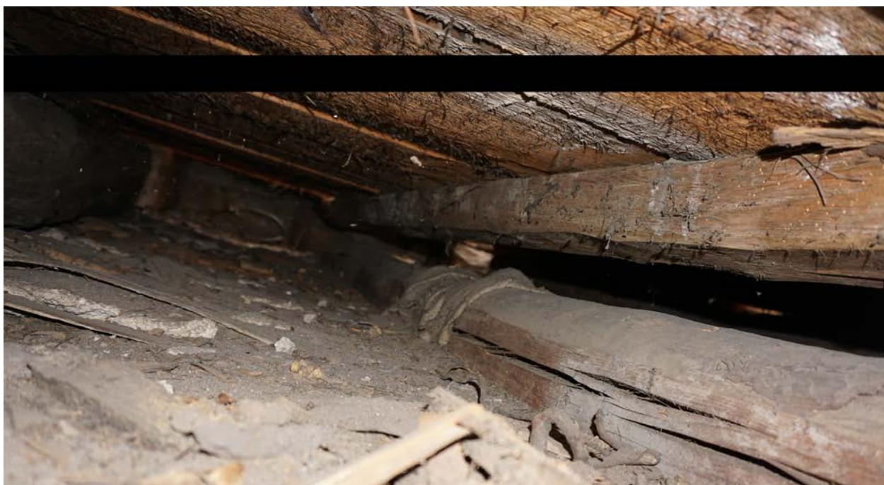
Plate 5 joists 5 and 6, 5 at top right, 6 at bottom right shows gap between, shakes and bark on the timbers, looking south (photo 28)
