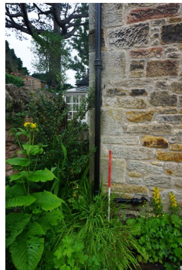
Plate 5 South elevation, ashlar quoins at SW corner
