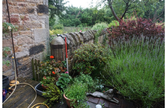
Plate 7 Garden boundary wall with rounded copes and glazed brick wall end.
