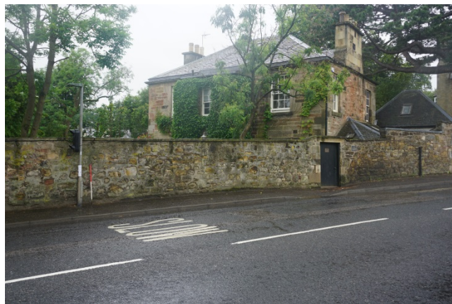
Plate 12 General setting view from east
