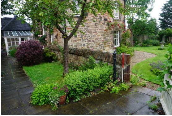
Plate 6 Garden boundary wall with glazed brick gate pier.
