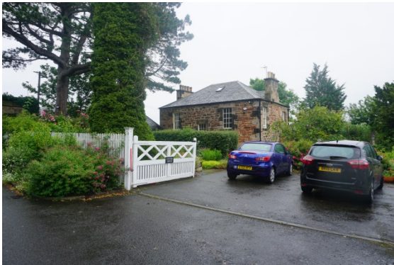
Plate 10 General setting view from west.
