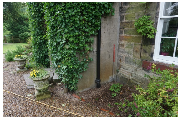
Plate 3 East external elevation with later cement-rendered porch abutting main elevation
