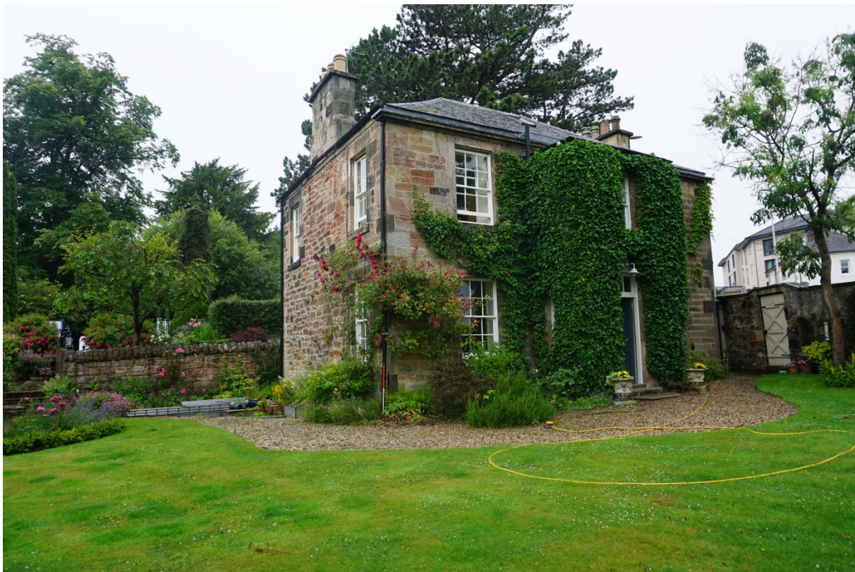
Eskside House from the southeast
