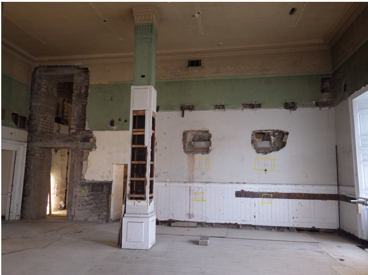
Plate 43 Room 1.294/6, general view with boxed column and west wall; blocked fireplace behind panelling at centre
