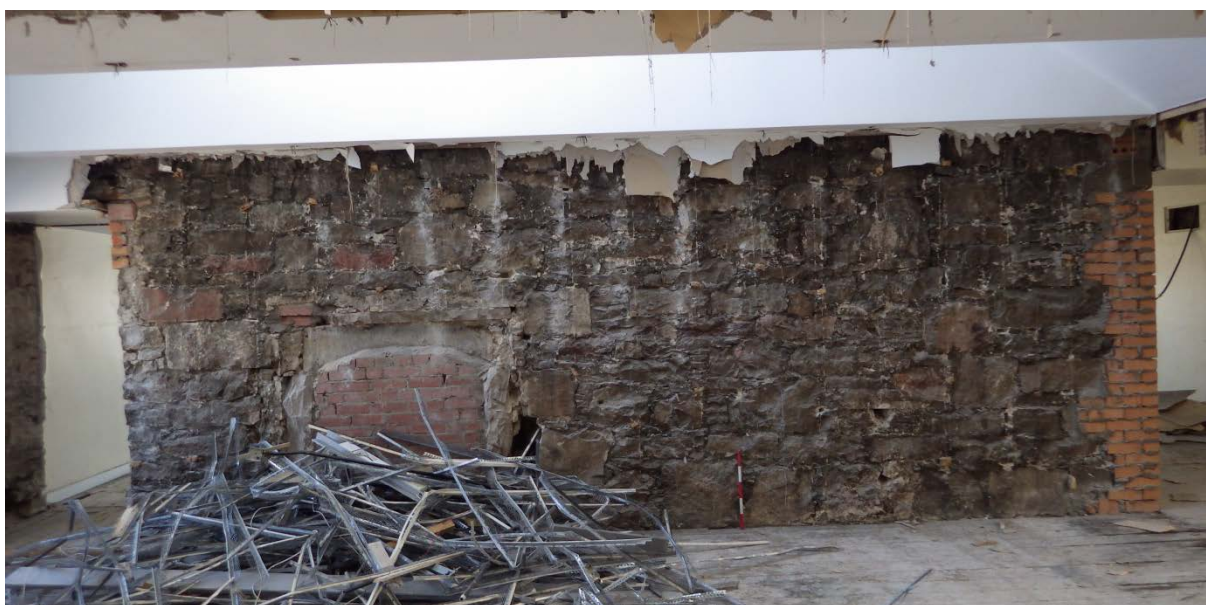
Plate 54 Room 2.361 east wall historic fabric with brick-blocked fireplace
