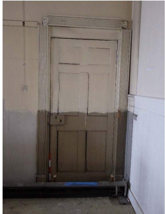
Plate 46 Room 1.298, southern wall showing exposed western relic door, access from the stairs beyond
