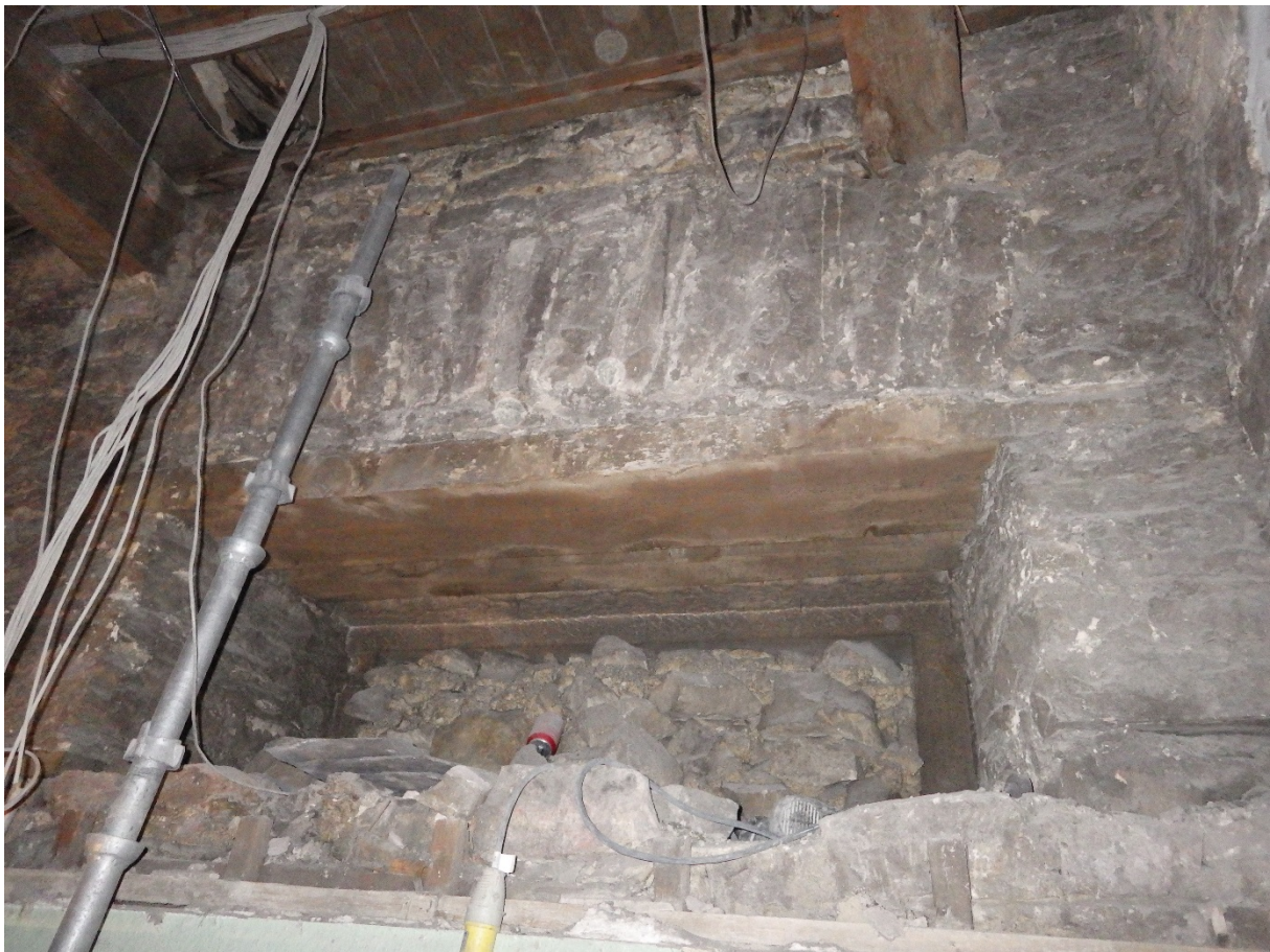
Plate 42 Room 1.Z28A blocked up windows visible above the low ceiling
