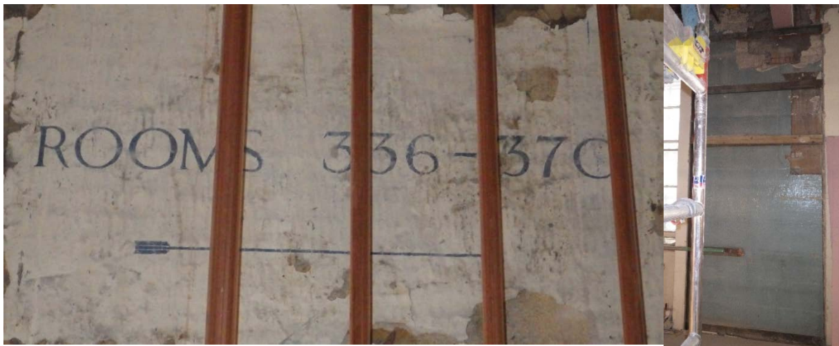
Plate 31 Room 1.278 painted room numbers on stairwell
