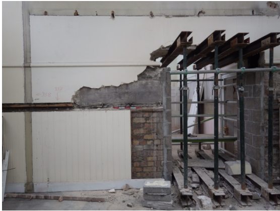
Plate 47 Room 2.Z21 east wall fireplace lintel in situ
