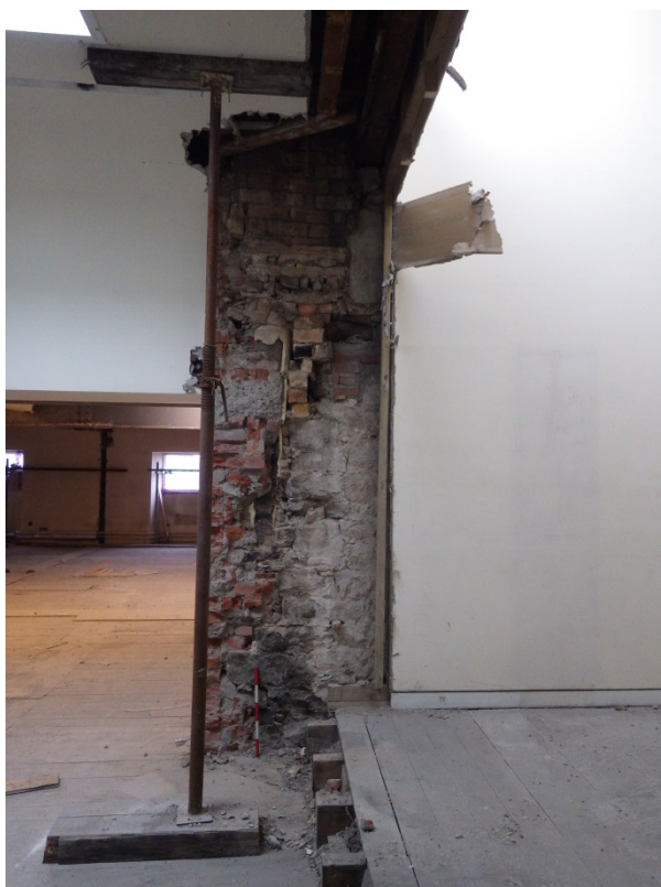
Plate 51 Room 2.344, blocked fireplace and ceramic pipe flue above
