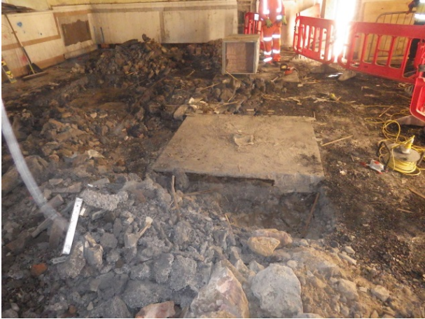
Plate 1 Trench 6 area pre-excitation with concrete surface broken out
