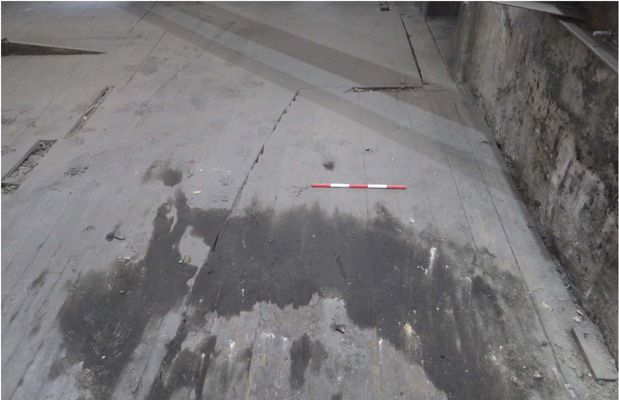
Plate 33 Room 1.288 early floorboards shows curved outline of lecture podium mid frame and rough line of lecture room seating to left (lifted boards) and narrower boards in the passage between.
