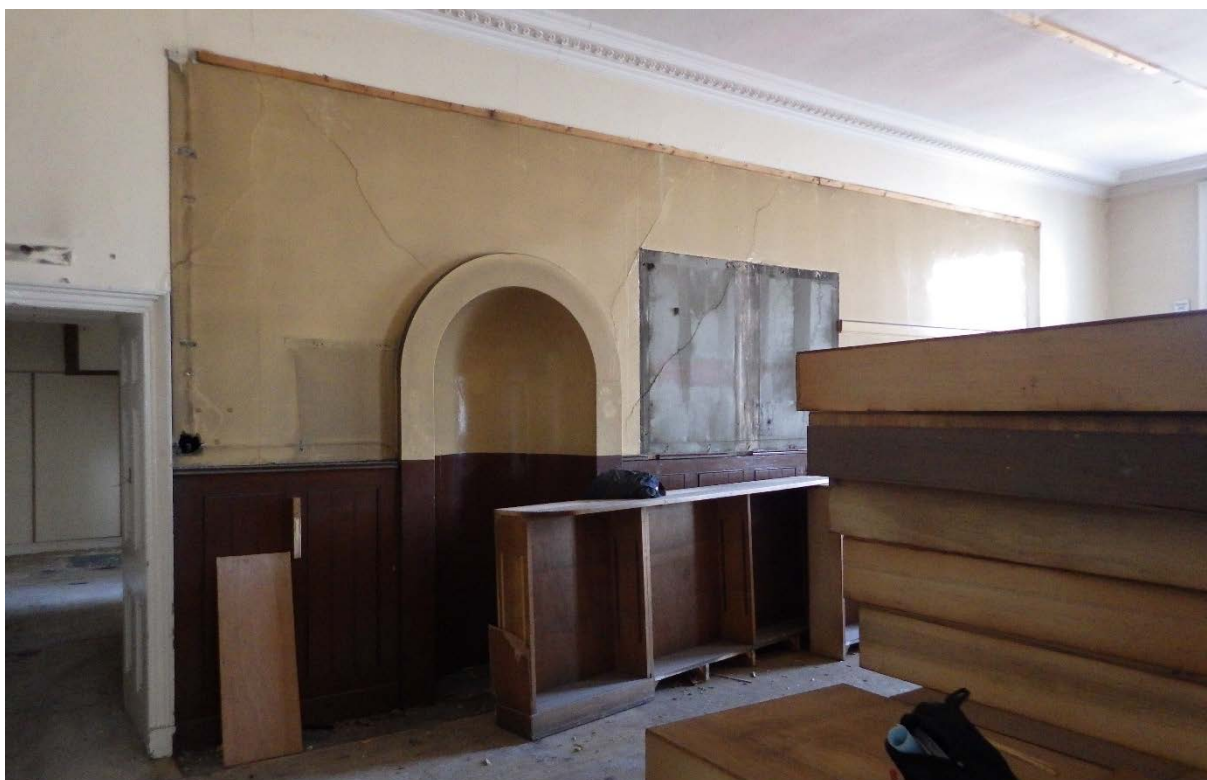
Plate 40 Room 1.292 western elevation shows earlier paint scheme and stove recess
