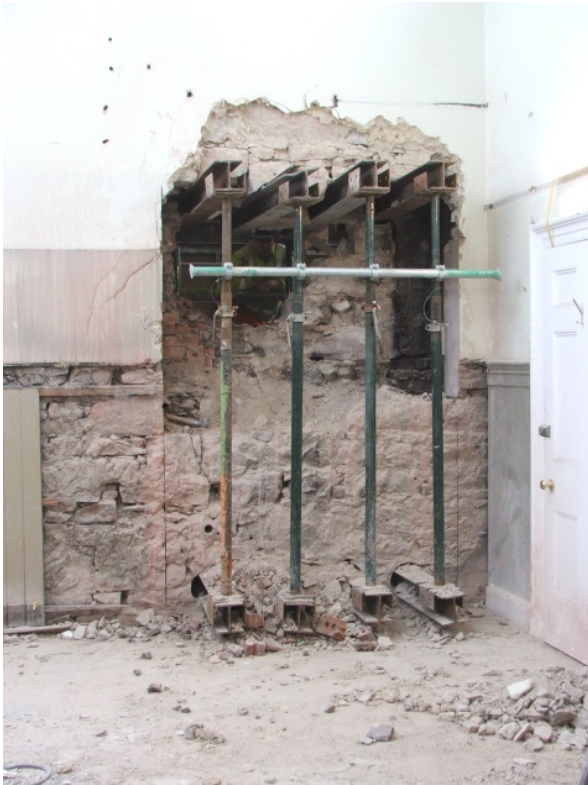
Plate 49 Room 2.340 east wall new door opening with flue exposed at right
