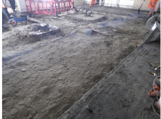
Plate 2 Trench 6 area after removal of concrete showing sleeper walls
