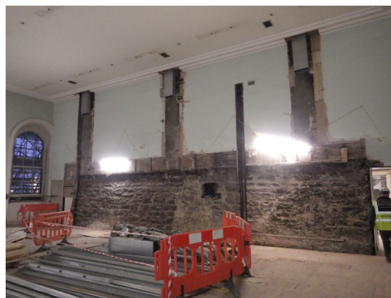
Plate 26 G.183 west wall with earlier dark green painted plaster and exposed rubble wall
