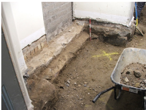
Plate 8 B.Z39-42 stone foundation courses of standing building revealed in ground reduction
