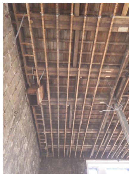
Plate 28 G.188 ceiling structure with integral box vents
