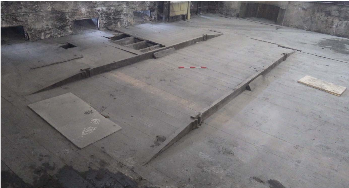
Plate 34 Room 1.288 floor truss rising above original floor
