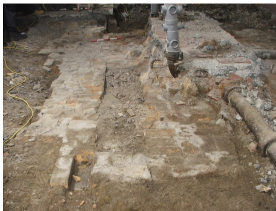
Plate 9 B.Z39-42 brick and concrete foundations
