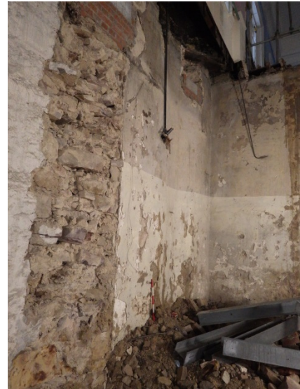
Plate 6 B.Z47 Demolished party wall in foreground with curving relict stair well at scale
