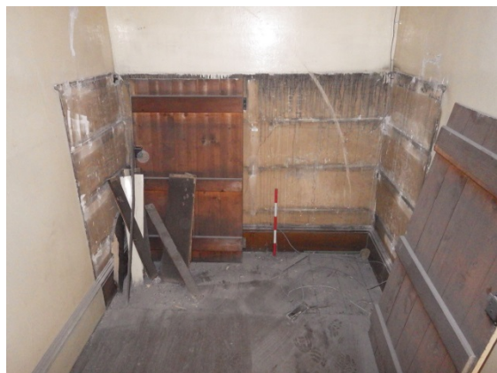
Plate 23 Room G.Z33 with original decorative scheme behind removed shelving
