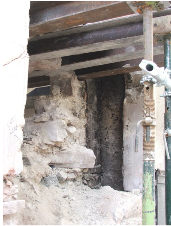
Plate 50 Room 2.340 detail of sooted and heat-affected flue
