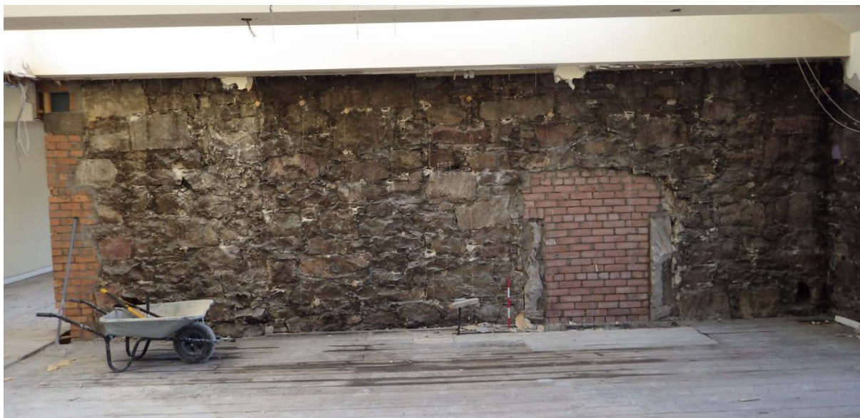
Plate 53 Room 2.360 west wall with blocked fireplace and cut-back cross-wall to right of wheelbarrow
