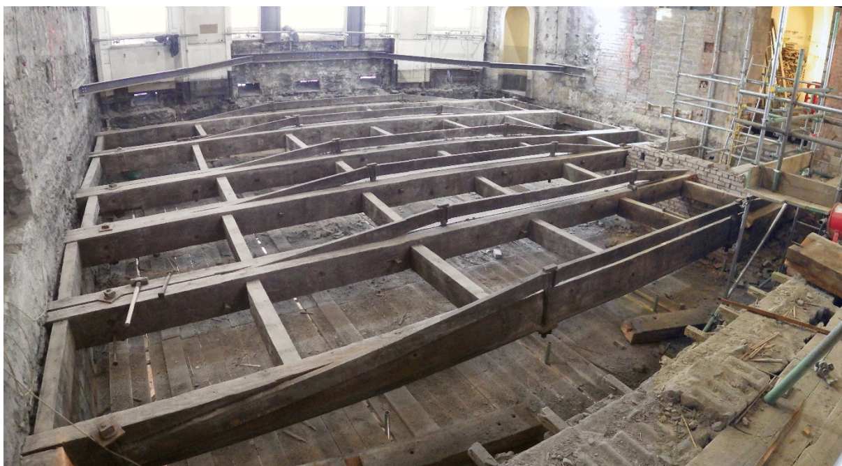
Plate 39 room 1.288 floor structure once floor joists and boarding removed
