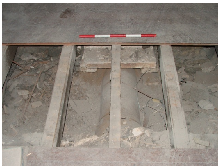
Plate 15 G.151 detail of floor structure with cast iron pipes below
