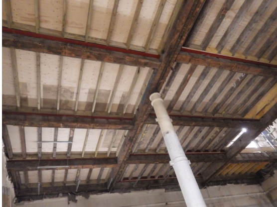
Plate 12 Room B.L05 with ceiling stripped showing floor structure
