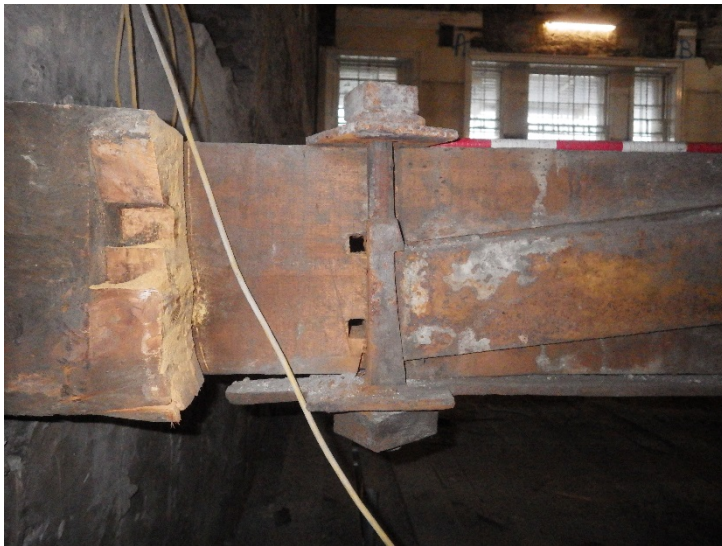
Plate 35 Room 1.288 detail of metal truss end exposed
