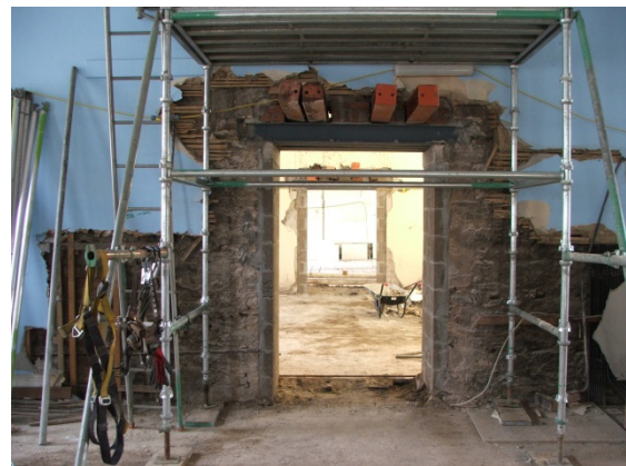
Plate 20 G.159 new opening in wall fabric with fireplace to left
