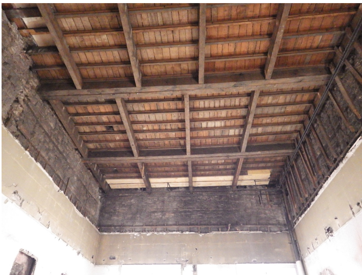
Plate 41 Room 1.292 false ceiling stripped exposing floor structure above and paint scheme
