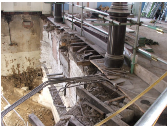
Plate 19 Room G.160/159 floor structure
