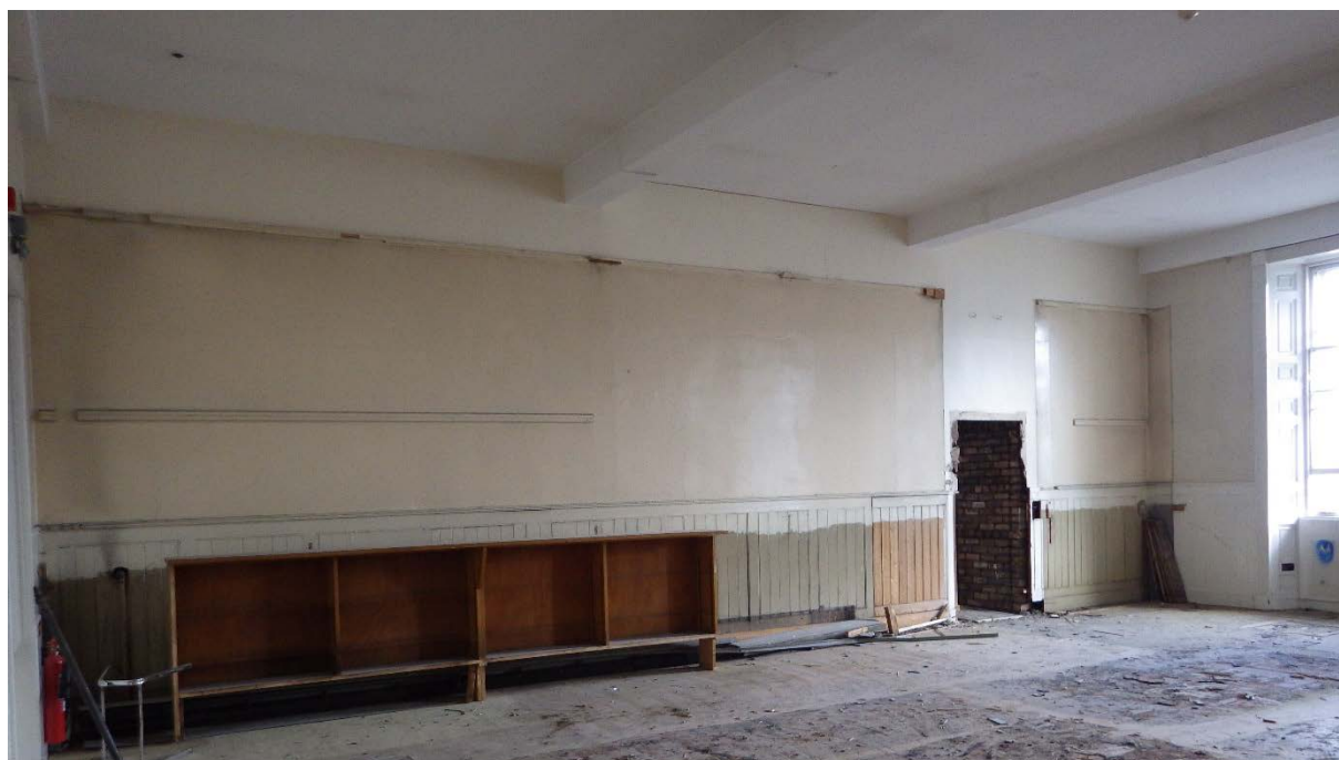
Plate 44 Room 1.298 north wall showing paint schemes
