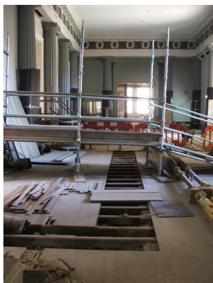
Plate 14 Room G.151 with 'trench' through flooring. Facing N
