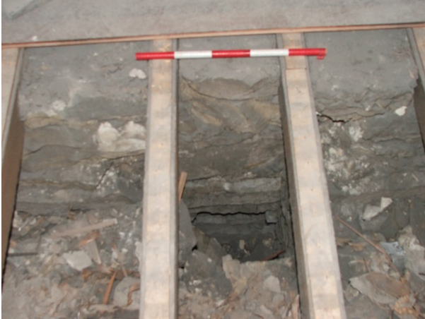
Plate 16 Room G.151 view of stone flue or vent
