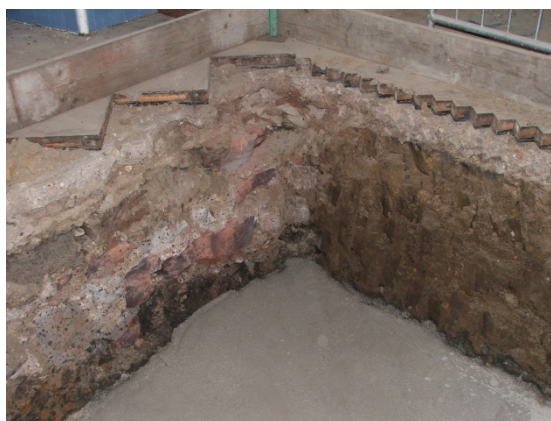
Plate 11 BL05 test pit, NE corner showing early masonry and foundation trench cutting natural clay
