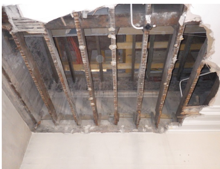
Plate 22 G.175 showing earlier, higher cornice line above existing ceiling
