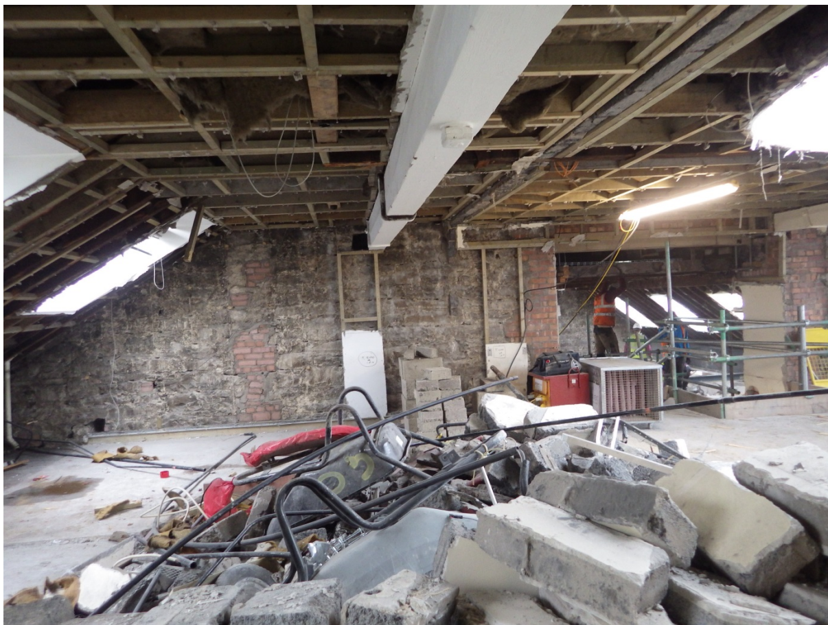
Plate 60 Room 3.413/4 west wall with historic fabric and rood structure exposed
