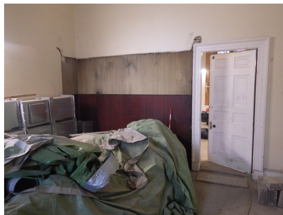
Plate 24 G.180 with earlier dark red and cream decorative scheme exposed below modern paint
