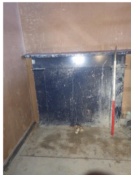
Plate 73 Room 2.1, detail of fireplace.
