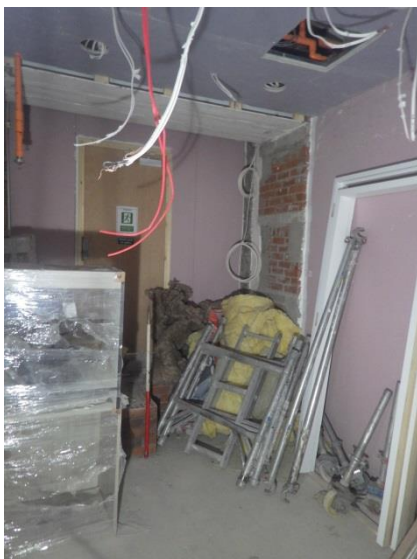
Plate 72 Room 2.1 (south), with Phase 4 brick wall and Phase 5 partitions. Facing NW.
