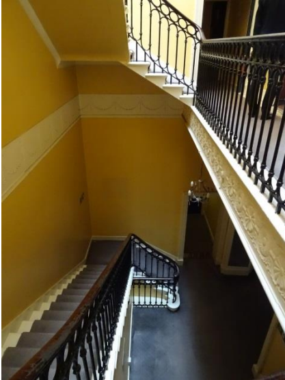
Plate 62 Main stair, decorative moulded plaster. S&B
