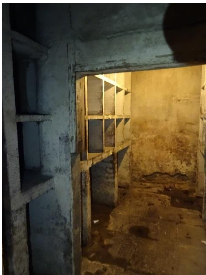
Plate 21 Basement, Room B.4, wine bins. S&B.
