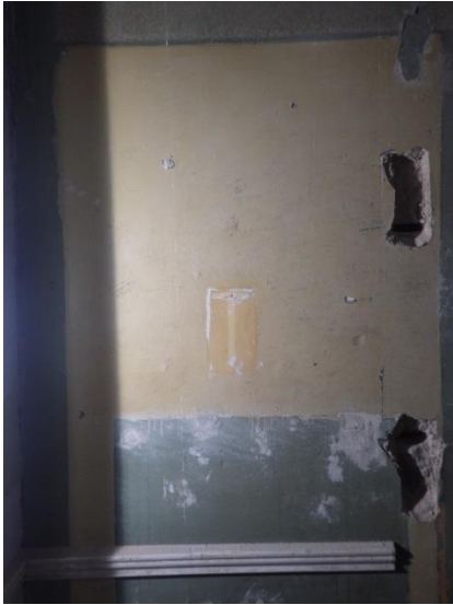
Plate 44 Ground floor Hall, Phase 4 telephone station
