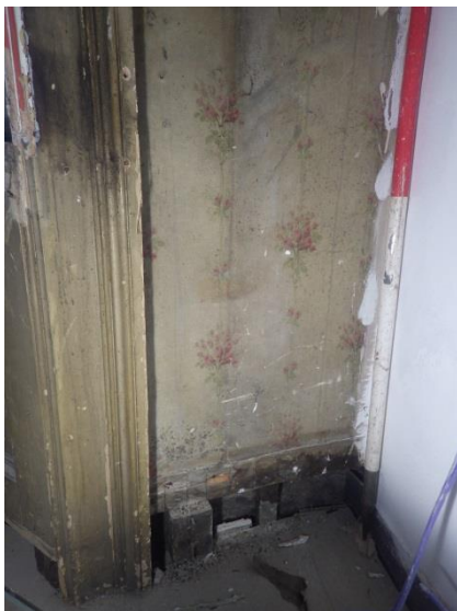
Plate 90 Room 3.4, detail of wall treatment.
