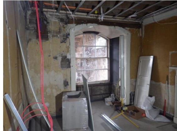
Plate 25 Lower ground floor, Room LG., north end.
