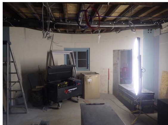
Plate 16 Basement, Room B.1, south end.
