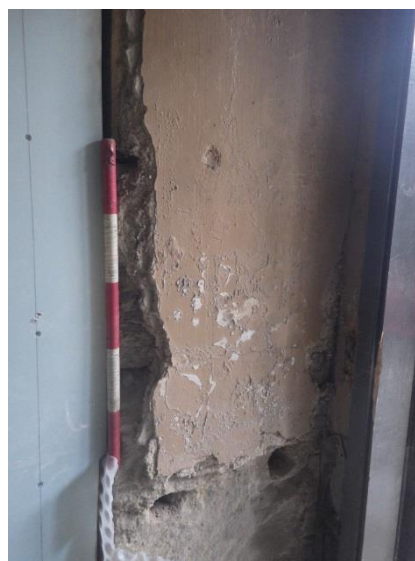
Plate 12 Basement, rear entrance jamb, wall treatment.
