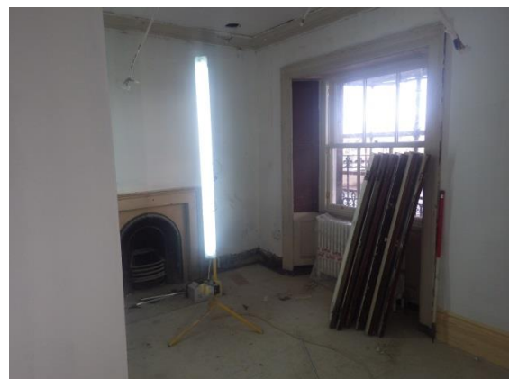
Plate 87 Room 3.4, general view. Facing NW.
