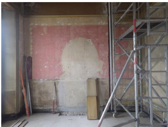
Plate 67 Room 1.1, former Boudoir, with Phase 1 removed fireplace. Facing W.
