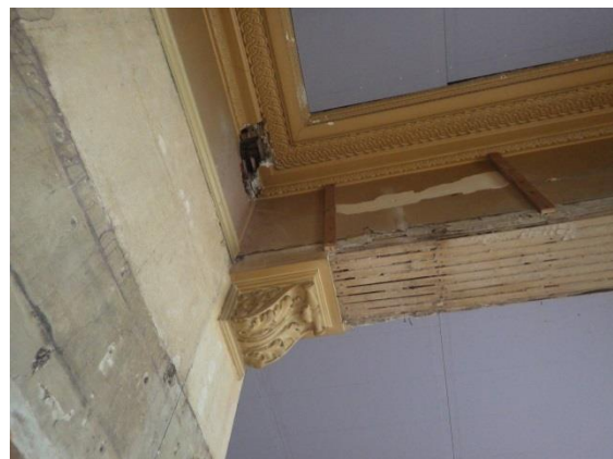
Plate 68 Room 1.1, Phase 2 beam soffit brackets at widened access into former Boudoir.
