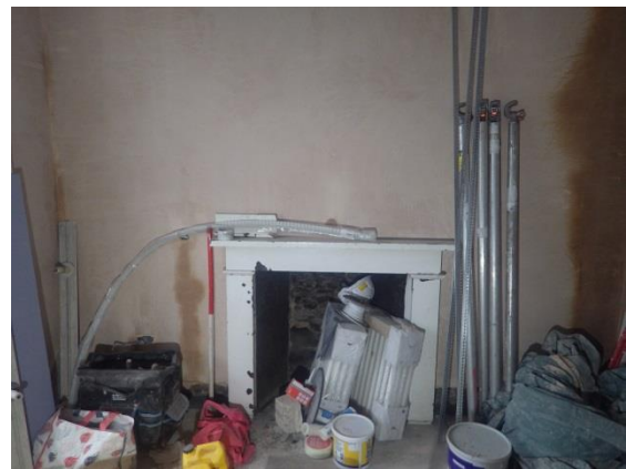
Plate 79 Room 2.4, fireplace. Facing W.
