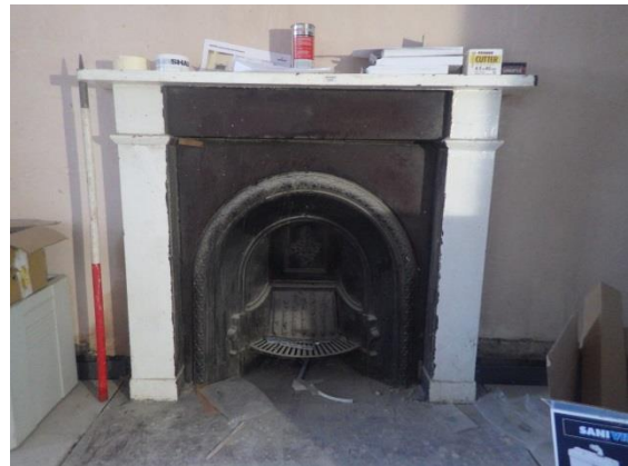
Plate 75 Room 2.2, detail of fireplace.
