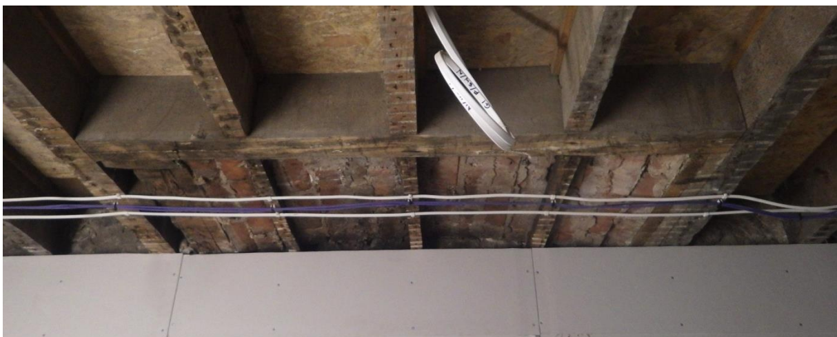
Plate 23 Basement, Room B.2, detail of brick hearth-setting for lower ground floor.
