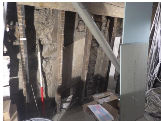
Plate 29 Lower ground floor, Room LG2 detail of spiral stair remnant.
