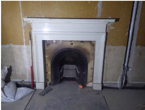
Plate 26 Lower ground floor, Room LG.1 fireplace.
