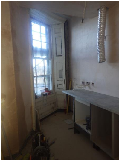
Plate 74 Room 2.2 west window. Facing NE.
