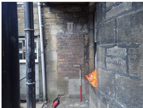
Plate 7 Northern offshoot, basement, Phase 1 blocked door Facing west.
