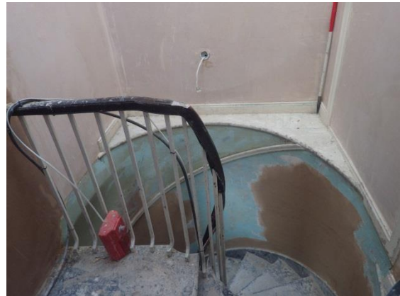
Plate 91 Room 3.5, back stair. Facing E.
