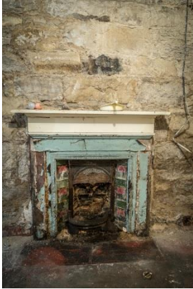
Plate 19 Basement, Room B.3, fireplace. Cooper Cromar
