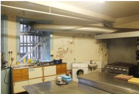
Plate 15 Basement, Room B.1 pre-strip view. Cooper Cromar.
