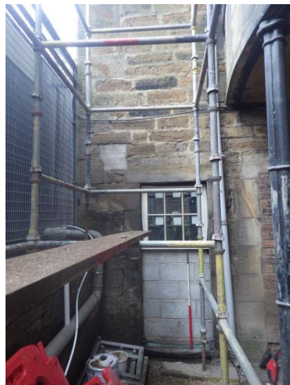
Plate 8 Northern offshoot, basement, Phase 1 blocked door Facing west..
