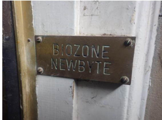
Plate 4 South elevation, external ground floor: Biozone/Newbyte nameplates.
