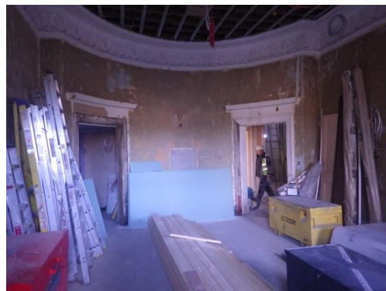
Plate 53 Room G.2, general view south end.
