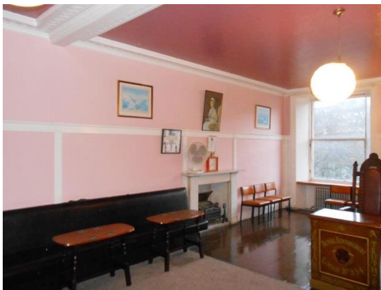
Plate 78 Room 2.3 general view pre-strip. Facing NE. Cooper Cromar
