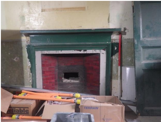
Plate 32 Lower ground floor, Room LG2 fireplace, south.
