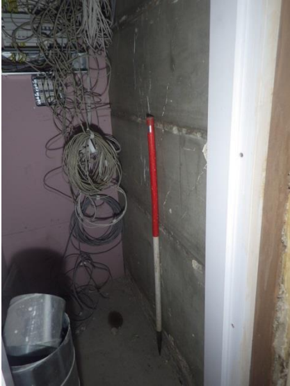
Plate 80 Room 2.5 with Phase 1 wall surface treatment
