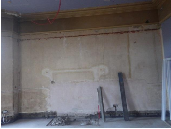
Plate 69 Room 1.2, former N Drawing Room, Phase 1 removed fireplace. Facing E.
