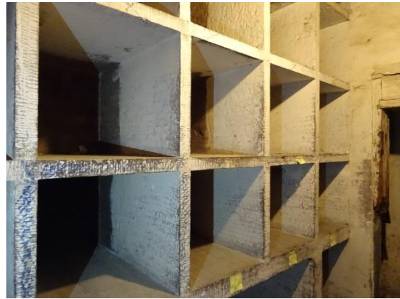
Plate 22 Basement, Room B.4, wine bins. S&B.
