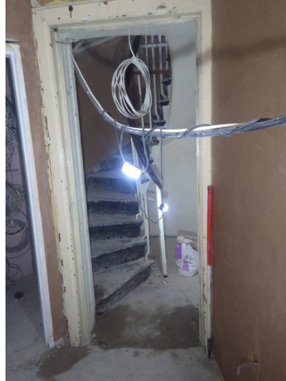
Plate 81 Second floor back spiral stair. Facing E.
