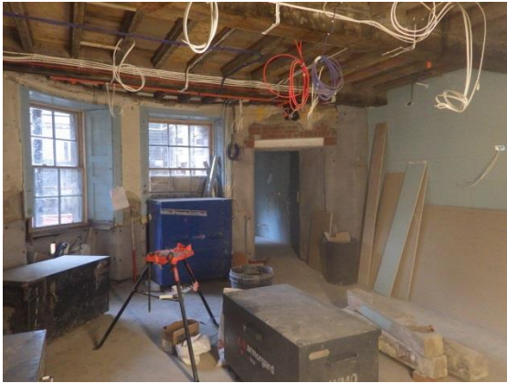
Plate 13 Basement, Room B.1 general view. Facing NE .
