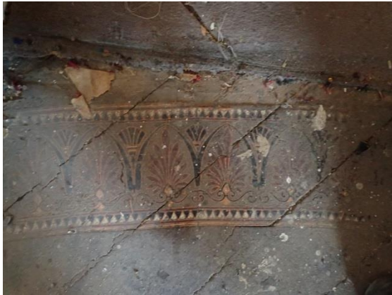
Plate 58 Room G.2, floor treatment. S&B
