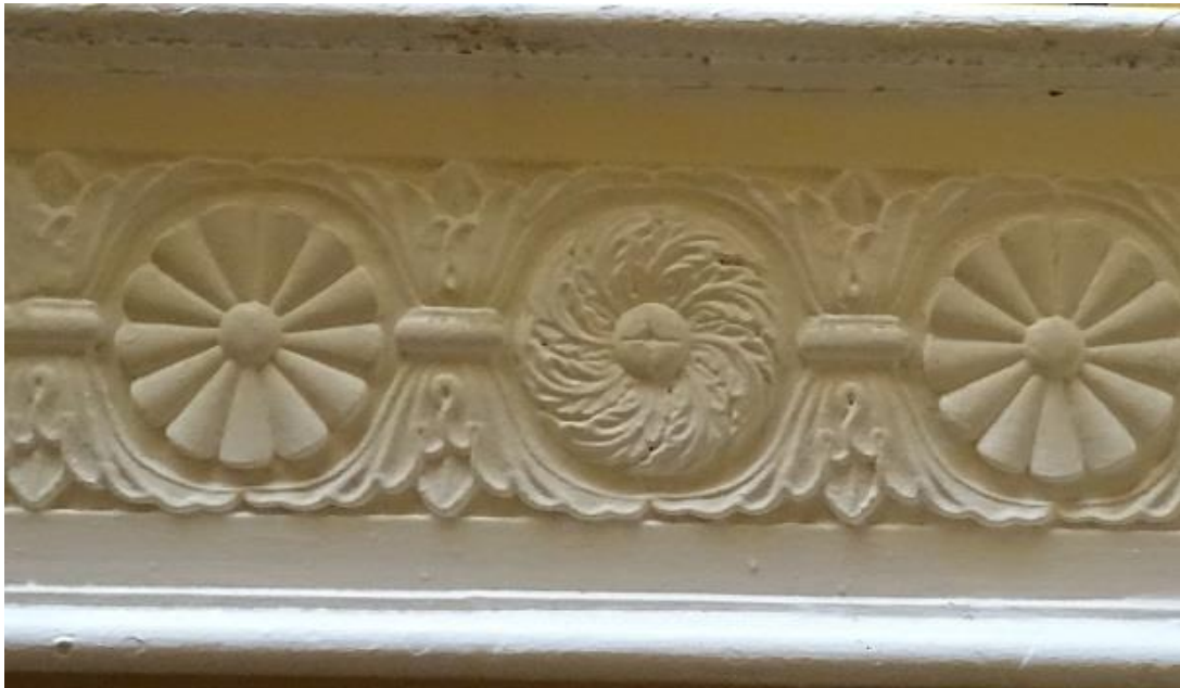
Plate 64 Main stair, plaster decoration on side of main beam of the stair landings. S&B
