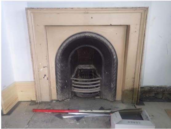
Plate 88 Room 3.4, fireplace. Facing W.
