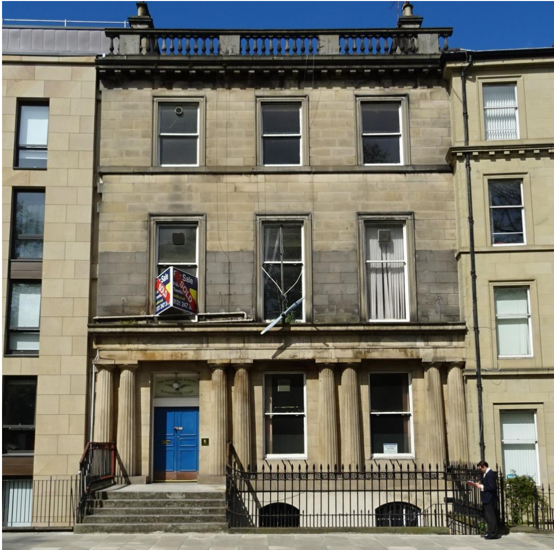
Plate 1 Main (south) elevation
