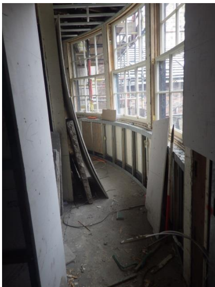
Plate 34 Lower ground floor, bowed passageway
