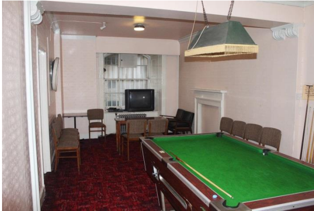
Plate 24 Lower ground floor, Room LG.1 pre-strip Cooper Cromar.
