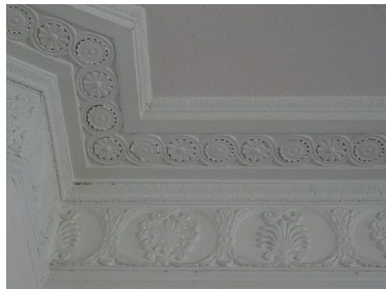
Plate 55 Room G.2, frieze and cornice detail. S&B.
