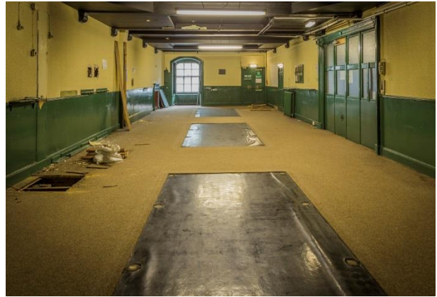
Plate 31 Lower ground floor, Room LG2 pre-strip Cooper Cromar.
