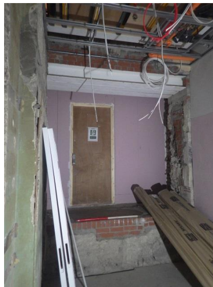
Plate 61 Room G.4, Phase 4 lift-shaft and new opening to west.
