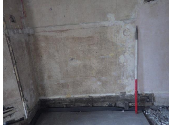
Plate 70 Room 1.2, detail of bell fitting at fireplace.
