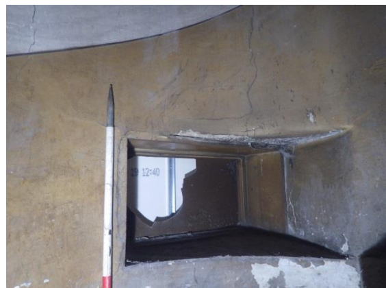
Plate 18 Basement, spiral stair window.
