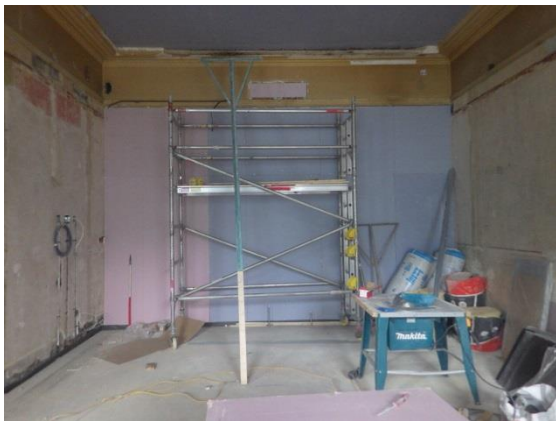
Plate 65 Room 1.1 with Phase 5 new partition and Phase 1 beams and cornicing. Facing N.
