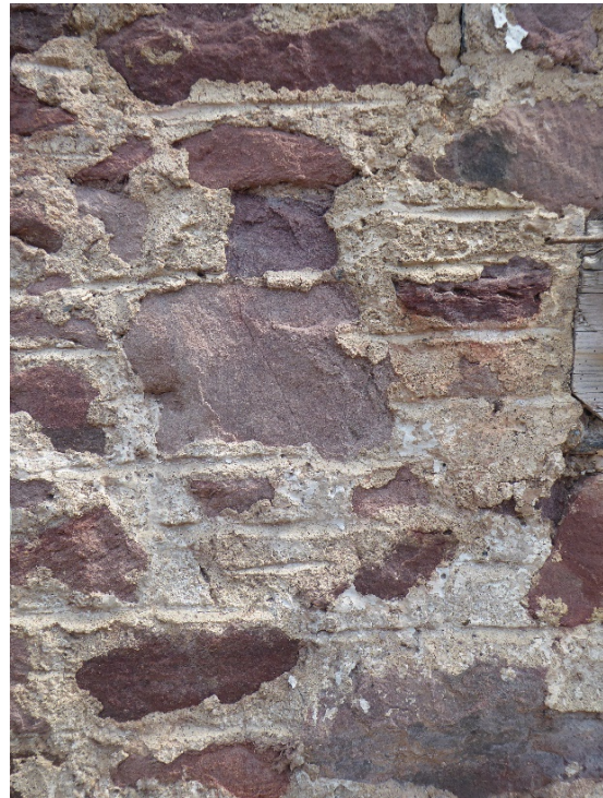
Plate 3 Pointing detail, W wall of machine house
