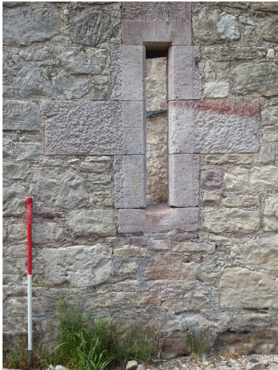
Plate 2 Tooling detail, vent opening on east wall of west range
