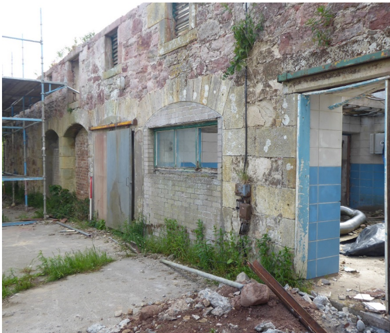
Plate 9 North elevation of cart shed
