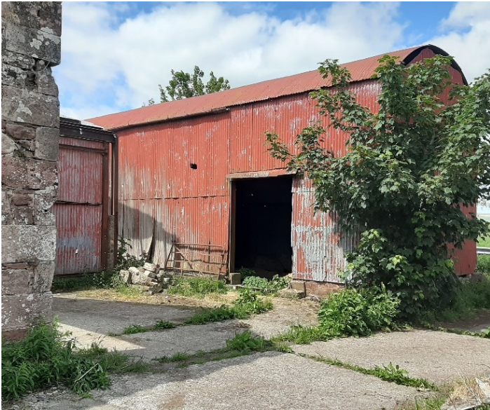
Plate 20 Exterior of Dutch Barn
