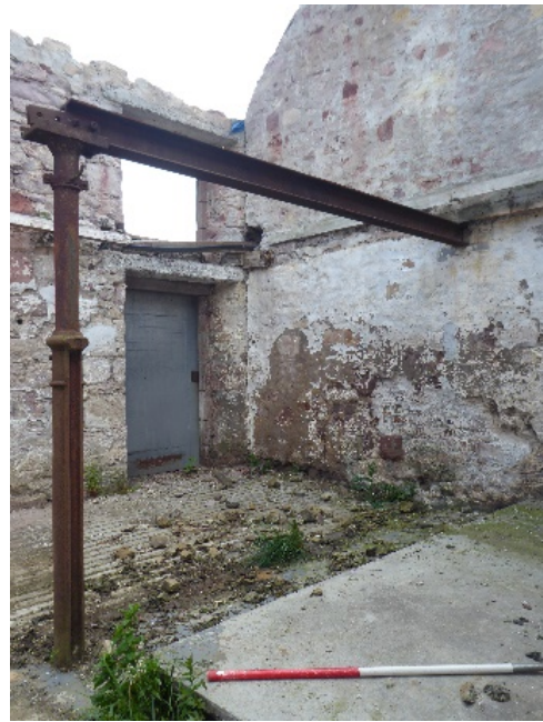
Plate 19 Pier and cast iron beam
