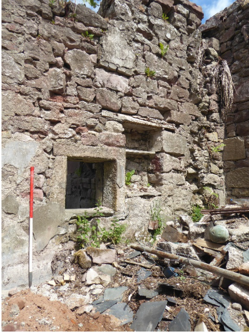
Plate 13 Wall recess in machine house
