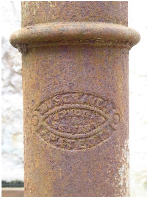
Plate 18 Cast iron pier detail
