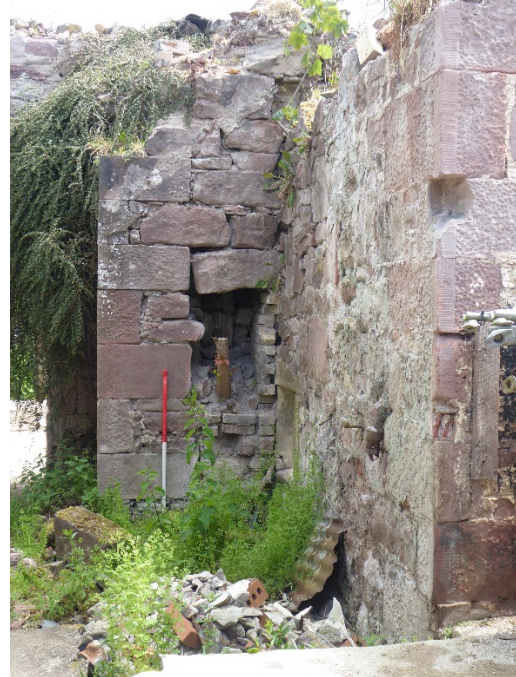
Plate 14 Stoke hole in base of chimney, looking east
