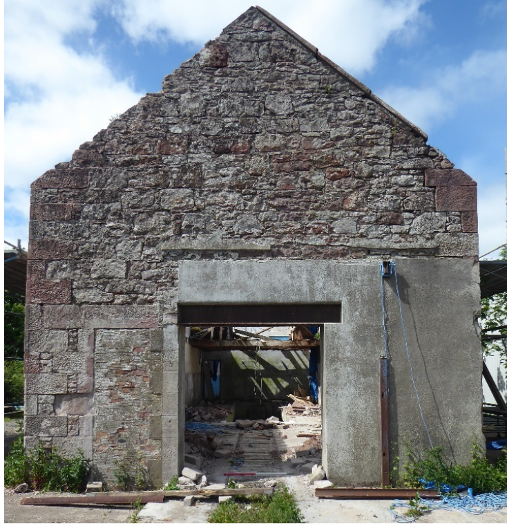
Plate 8 East gable showing former entrance to stable to left
