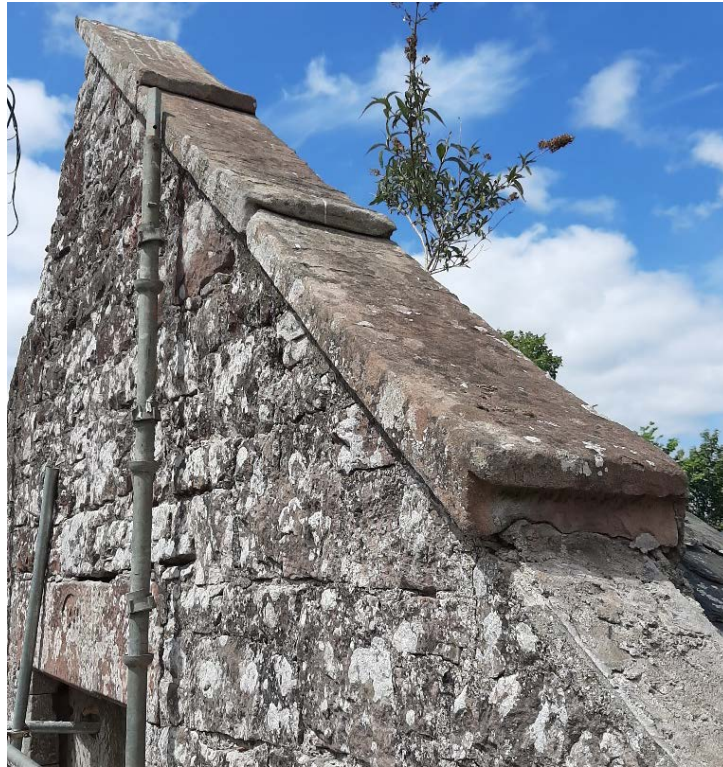
Plate 6 Detail of coping
