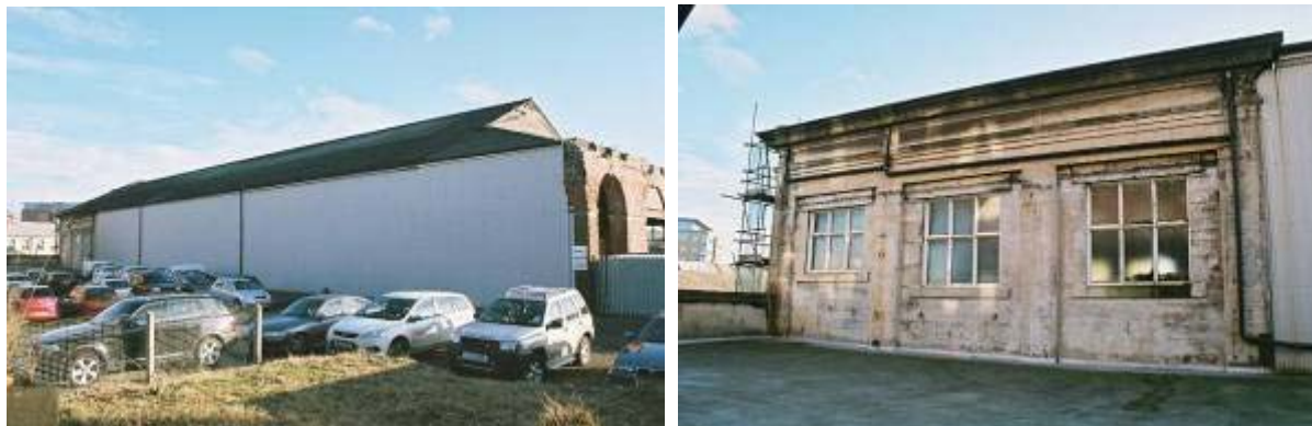
Plate 57: N elevation of Goods Warehouse, general view looking SE, showing later covering Plate 58: N elevation of Goods Warehouse, original masonry at E end
