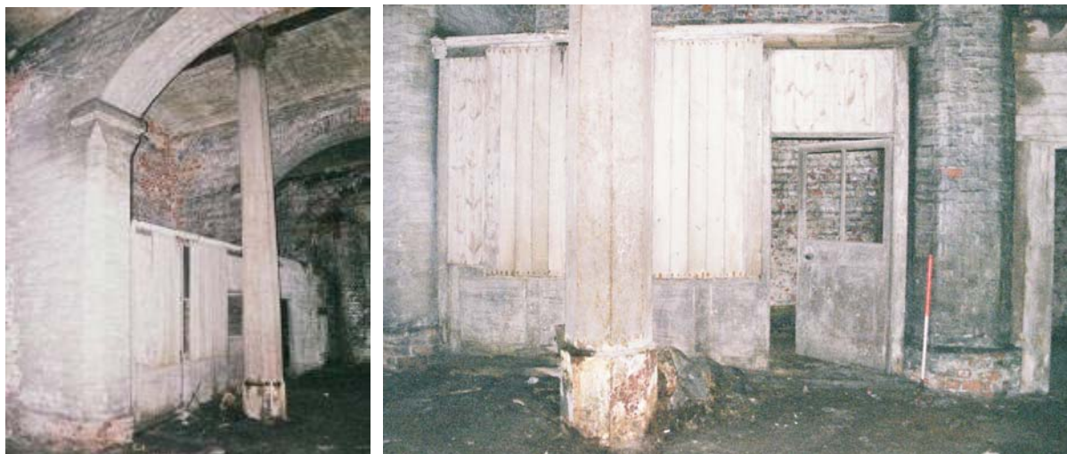
Plate 19: Partitions at northern end of aisle 2 and 3, view looking NE
