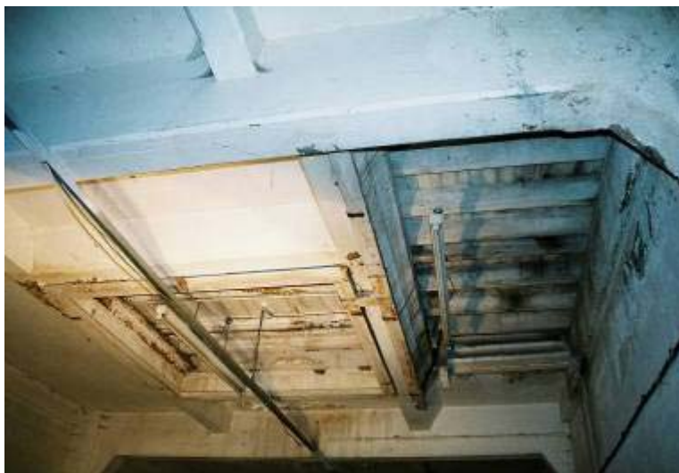
Plate 76: Link Building first floor, room 9, boarded over hole in floor indicating former location of stairs leading up from the ground floor
