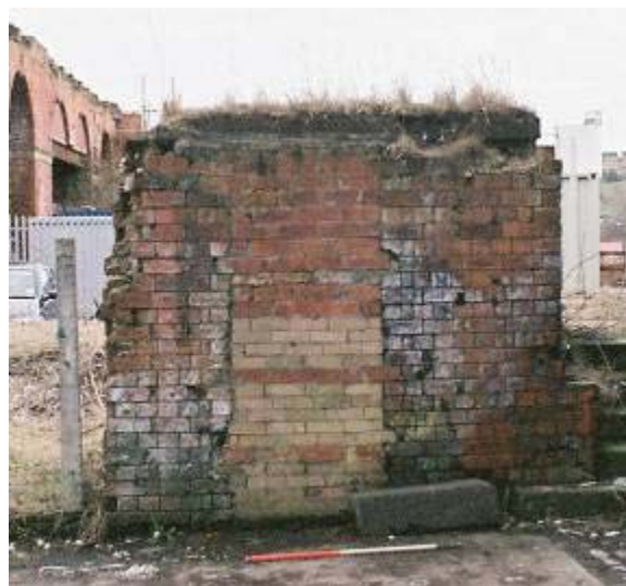
Plate 13: Brick structure in car park area, formerly providing access to the viewing platform in the station undercroft below (bay 9, aisle 2)
