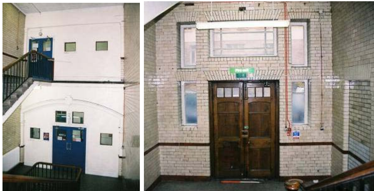
Plate 26: W elevation in principal stairwell, to second and third floors
