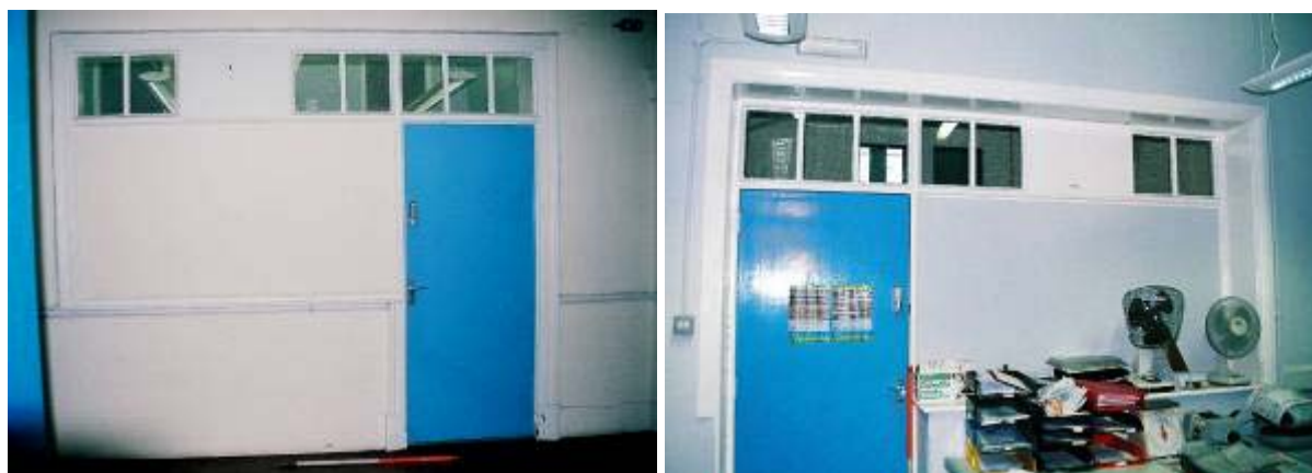
Plate 42: blocked Messenger office window, view looking from corridor into room 5, first floor
