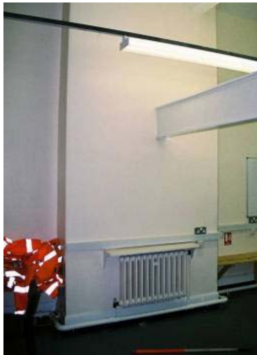
Plate 34: wall scar and cut in window sill and skirting, showing former counter location for Receiving Office, now in room 7
