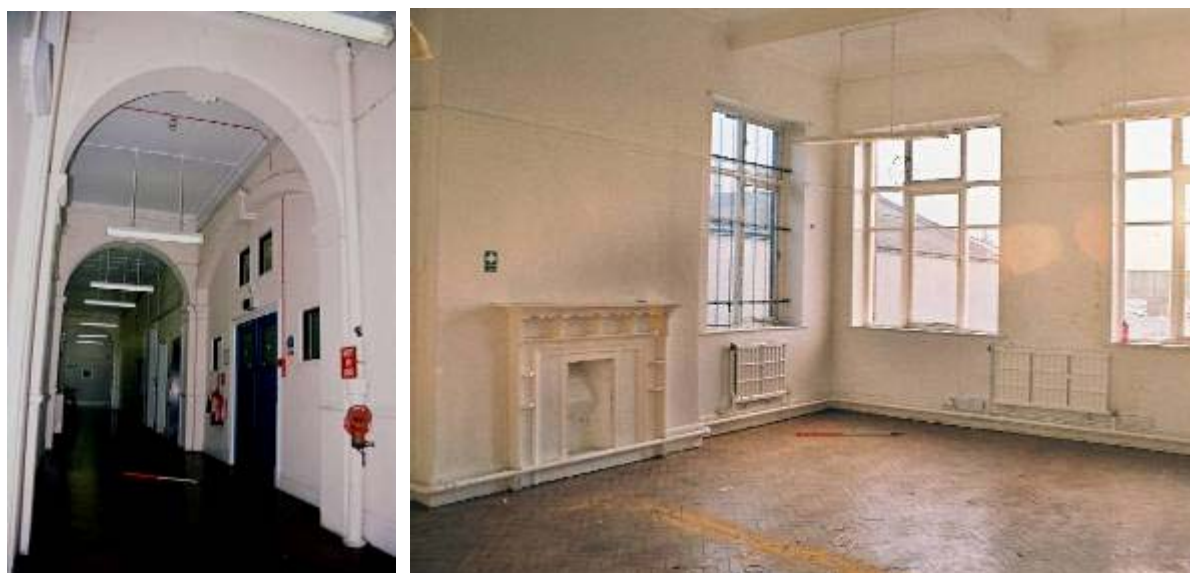
Plate 40: Detail of arches in corridor at entrance from stairwell, view looking N Plate 41: Room 2, first floor, view looking SW, with original fireplace in S wall
