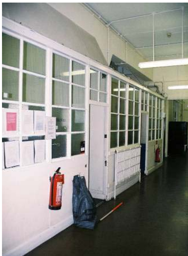
Plate 32: secondary half glazed partitions forming W wall of former Enquiries Office, view from NW corner of corridor 2
