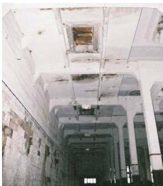
Plate 60: 'Hyatt's lights' in ceiling of warehouse, ground floor, above the N rulleway
