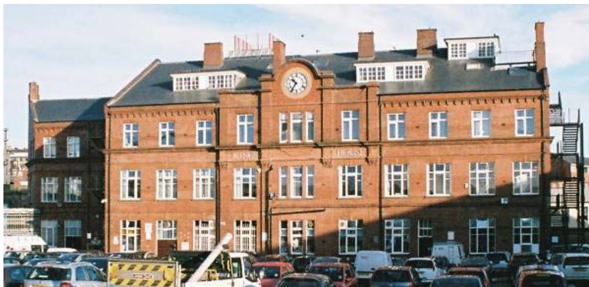
Plate 23: W elevation of Kings House
