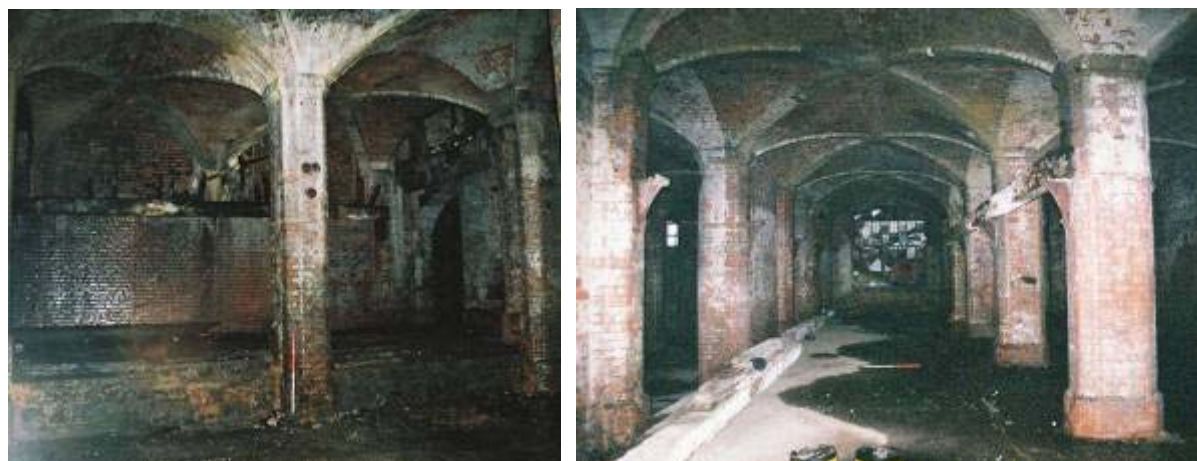
Plate 9: raised area to the west of 'aisle 4' in the Goods Station undercroft, looking west
