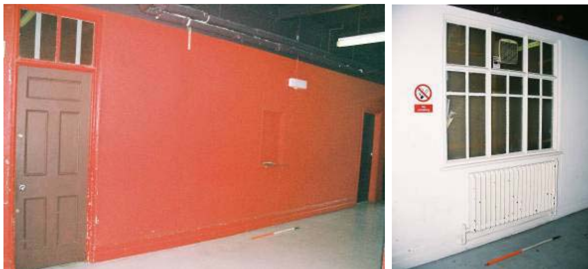
Plate 28: lower ground floor corridor 2, doorway to library, with blocked librarians hatch in the centre of the image, with later insertion doorway to room 13 towards the right of the image
