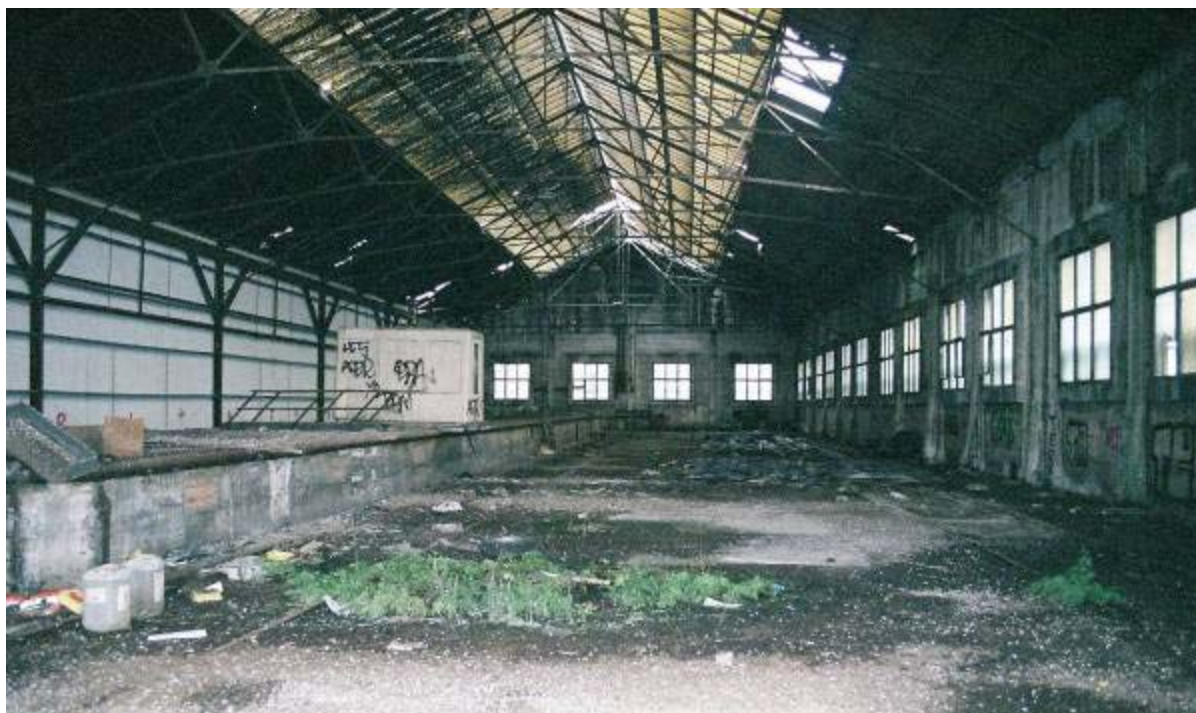
Plate 62: general view of upper floor of warehouse, looking E
