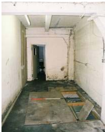
Plate 76: Link Building first floor, room 9, boarded over hole in floor indicating former location of stairs leading up from the ground floor
