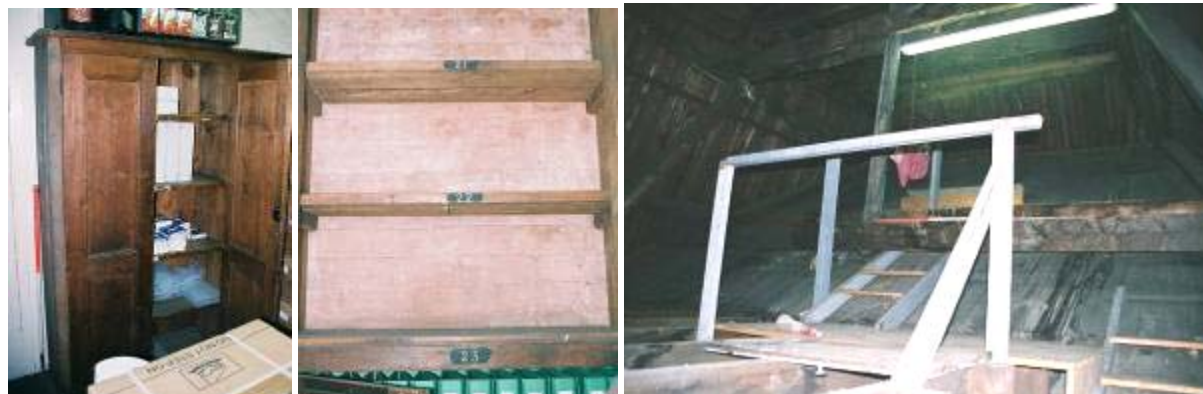
Plate 52: cupboards in room 13.1
