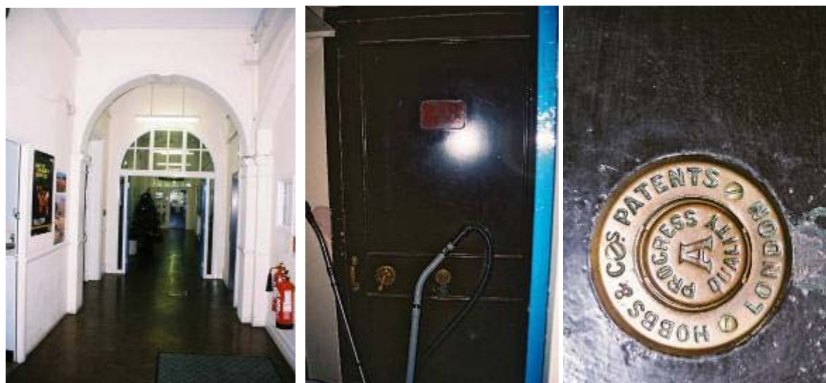
Plate 44: General view down corridor on second floor, looking N
