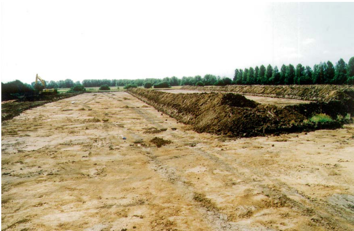
Plate 2. Processing area, general site shot, looking south.
