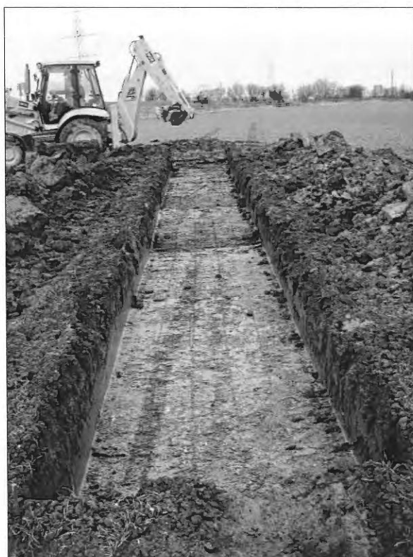
Plate 6. Trench 4 showing Ditches 121 and 127, and field drain, looking north-west, pre-excavation
