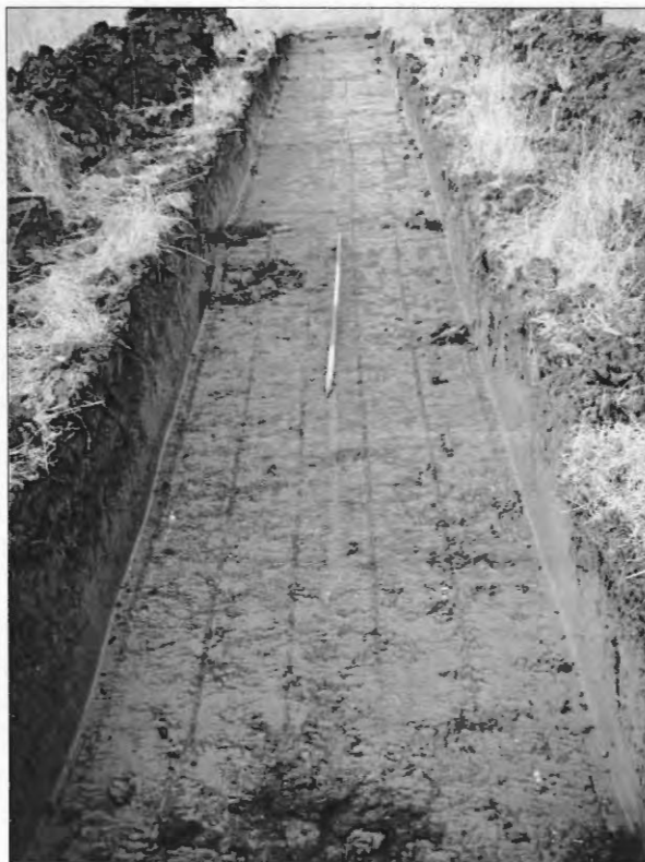
Plate 3. Trench 2 showing field drain filled with industrial waste material, looking south-east
