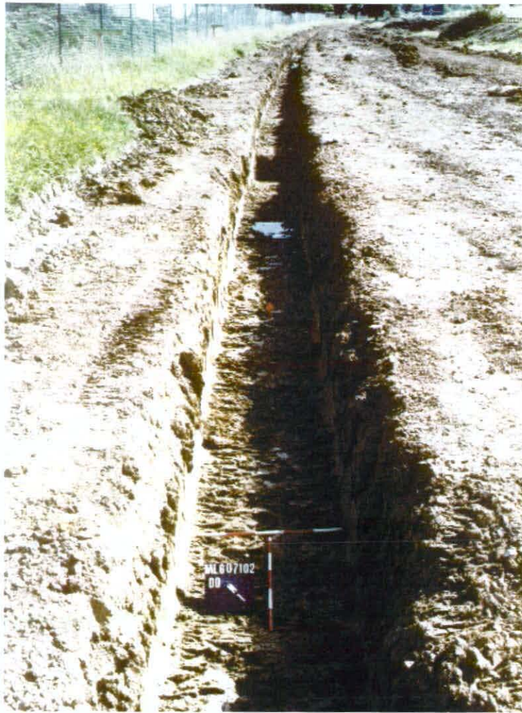
Plate 1. General shot of drainage trench, looking north-west.
