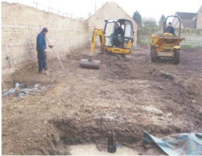
Plate 12 – Machine excavation during work
