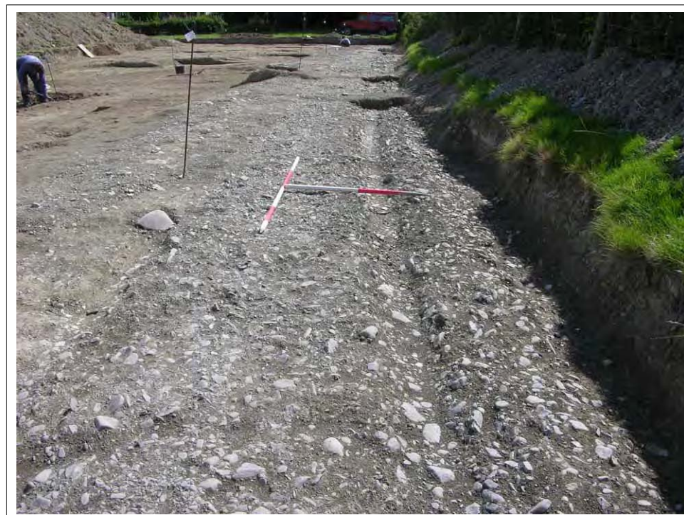
Plate 20: View along road surface, Looking SE, Scales 1x1m & 1x2m
