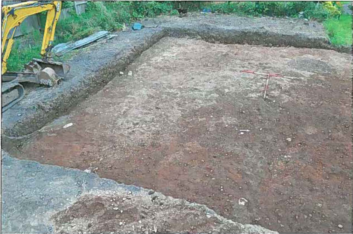
Figure 11. Structure 102/105/112 prior to excavation
