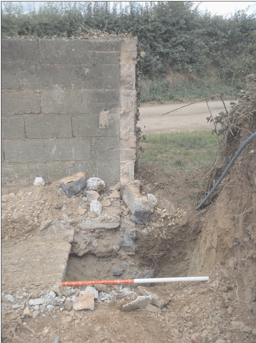
Plate 1: Test Pit 1, view to the south (Scale 1m)
