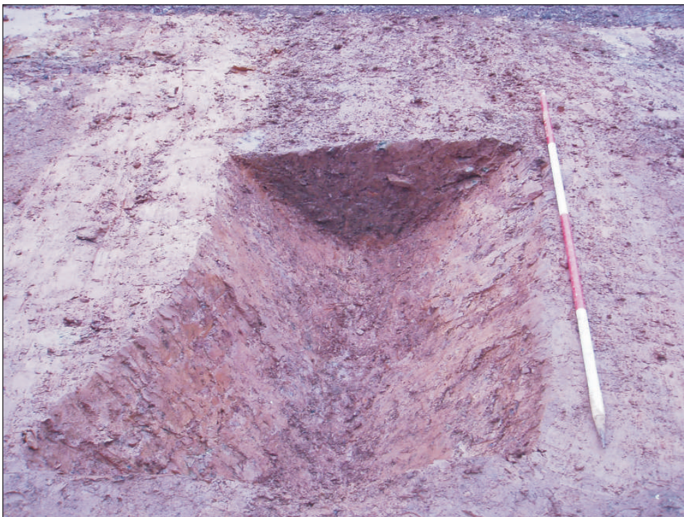
Plate 12: The Car Park, section through mausoleum F3108, viewed from the west. 2m scale.
