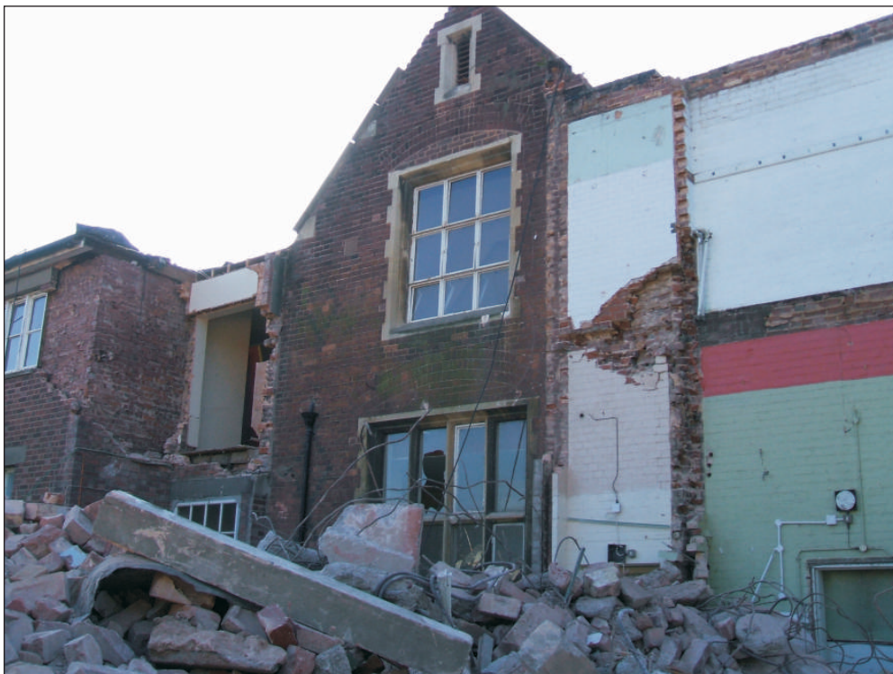
Plate 2: The north elevation of the Episcopal School during demolition showing the central inserted 1936-8 windows, viewed from the north.
