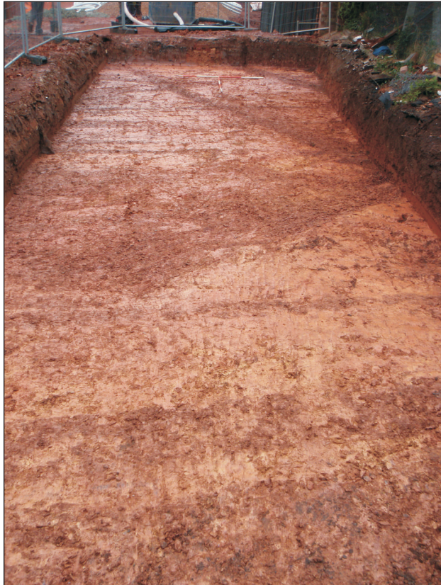
Plate 13: The Ramp, pre-excavation view showing Roman post-trenches (rear) and post-medieval gullies (foreground), viewed from the northeast. 2m scales.
