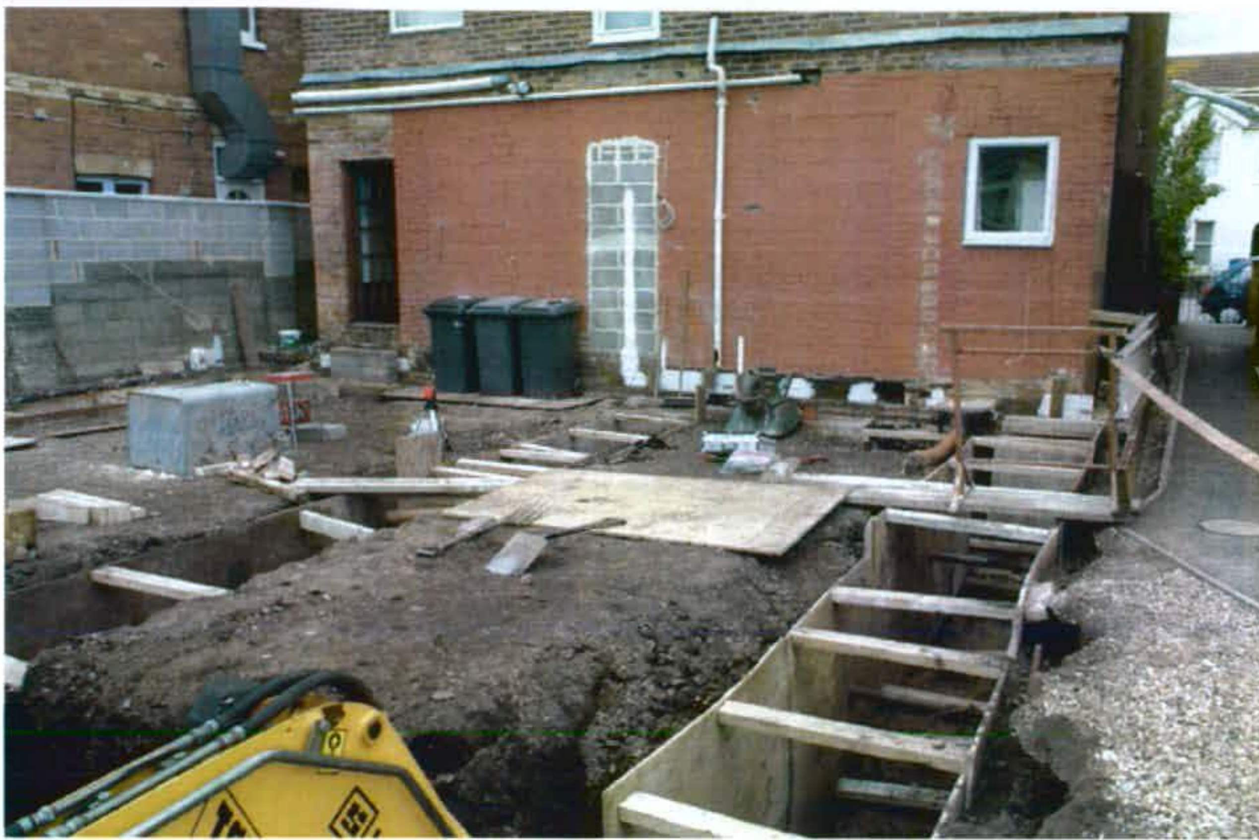
Plate 1: General view of site looking north.
