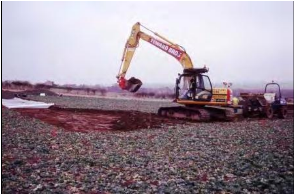
Plate 1 Stripping an access track and laying down protective membrane
