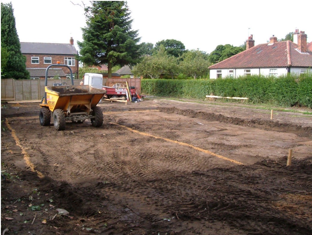
Plate 1. View of Site after Topsoil Strip. Facing South West
