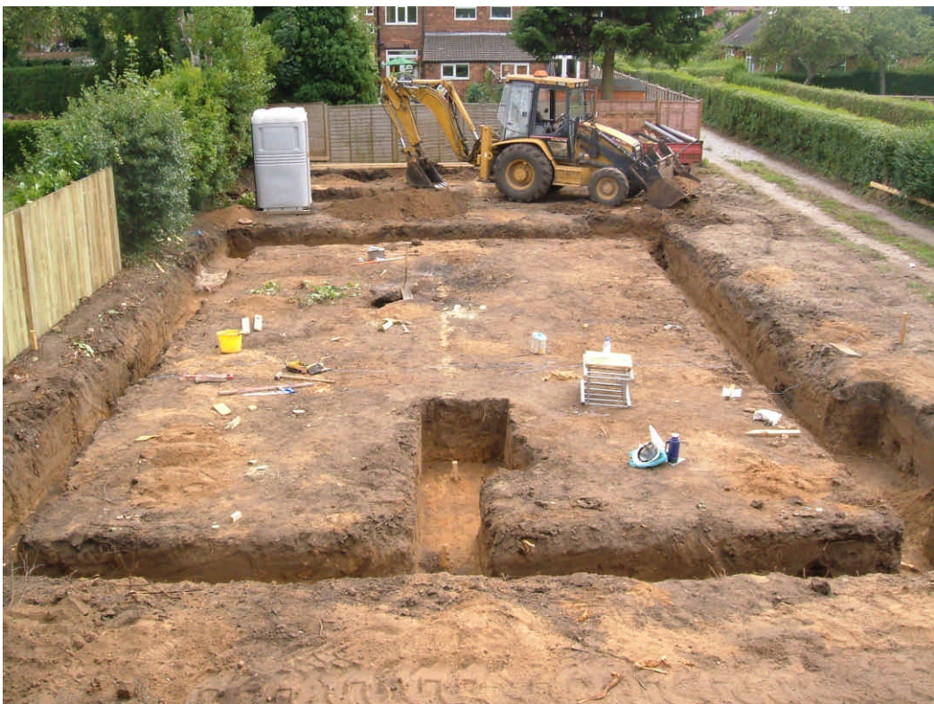
Plate 2. Overall View of Foundation Trenches. Facing South
