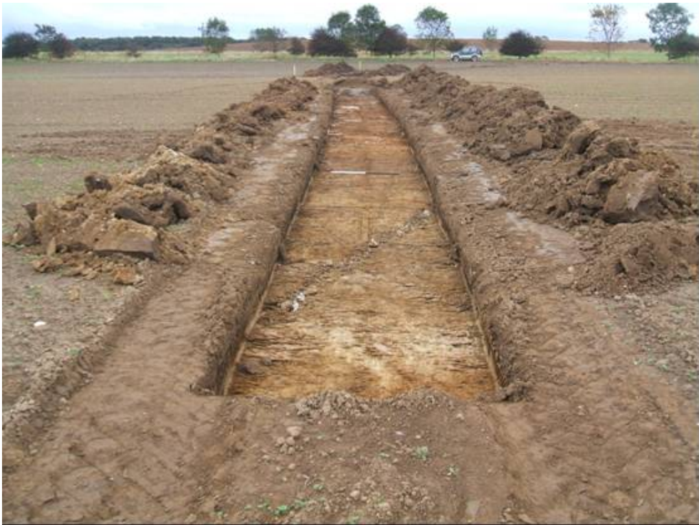
Plate 14 Trench 33, looking south, with stone-lined field drain [33002] in the foreground (1m scale)
