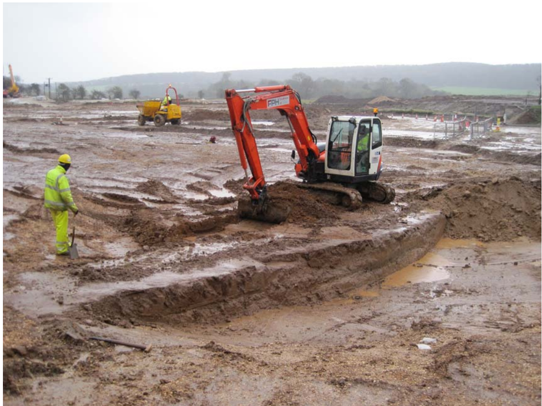
Plate 12: Area 1 – Excavating hollow 7740, looking south-east
