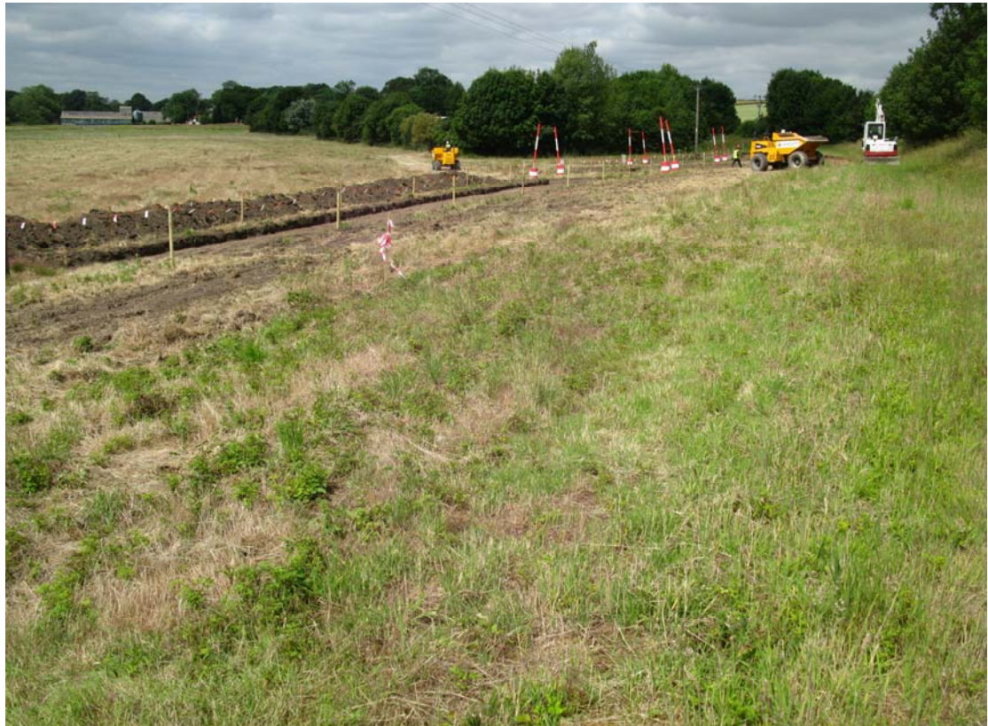
Plate 35: Area 1 – During the removal of topsoil, looking west
