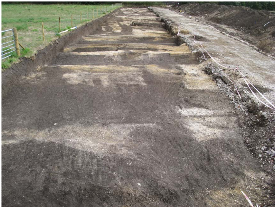
Plate 38: Area 2 – Southern end pre-excitation, looking north (1m scale)
