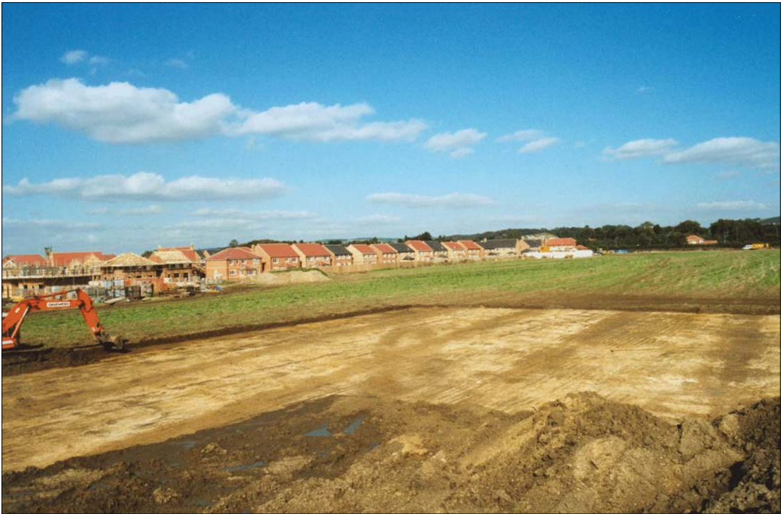
Plate 2: Topsoil stripping in Area C, looking north-east
