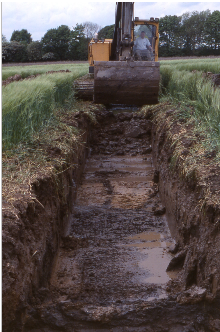
Plate 2 Excavation of Trench 3 exposing continuation of droveaway ditches from Trench 2
