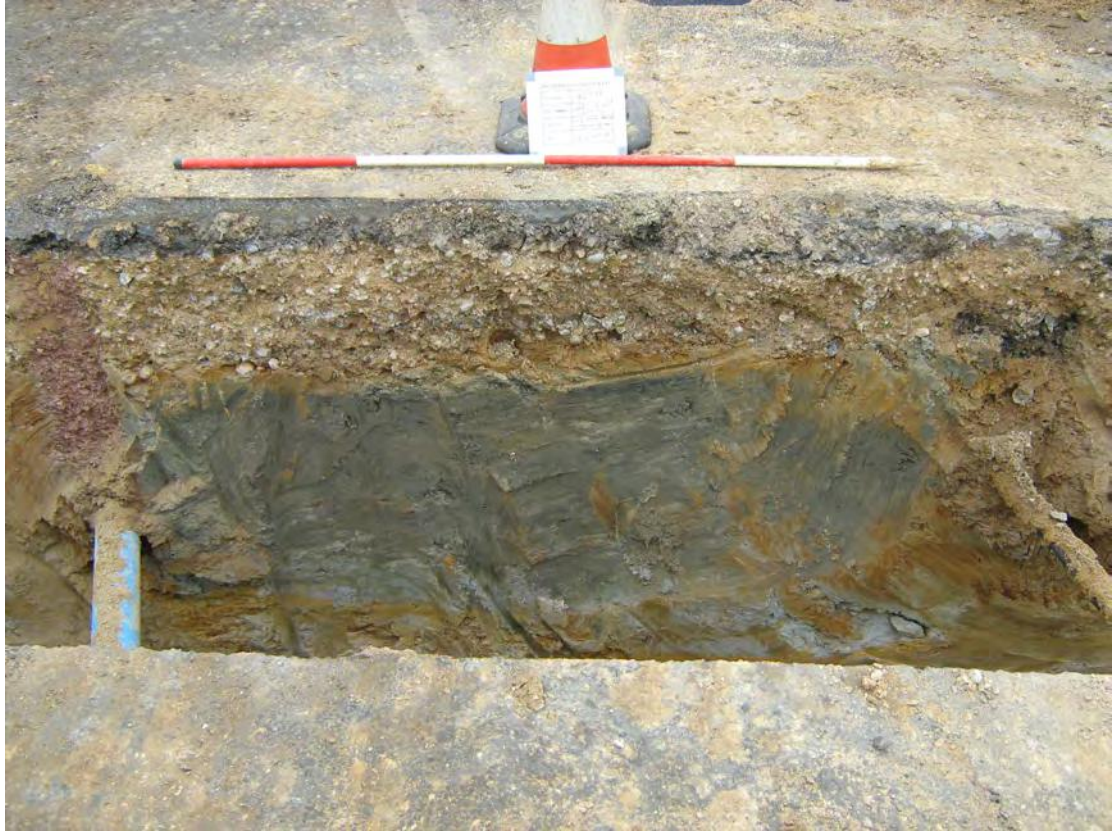
Fig. 17: Wartling Road crossing
