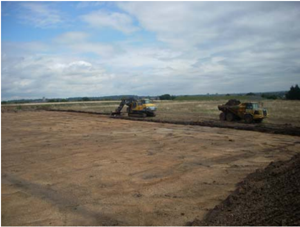
DP 1. Soil stripping. NE facing.
