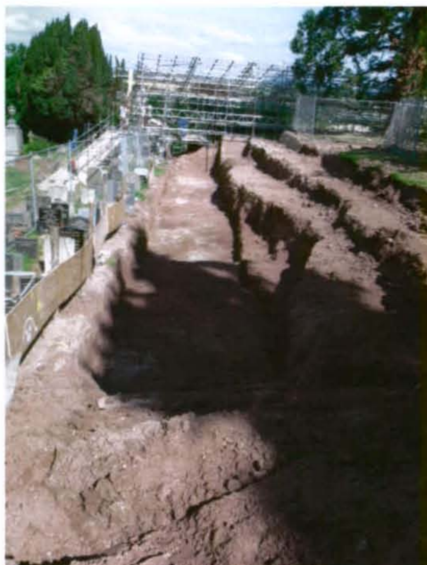
Plate 3: Overview of works on W side of structure
