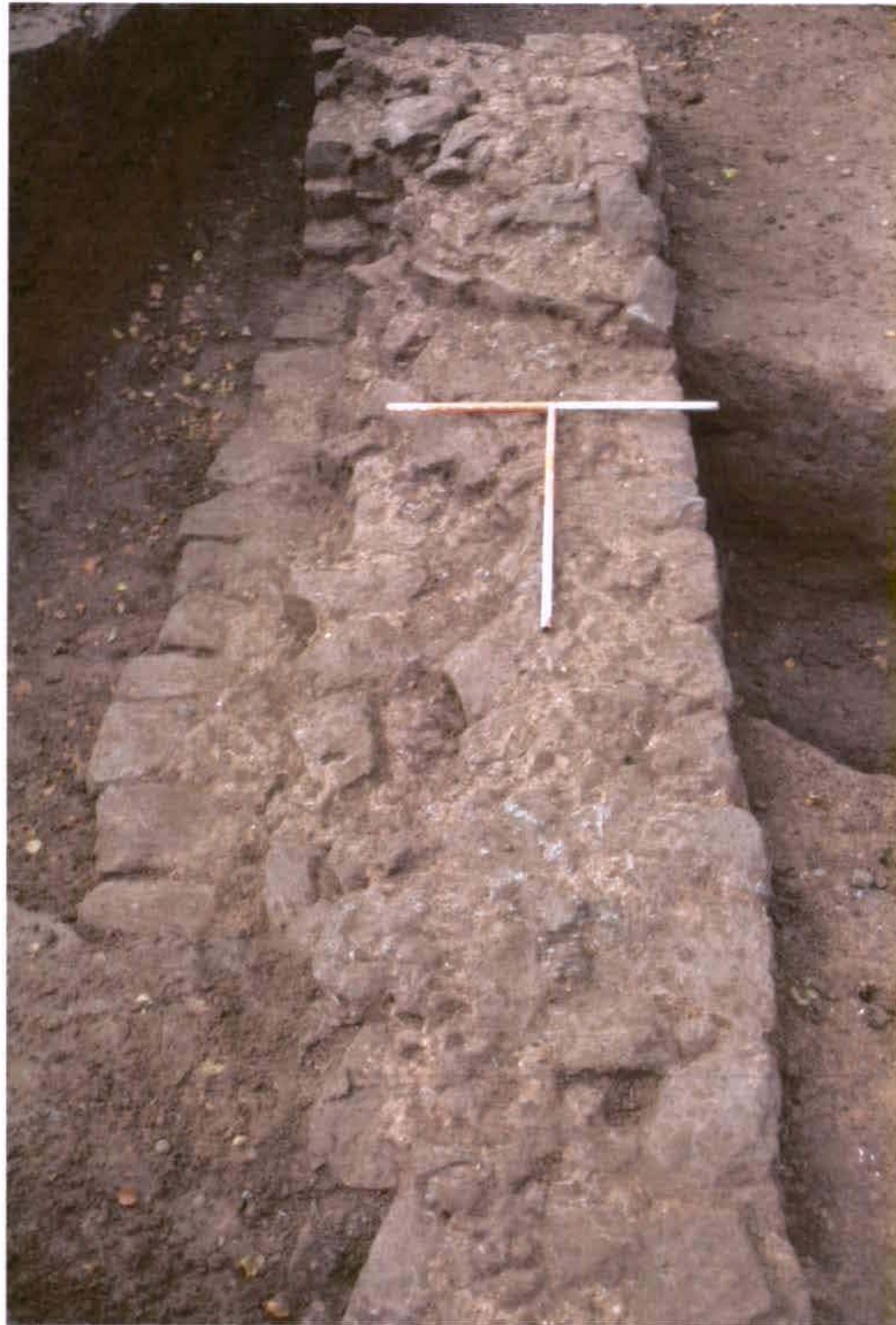
Plate 35: View NW of masonry wall (1006)
