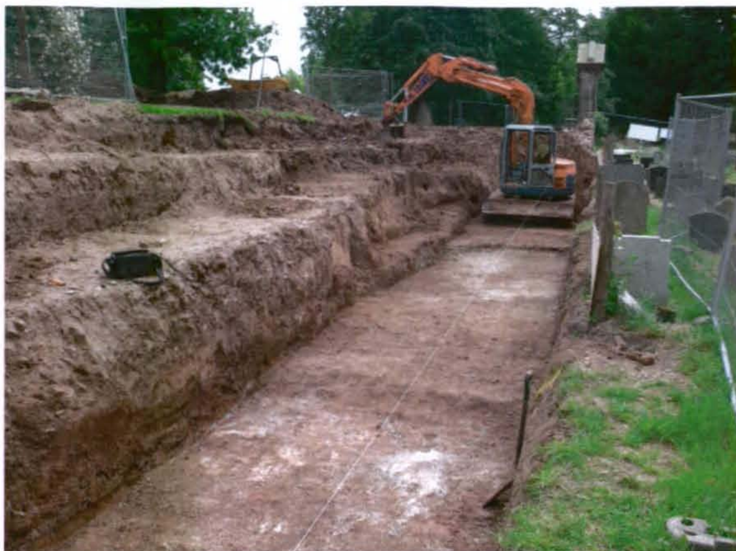
Plate 2: Excavations in progress during the Prospect watching brief
