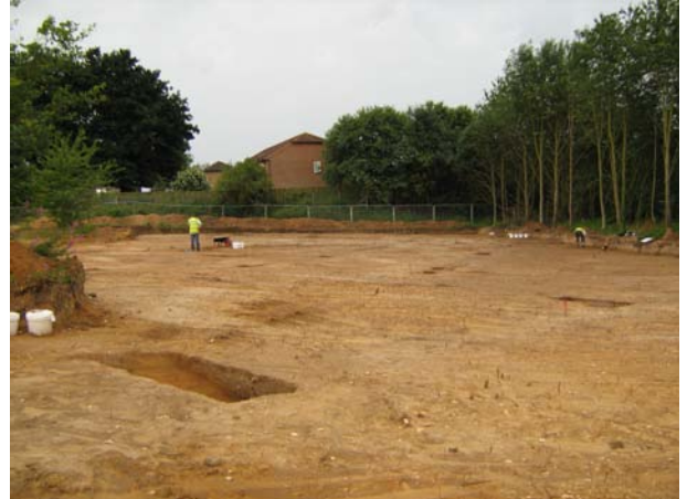
Plate 2: General site shot (facing south)
