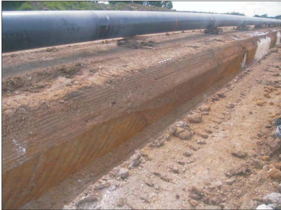
Plate 3: Palaeochannel [6455] following pipe trenching
