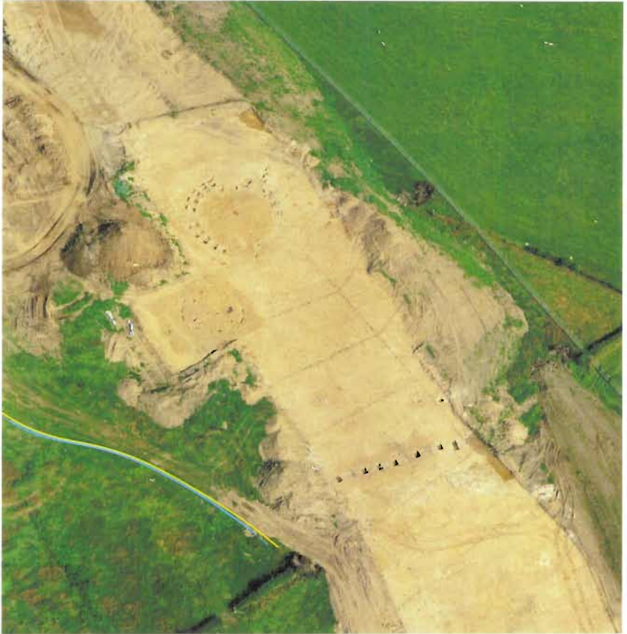
Plate 1: Aerial view of excavation area along the line of the proposed South West campus access road, with partially excavated boundary ditch 222 in the foreground and the roundhouse and enclosure in the east of the area
