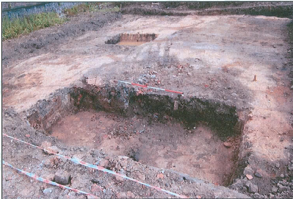
Figure 20 Sectioned demolition hole 014/015, probably location of former coal cellar. View to north east.
