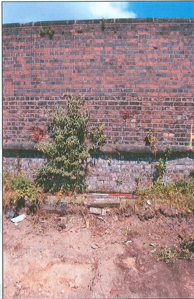
Figure 6 Brick boundary wall 017, delineating the northern boundary of the development site, note stone kerbstone at base of wall and absence of Copenhagen Road surface in foreground.
