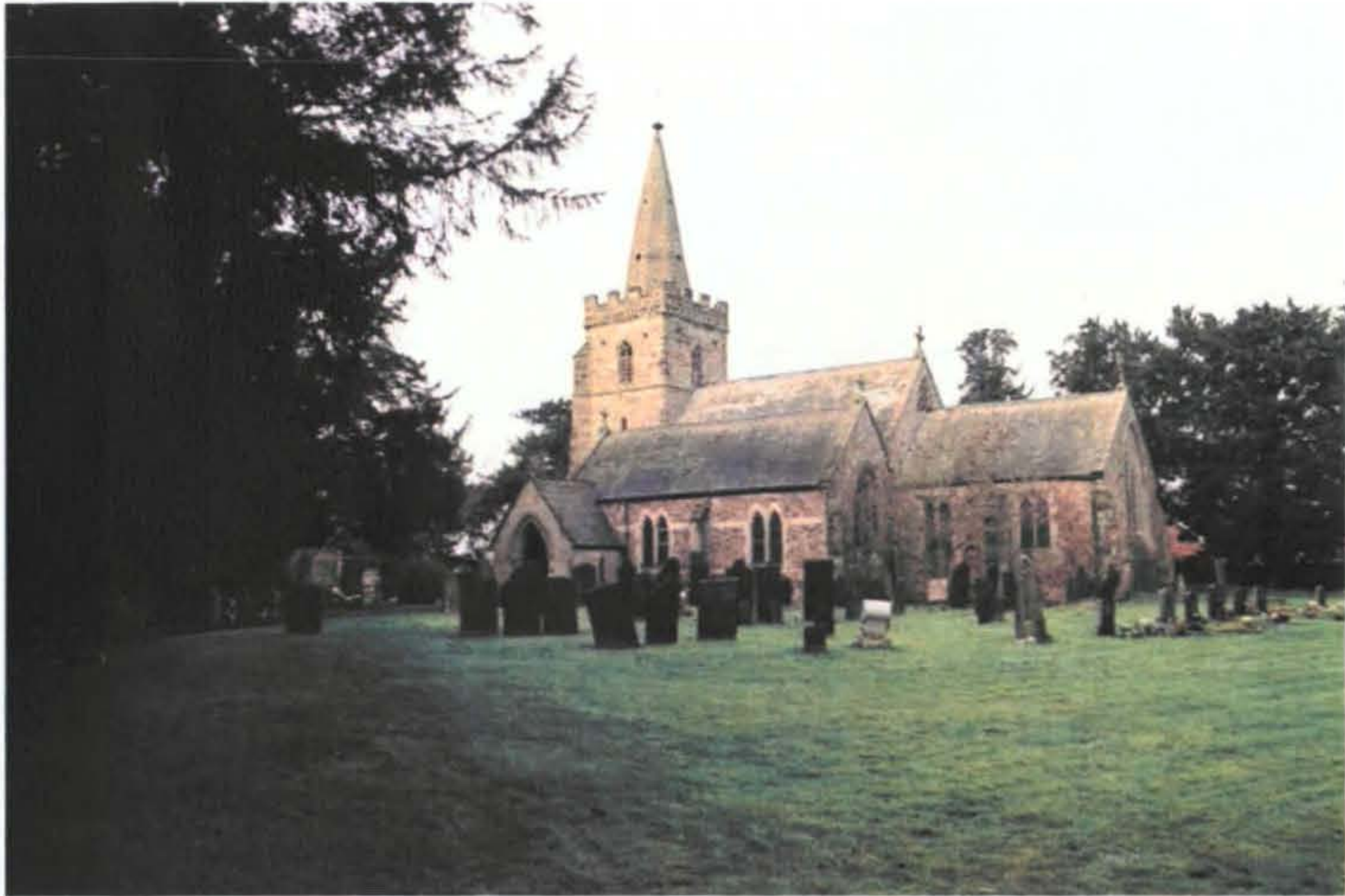
Plate 1 Northwest facing view across churchyard towards parish church
