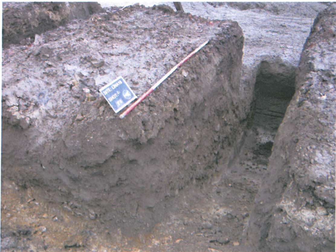
Plate 18. Block A watching brief. North edge of quarry pit [609], Section 28 looking south
