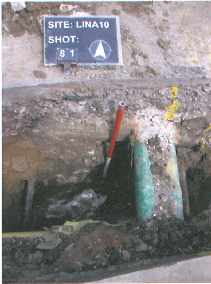
Plate 19. Watching brief on Newport service trench. Wall [627] looking north
