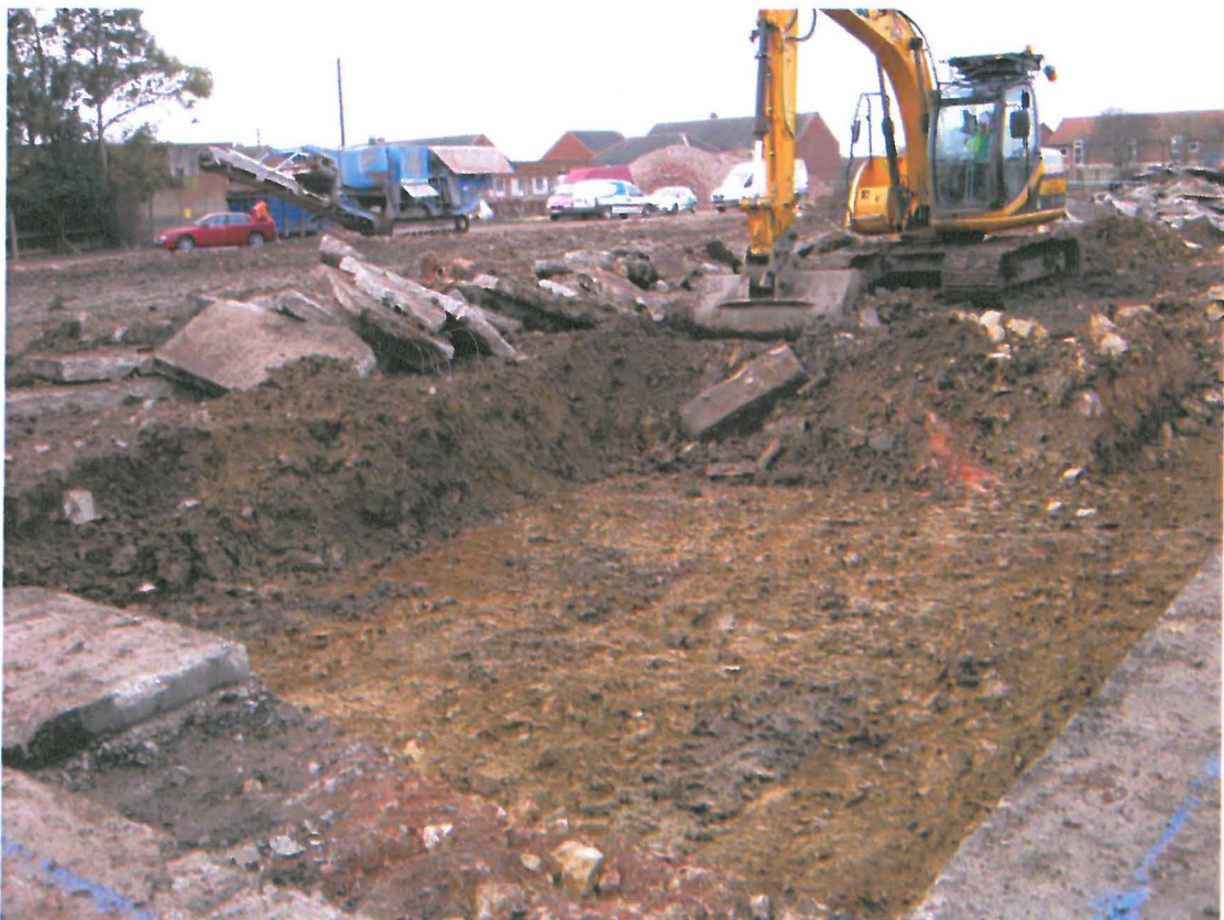
Plate 2. Machining east end of the site looking southwest
