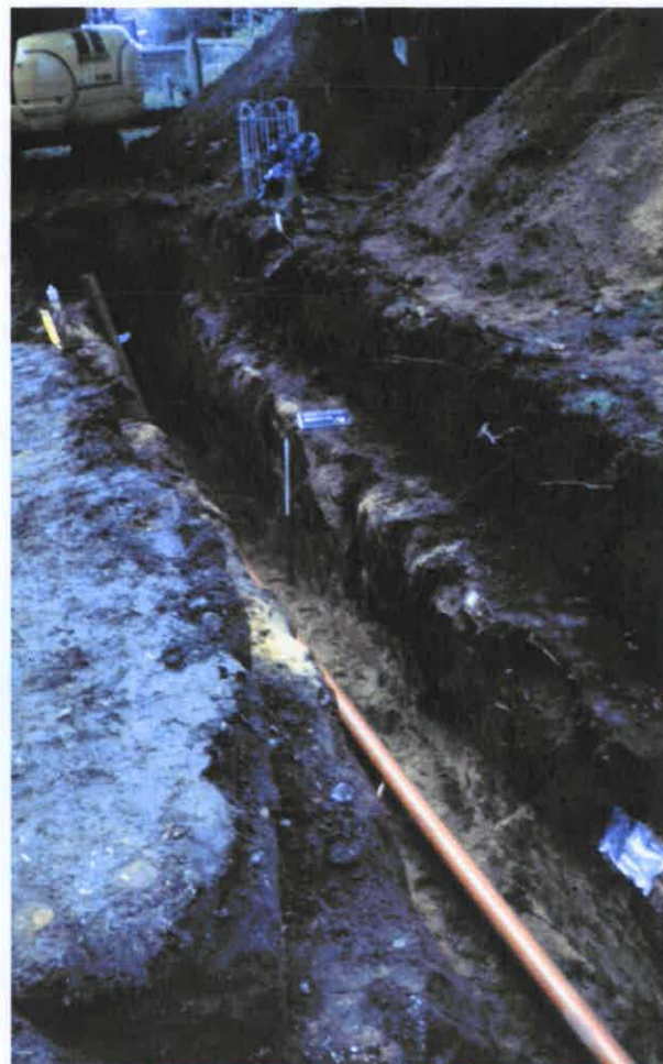
Plate 4 Service Trench at western end of church, looking south
