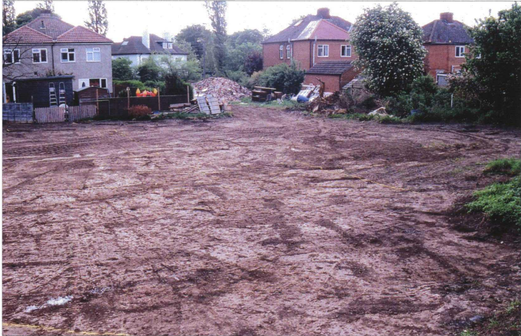
Plate 1 Leeming Lane, Catterick: view of site after soil stripping
