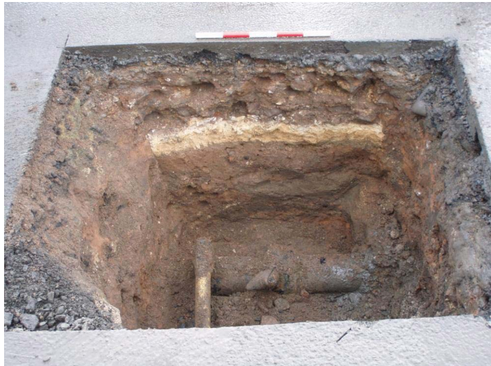
Plate 4 Metalled surface, predominantly of cobbles, below modern road materials in Trench 50. The pale coloured layer of crushed stone immediately below may relate to a bedding/makeup. Looking S
