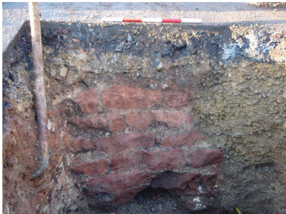
Plate 12 Wall of mortared red sandstone, 855, in Trench 85, looking W. Truncated to three sides by modern services the orientation of the blocks indicates the alignment of the wall.
