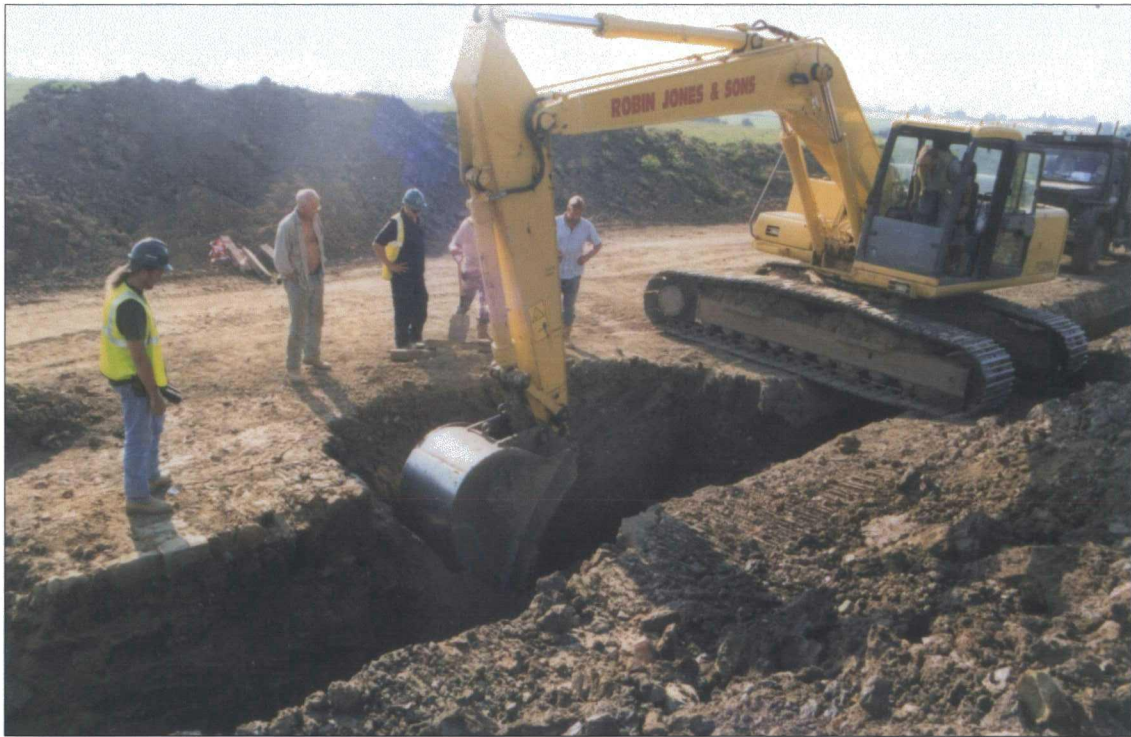
Plate 1 Monitoring of pipe trench
