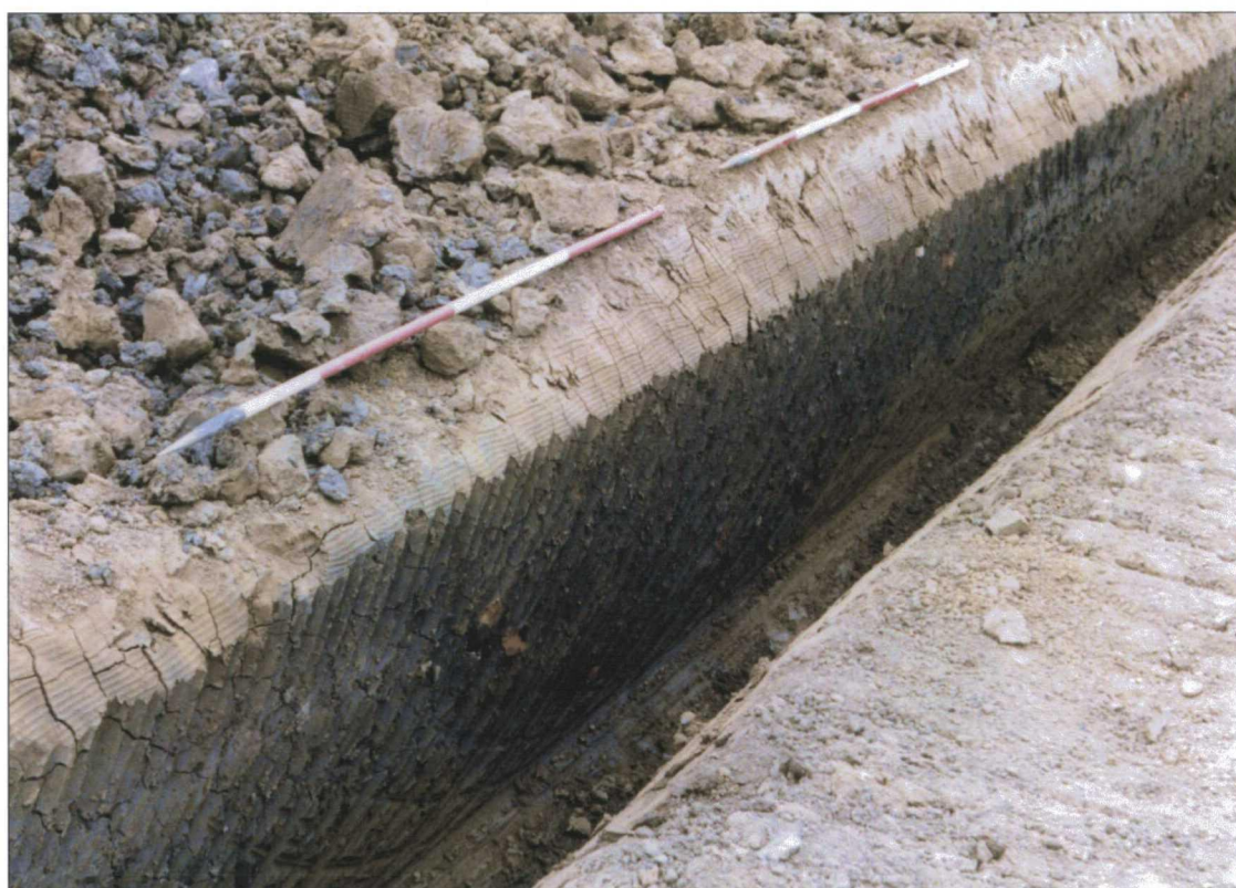
Plate 4 View along pipe trench showing feature 76, facing south-east
