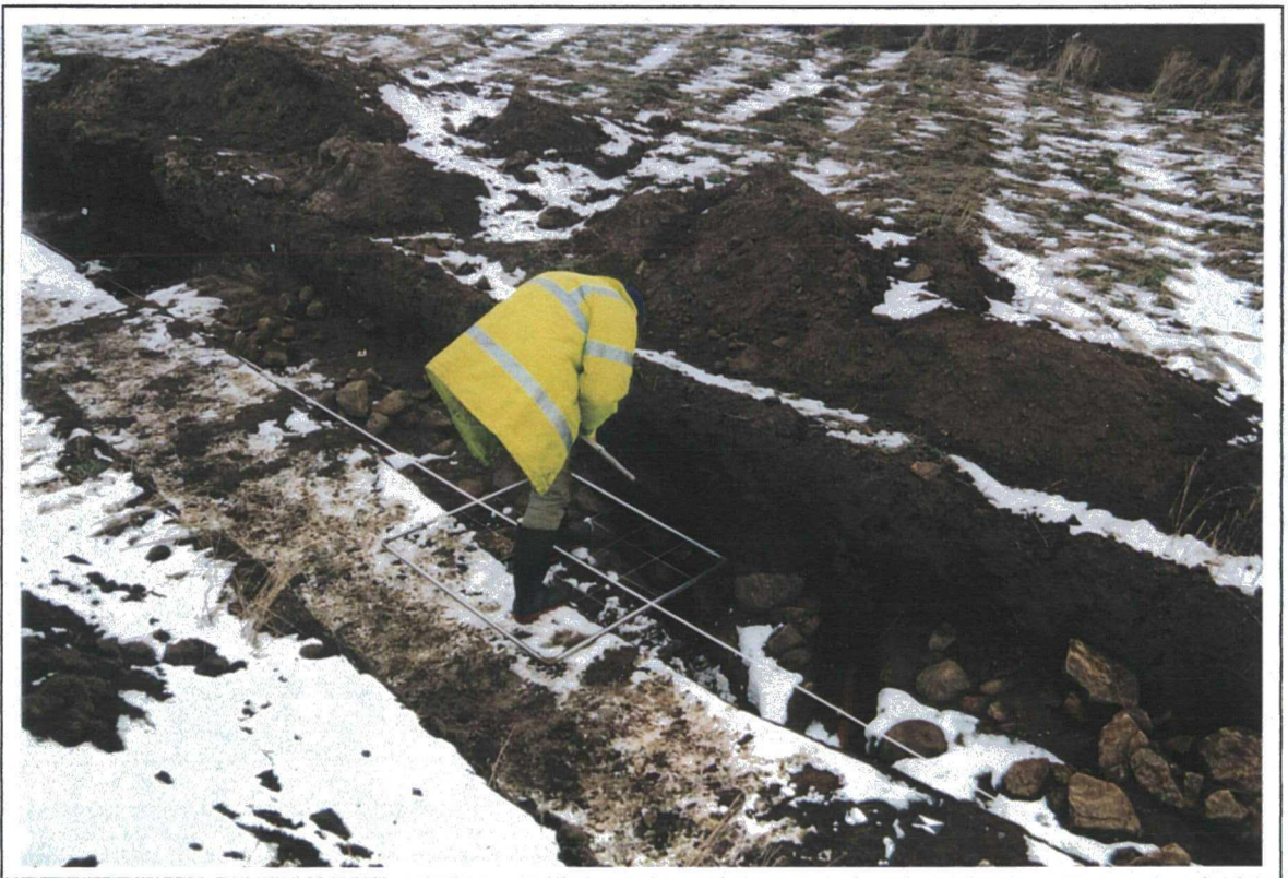
Plate 8. Trench 4. Dave Tyler at work.
