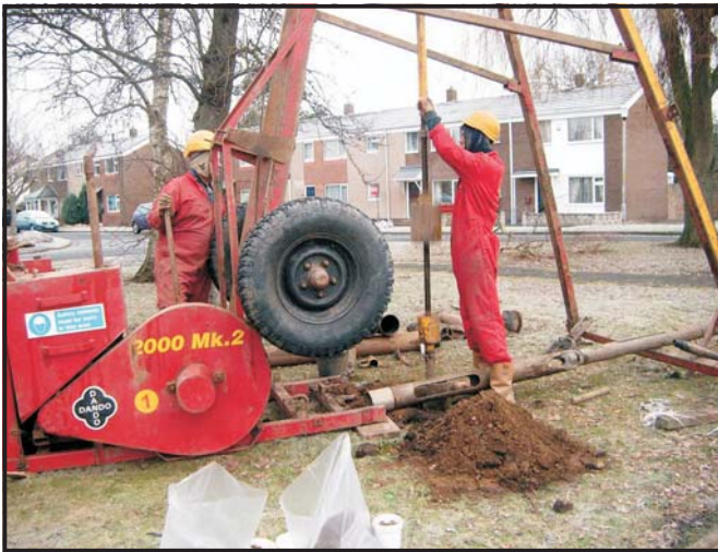
Illus 23: The coring rig in use.
