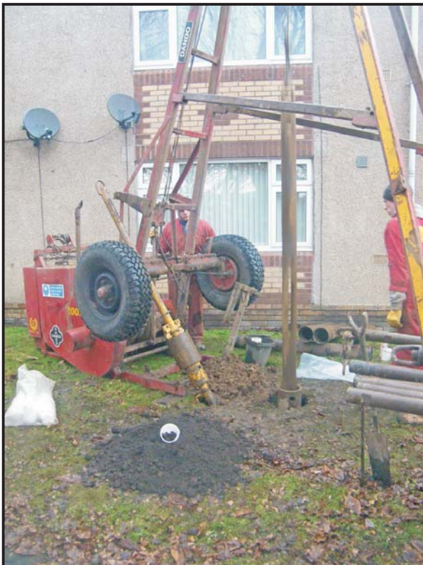
Illus. 28: Borehole 7, during drilling, with spoil from hand-excavated initial pit in foreground.
