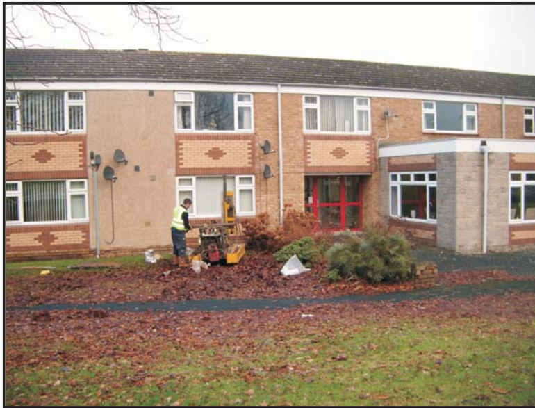
Illus. 13: Borehole 3 viewed from the south.
